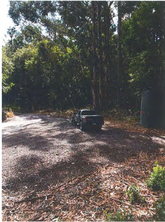
Figure 7: RP 4. Large turnout leading to the Single-Lane Bridge. Vehicle traveling east, photo taken facing east.
