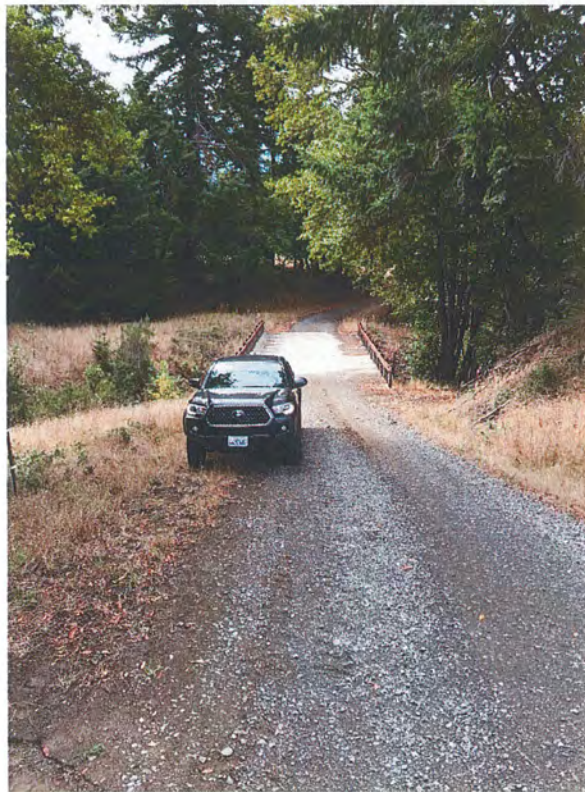
Figure 30: RP 11. Two-Lane Bridge. Vehicle traveling east, photo taken facing west.
