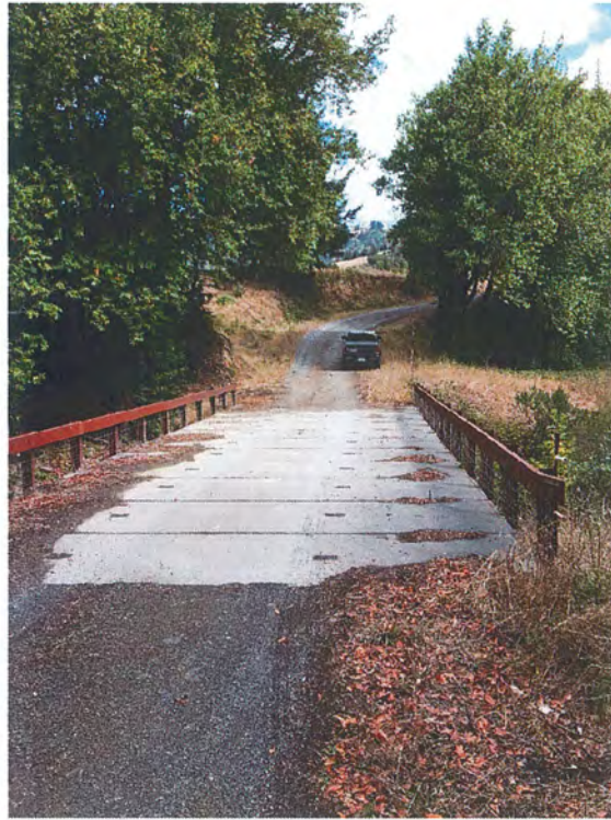
Figure 29: RP 11. Two-Lane Bridge. Vehicle traveling east, photo taken facing east.
