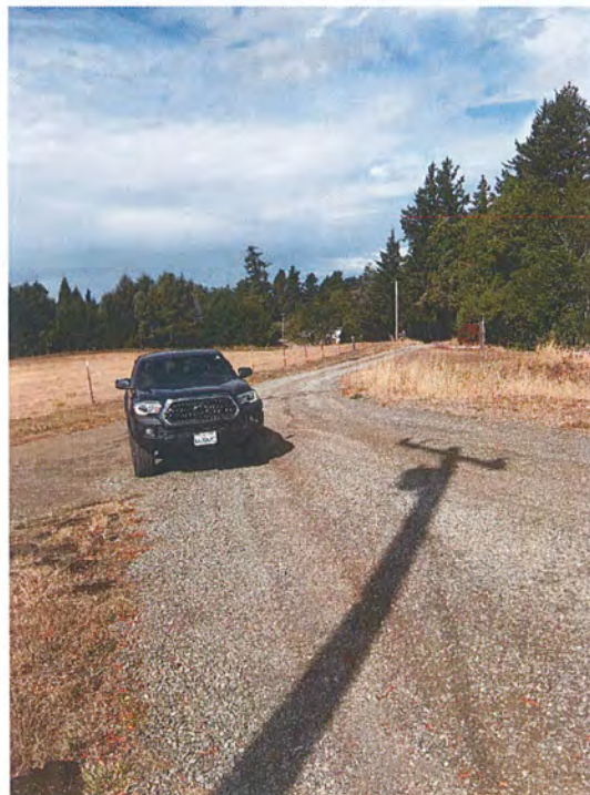
Figure 19: RP 8. Typical section of Chambers Rd (non-County maintained). Large turnout areas adjacent to structures. Vehicle traveling east, phot taken west.
