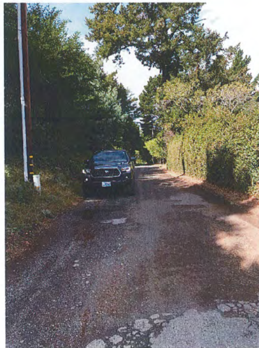
Figure 15: RP 6. Typical section of Chambers Rd (County maintained. State Road No.: 2D020). Vehicle traveling east, photo taken facing east.
