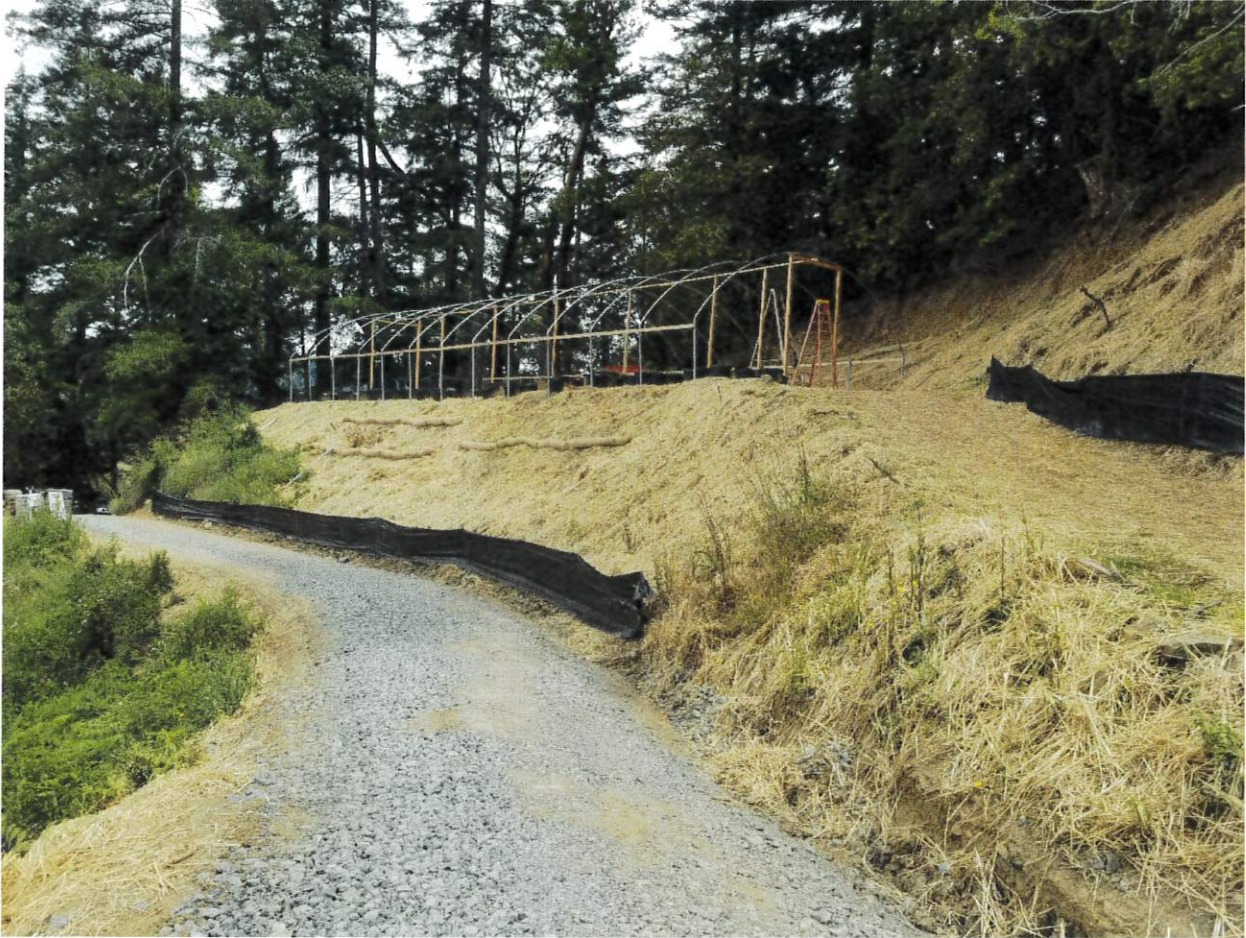
Photo 5: Greenhouse #8. Photo date 6-11-2020
