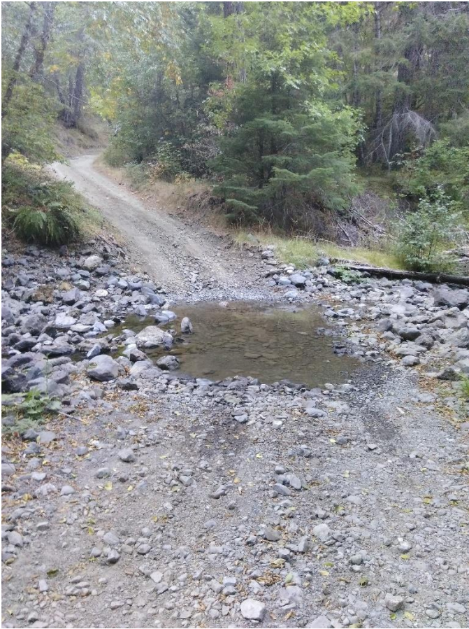
Figure 21. Unimproved stream crossing (Lat/Long 40.6038, -123.7014).
