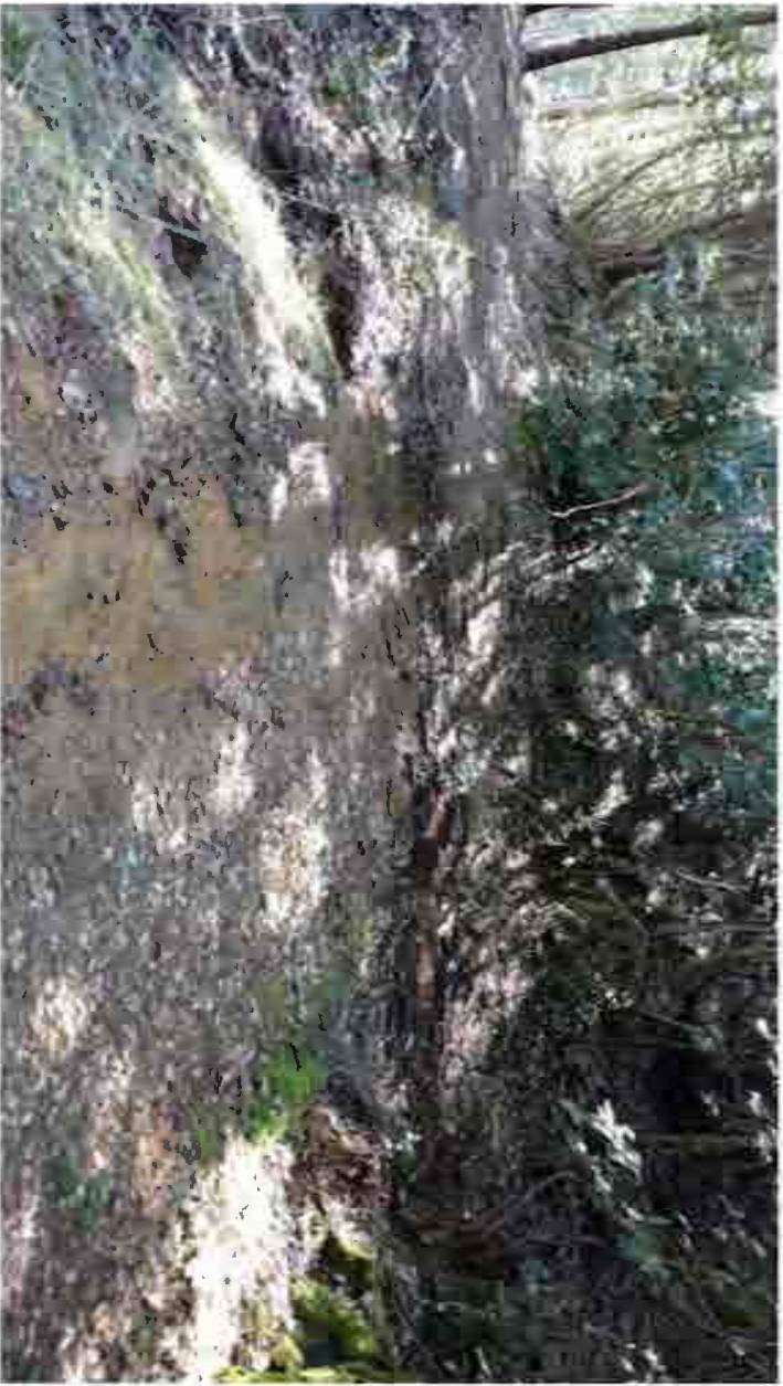
Figure 4. Site number 4, fill crossing on a Class III Watercourse
