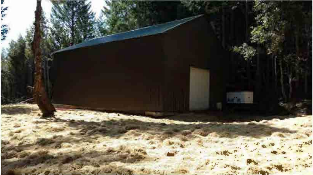
Figure 14. Site number 14, generator without fuel containment in front of storage barn
