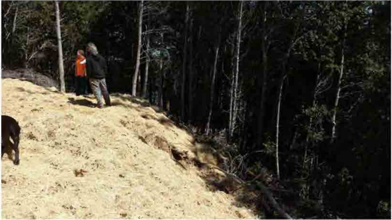
Figure 21. Site number 20, main drainage path of lower graded flat
