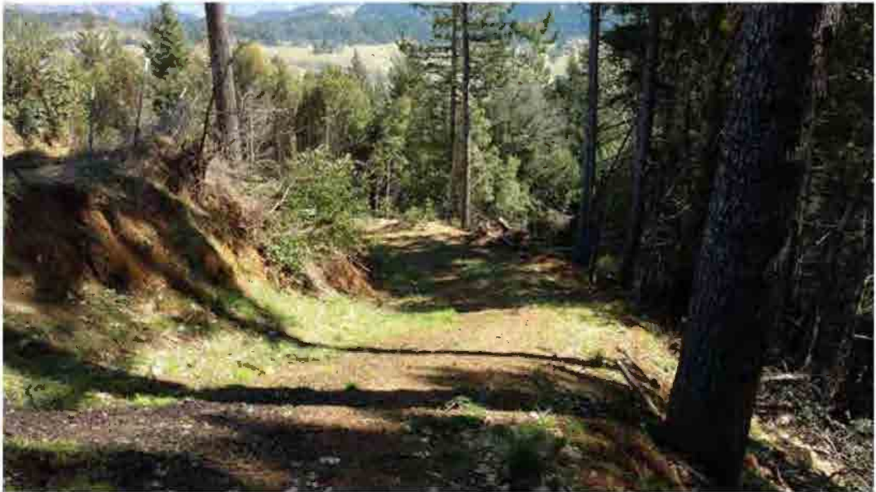
Figure 22. Site number 21, road drainage needed, rolling dip location
