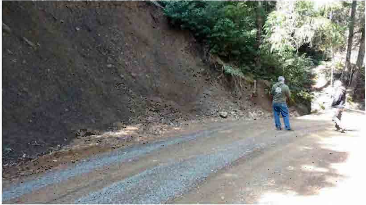
Figure 30. Site number 30, inside dich leading to the culvert inlet at Site 31
