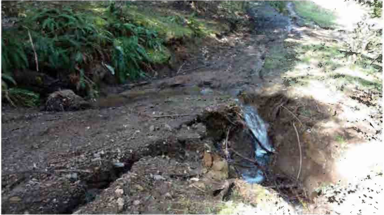
Figure 7. Site number 6, fill crossing on Class II Watercourse
