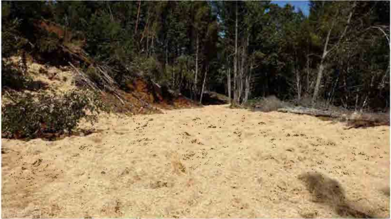
Figure 20. Site number 19, lower graded pad
