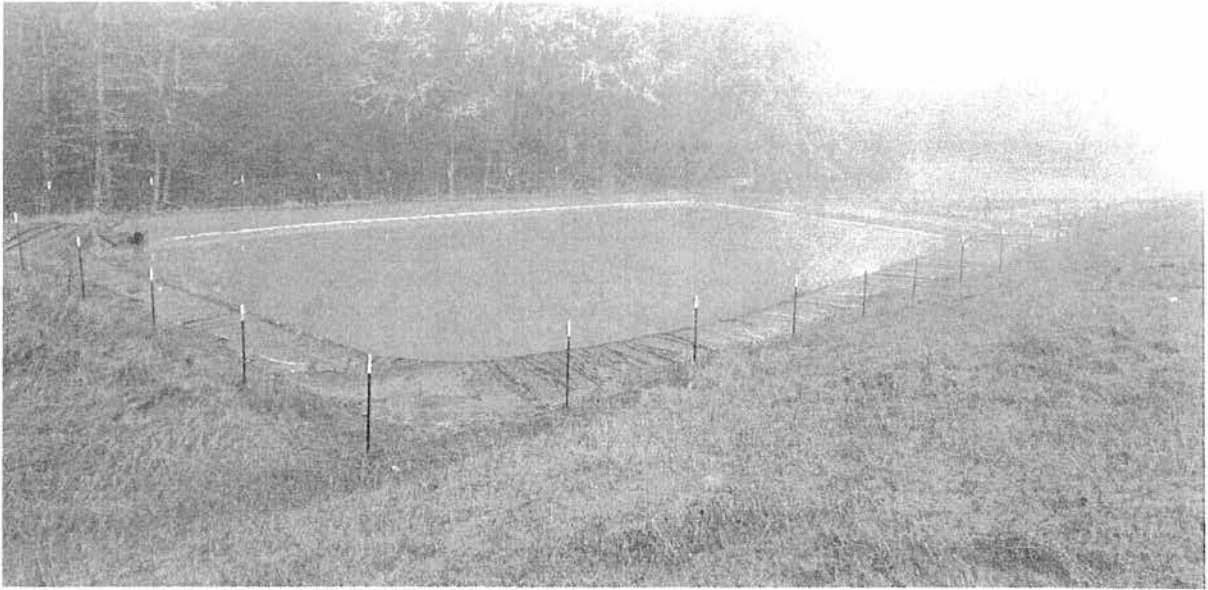
Photo looking southwest at the rain-catchment pond.
