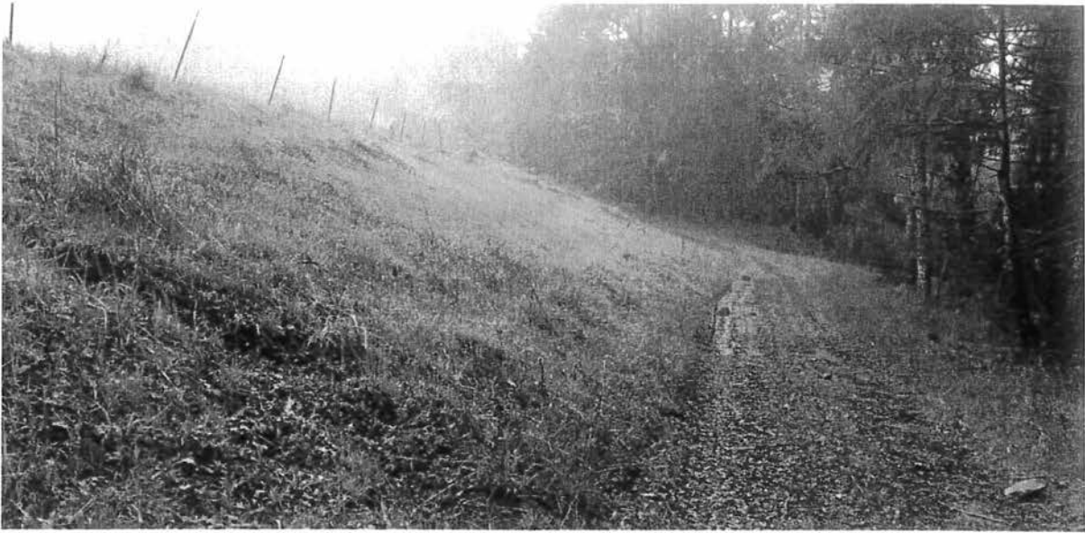
Photo looking southeast the the southern pond embankment.
