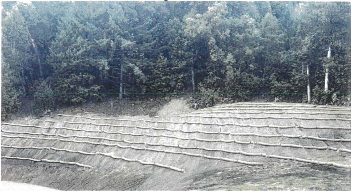
Jute netting & Straw-wattles
