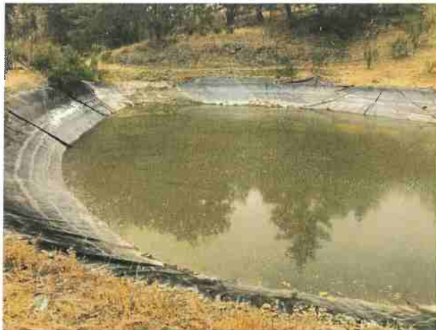
Photo 3. View of lowest side near the outlet pipe.
