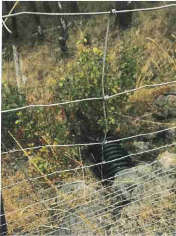
Photo 1. Outlet pipe to adjacent stream.
