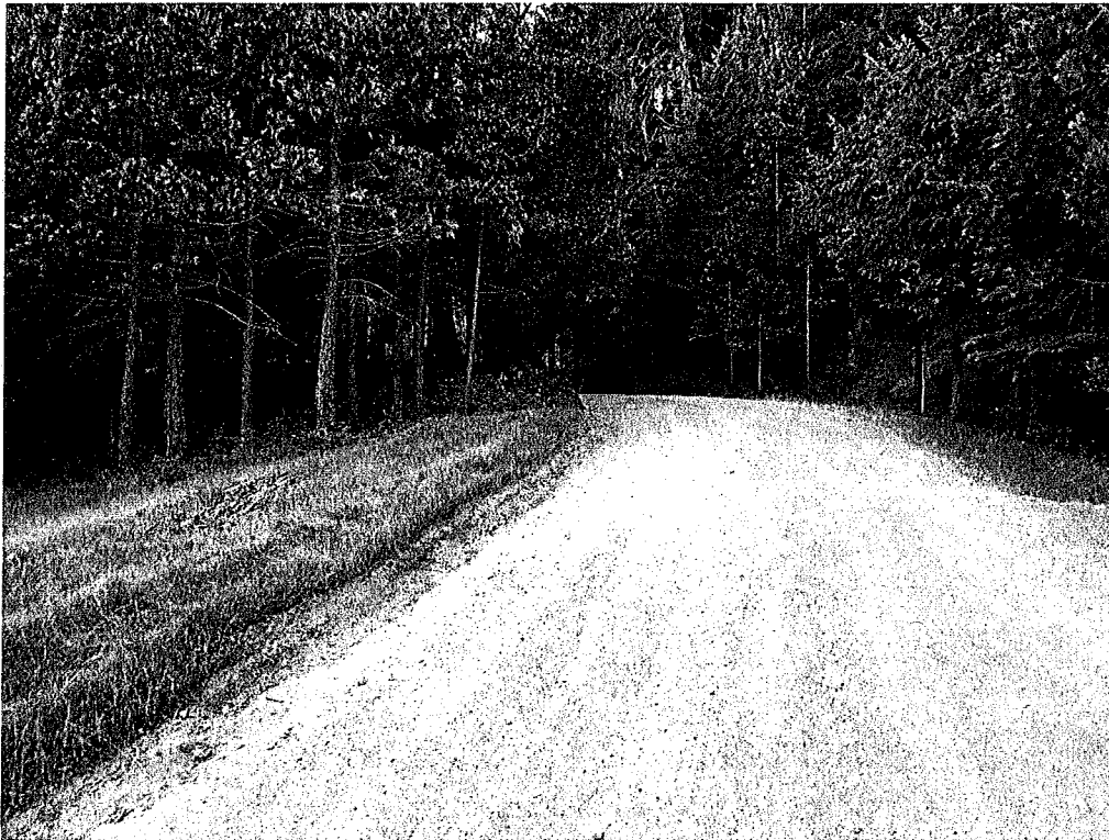
Photo 4. Mile 0.25: 15-ft road width at pinch point with tree.
