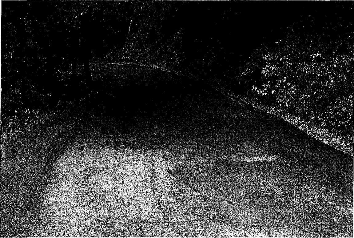
Photo 3. Mile 0.3: 18-ft road width with 1-ft shoulders.
