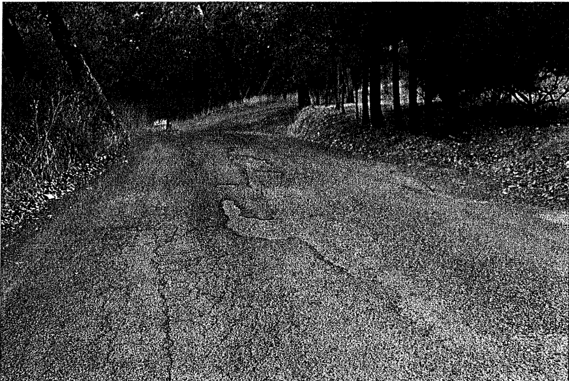
Photo 4. Mile 0.4: 18-ft road width with 1-ft shoulders.
