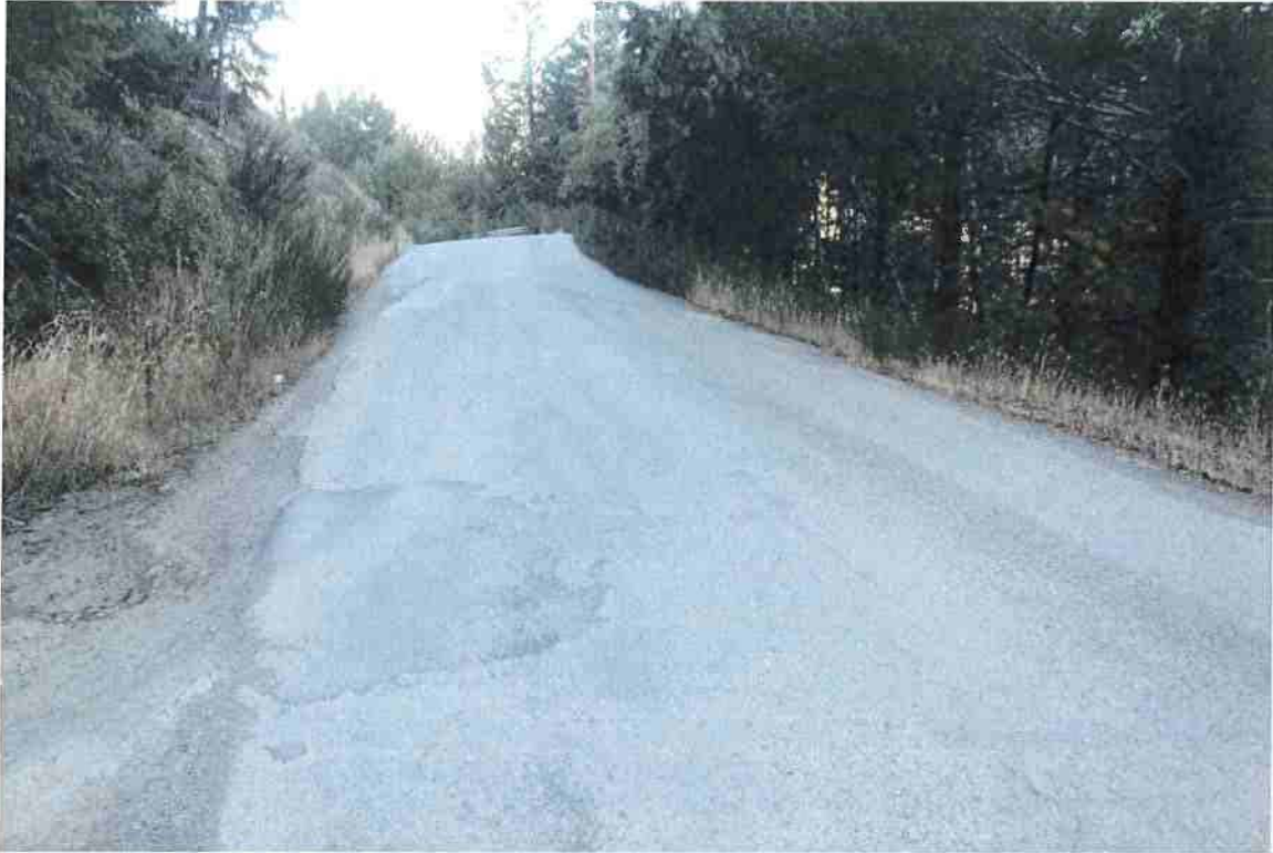
Photo 31. Mile 2.7: 20-ft road width with 2-ft shoulders.
