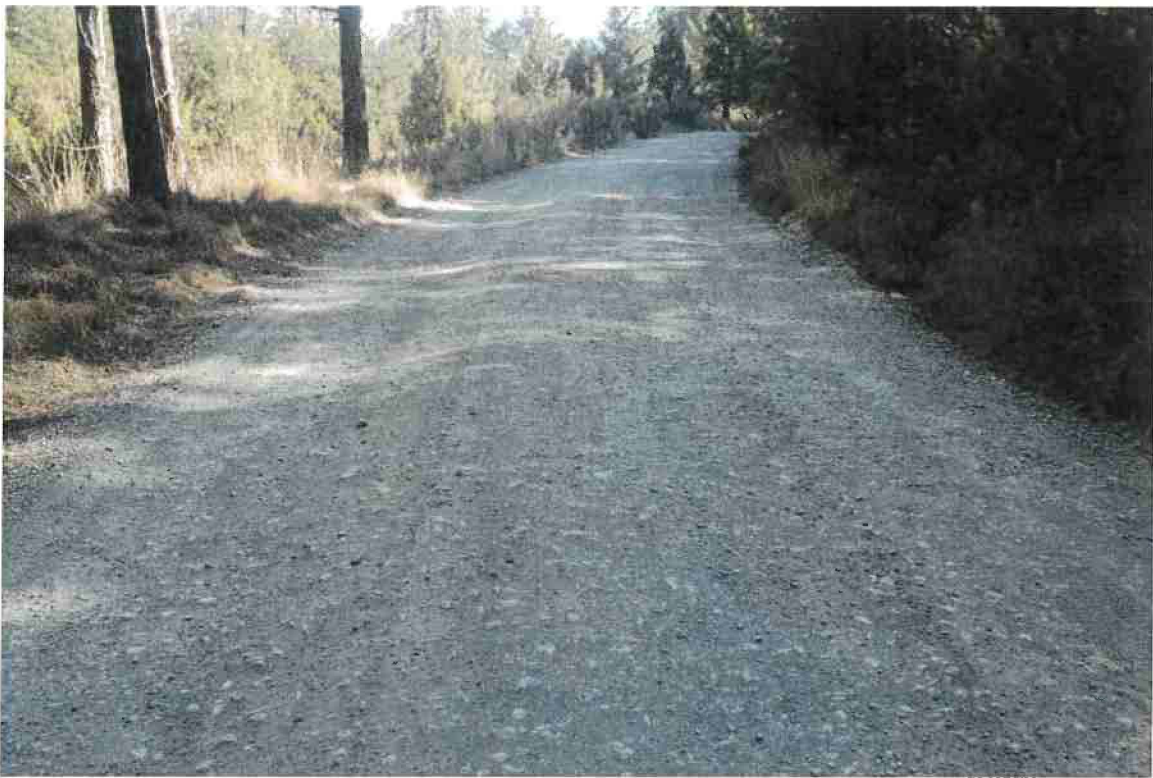
Photo 12. Mile 0.9: 18-ft road width with 1-ft shoulder.
