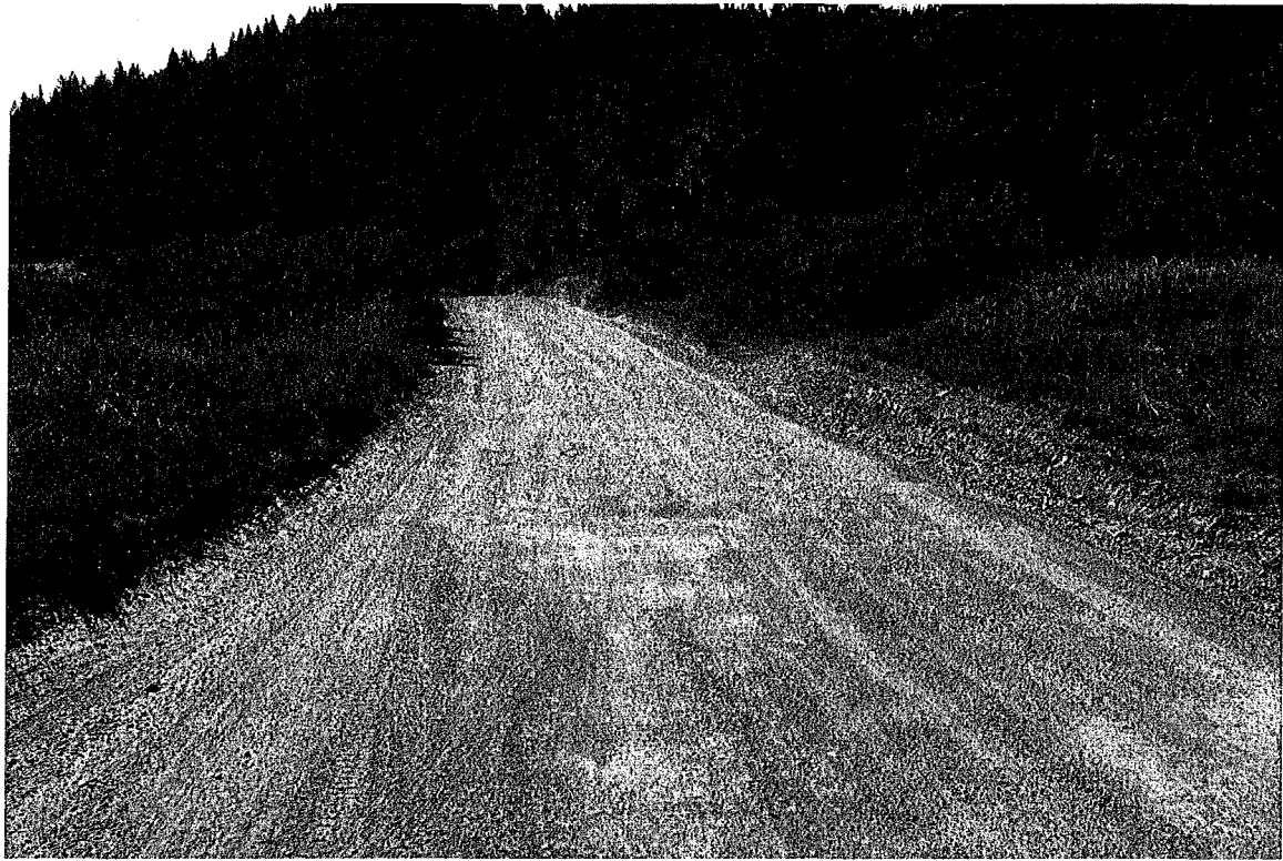
Photo 19. Mile 1.6: 18-ft road width with 1-ft shoulder. End of Segment 3 at Salmon Creek School.
