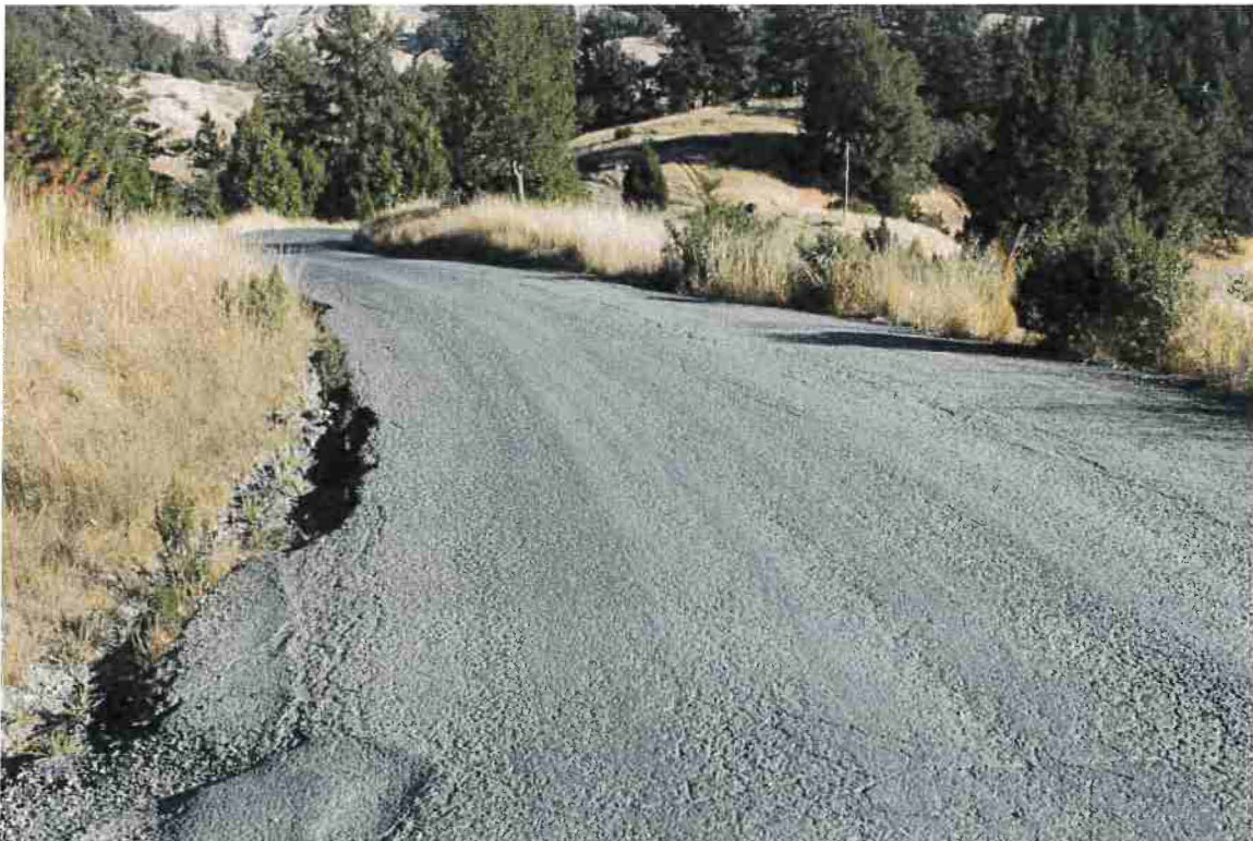
Photo 44. Mile 3.8: 18-ft road width with 1-ft shoulders.
