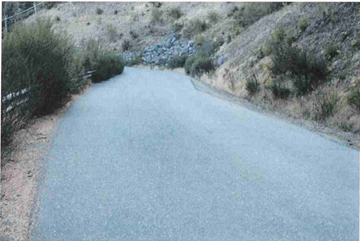
Photo 32. Mile 2.8: 18-ft road width with 1-ft shoulders.
