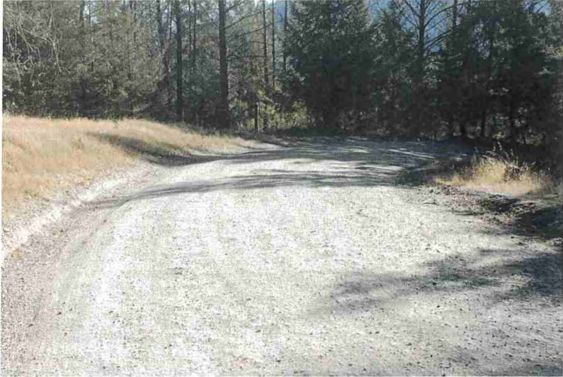
Photo 3. Mile 0.3: 20-ft road width with 2-ft shoulder.
