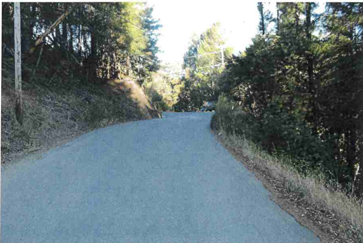
Photo 28. Mile 2.4: 16-ft road width with 1-ft shoulders at blind corner. Potential spot to widen corner on the inside to improve width and visibility.
