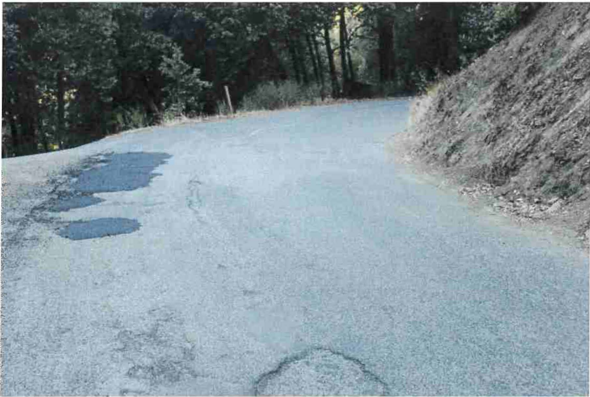
Photo 20. Mile 1.9: 18-ft road width with 2-ft shoulders.
