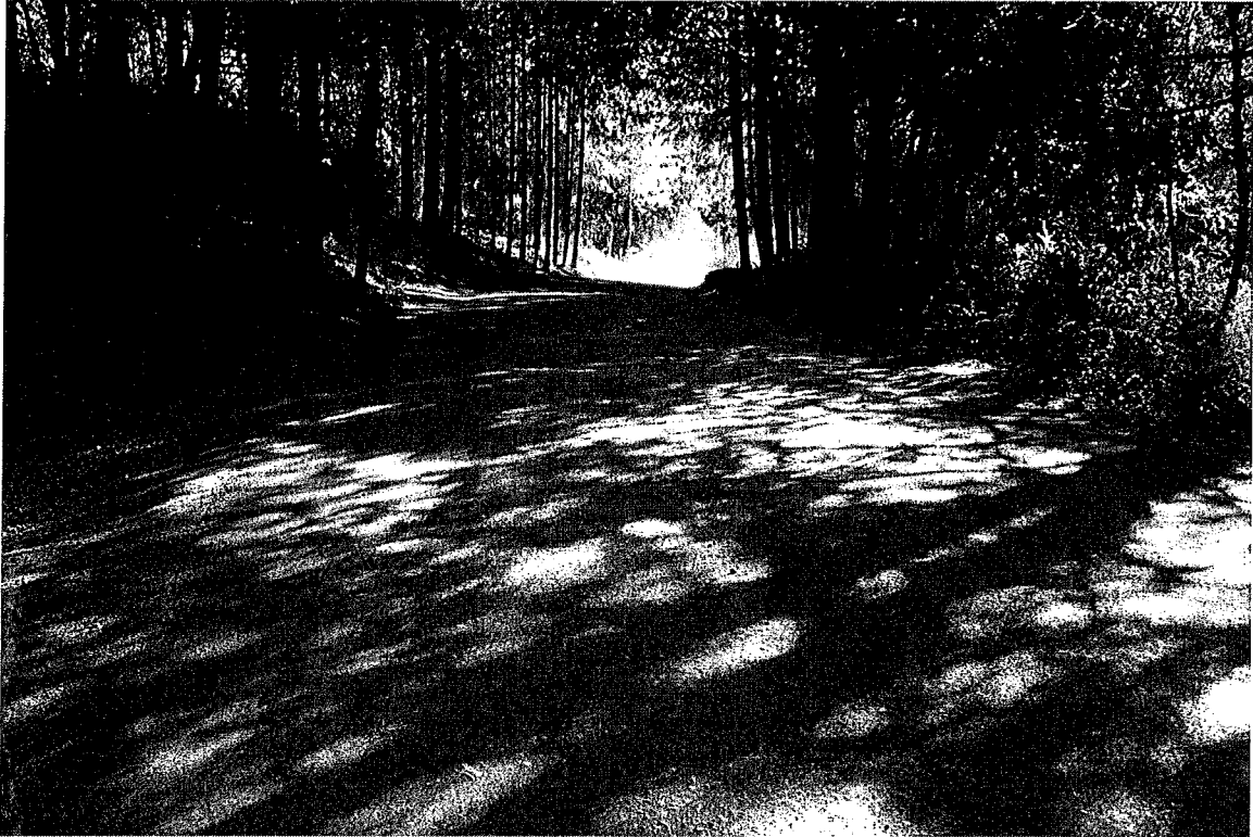
Photo 17. Mile 1.4: 20-ft road width with 2-ft shoulder.
