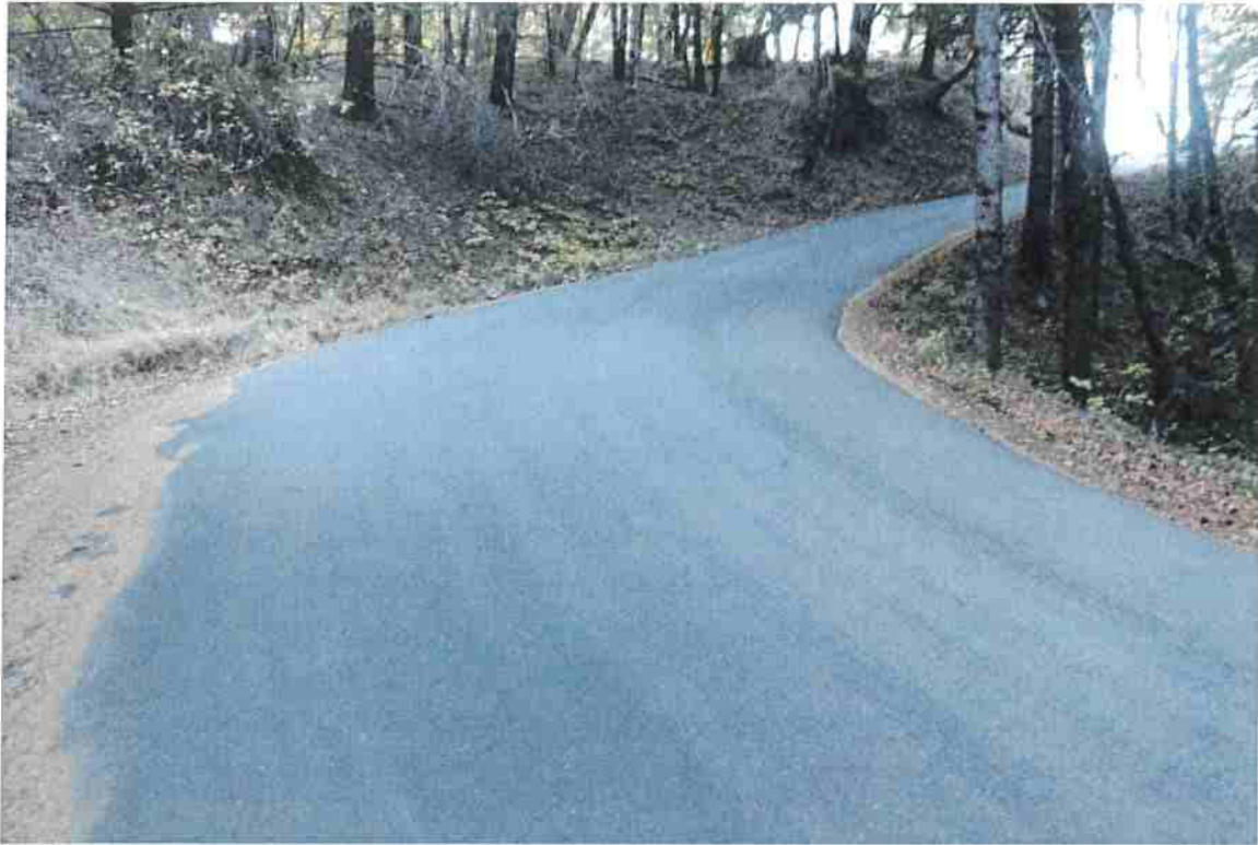
Photo 37. Mile 3.2: 20-ft road width with 2-ft shoulders.
