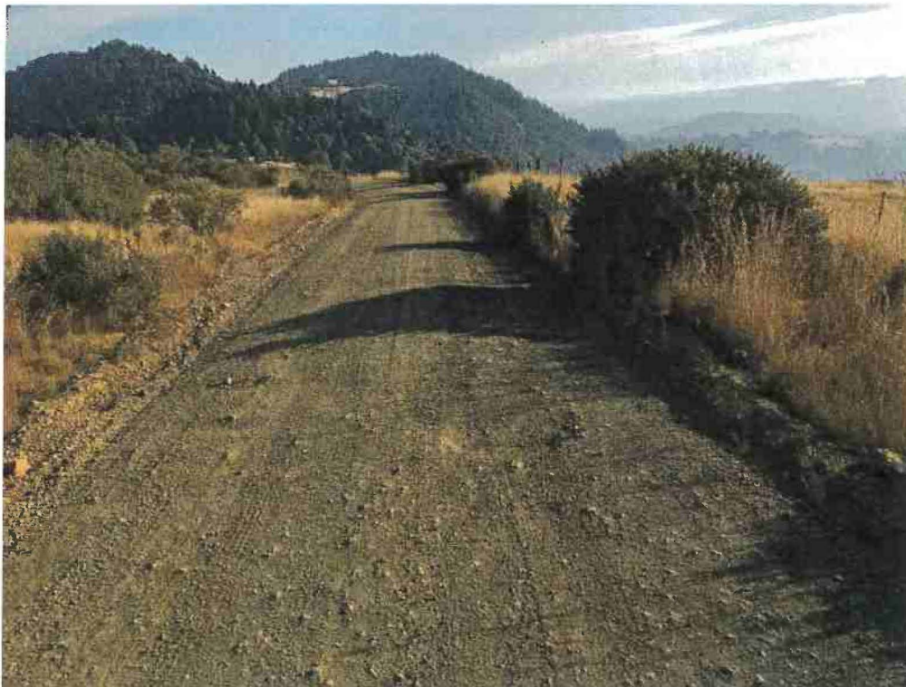
Photo 14. Mile 1.2: 16-ft road width with 2-ft shoulders.
