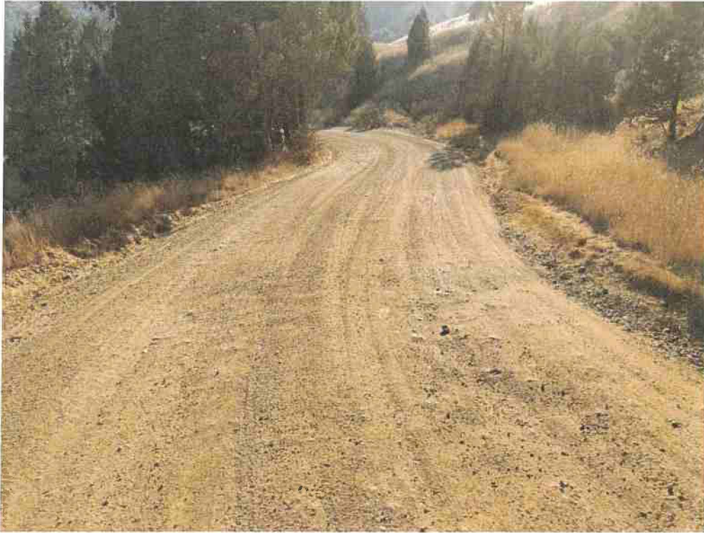
Photo 7. Mile 0.5: 18-ft road width with 2-ft shoulders.
