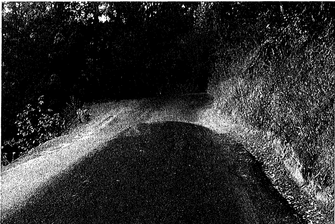
Photo 4. Mile 0.9: relatively narrow section, 15' width, 1' shoulders.
