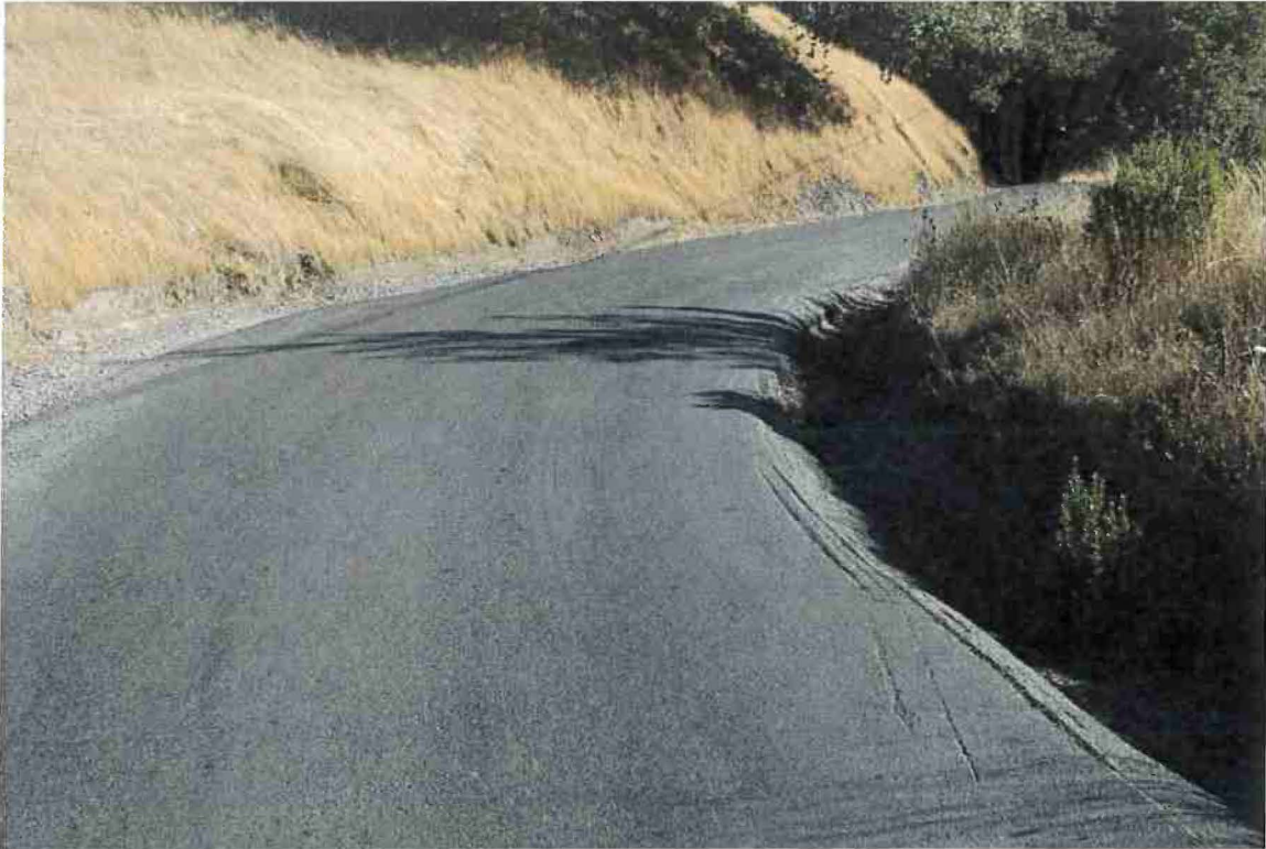
Photo 43. Mile 3.7: 12-ft road width with 1-ft shoulder. Partially blind corner with deep ditch. Potential spot to widen corner on inside to improve width and visibility.
