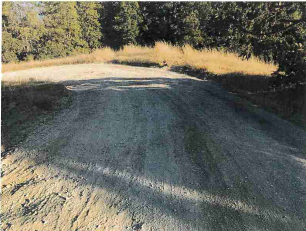
Photo 6. Mile 0.4: 18-ft road width with 1-ft shoulders.
