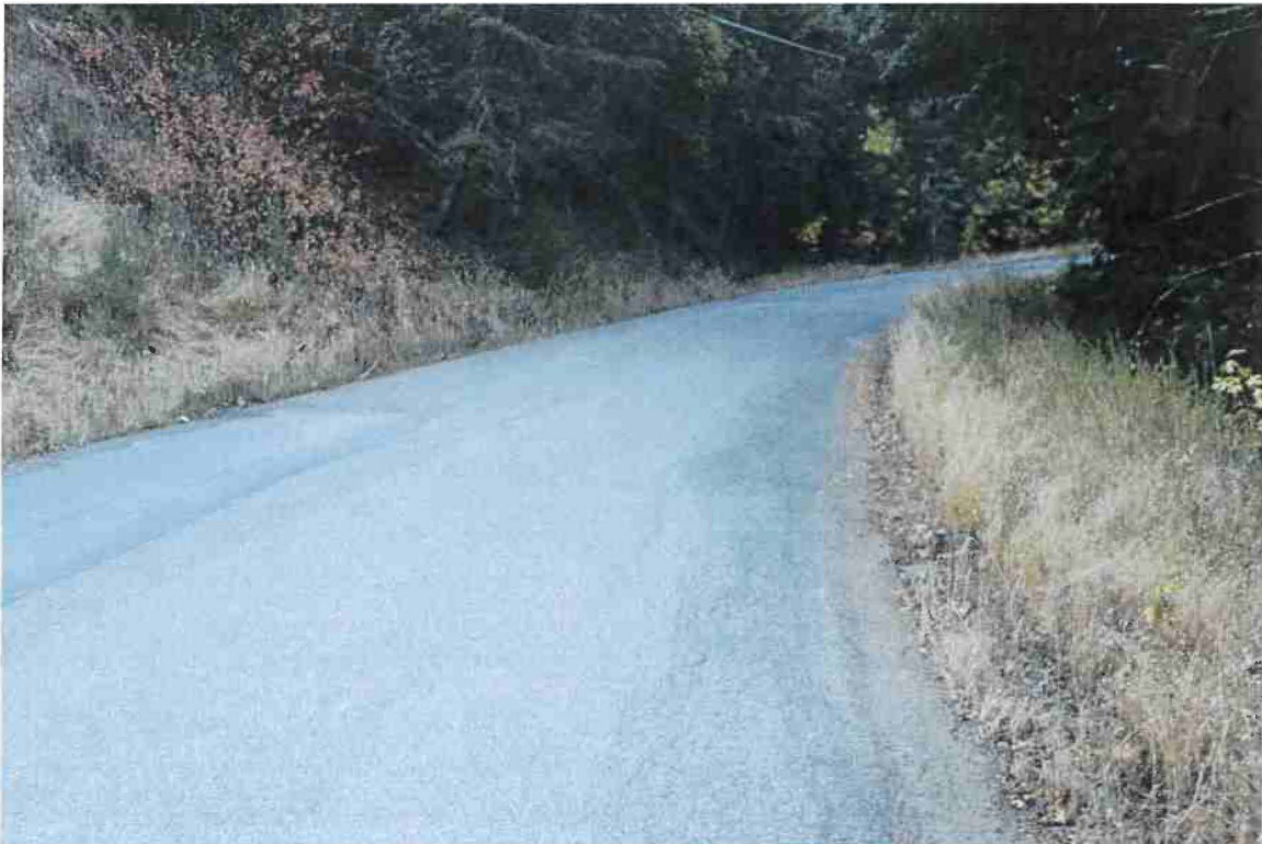
Photo 14. Mile 1.3: 22-ft road width with 2-ft shoulders.
