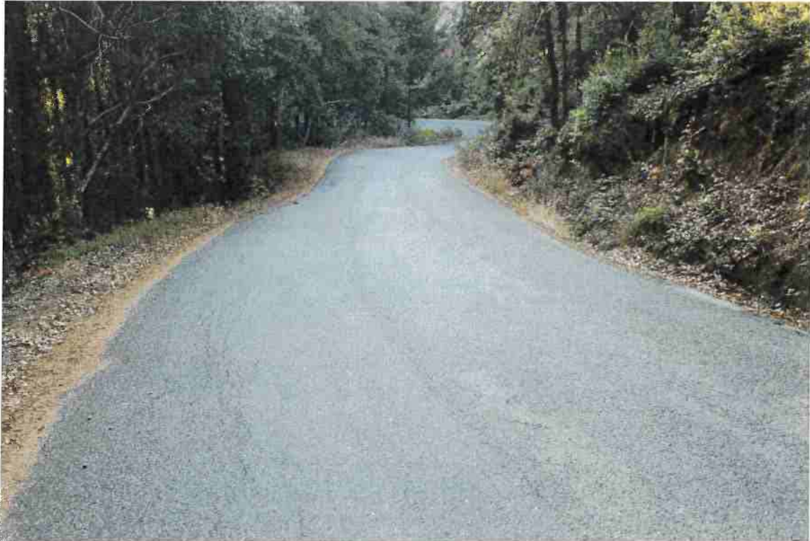
Photo 16. Mile 1.5: 20-ft road width with 1-ft shoulders.
