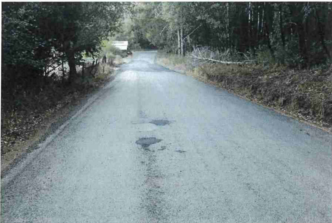
Photo 8. Mile 0.7: 20-ft road width with 2-ft shoulders.
