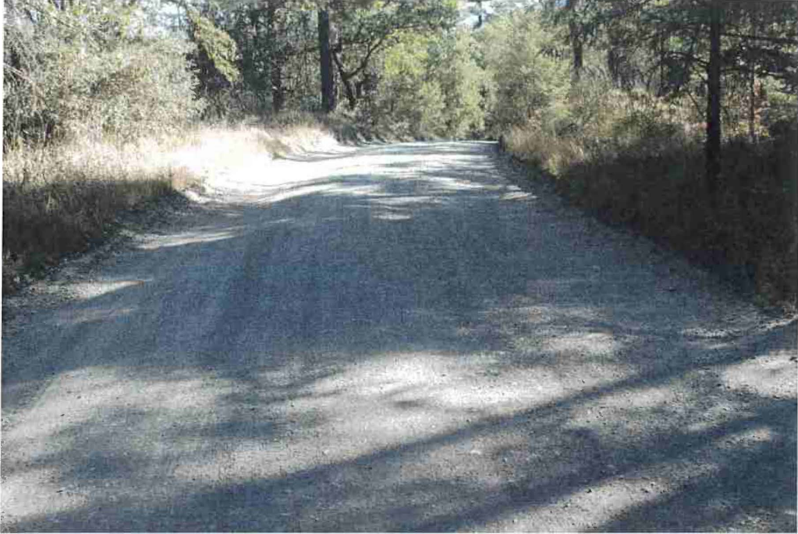
Photo 9. Mile 0.6: 18-ft road width with 1-ft shoulder.
