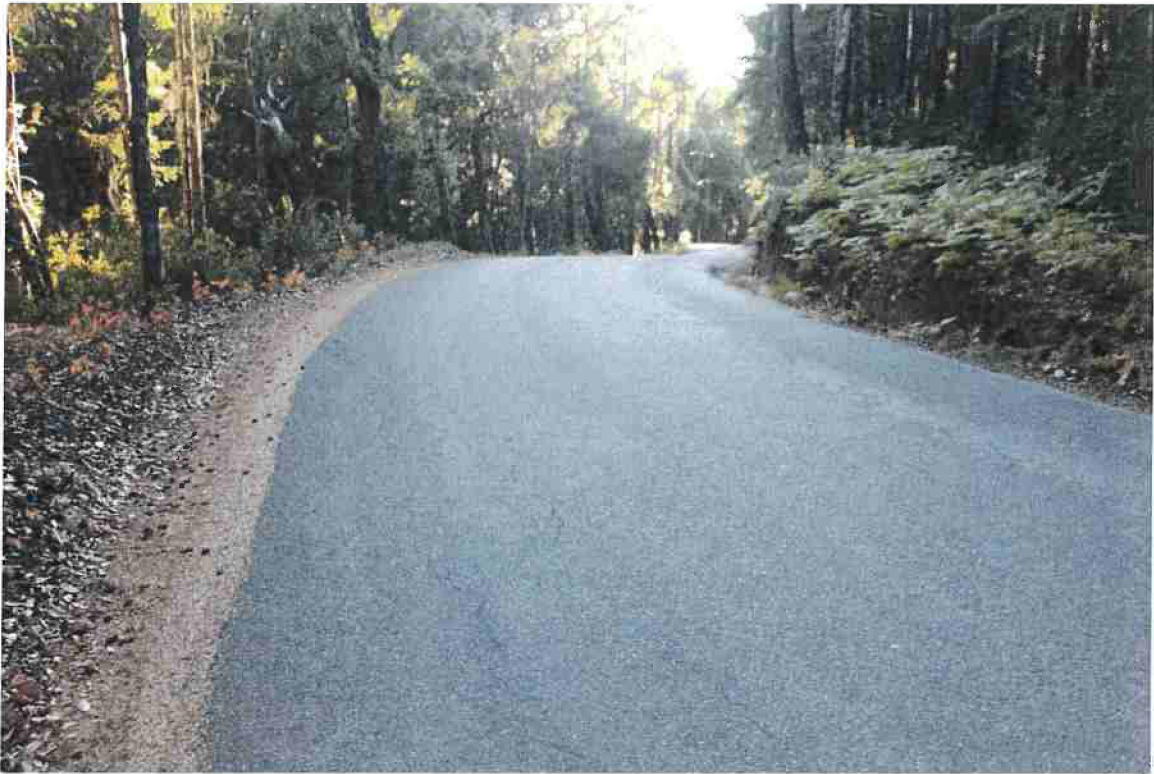
Photo 17. Mile 1.6: 20-ft road width with 2-ft shoulders.
