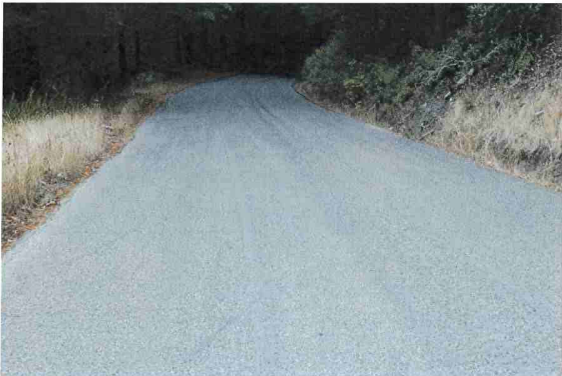
Photo 2. Mile 0.2: 18-ft road width with 1-ft shoulders.
