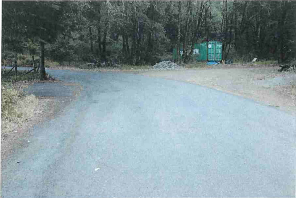
Photo 7. Mile 0.6: 24-ft road width with 2-ft shoulders.
