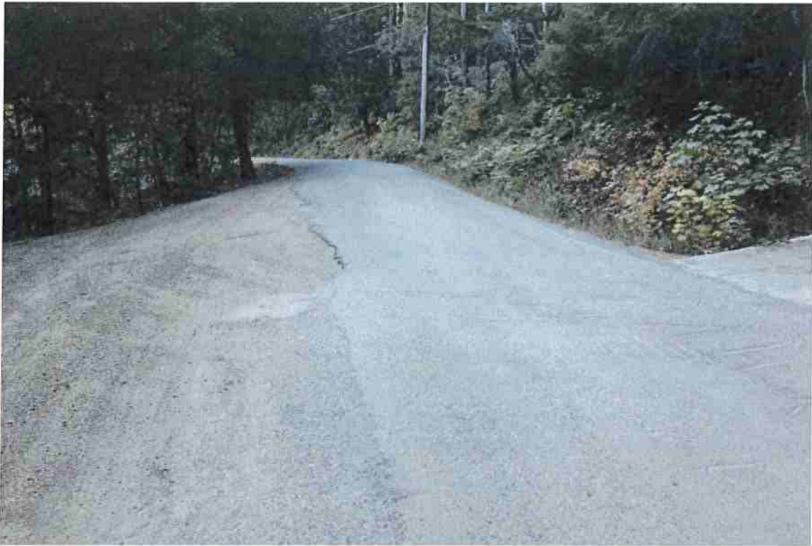
Photo 25. Mile 2.3: 20-ft road width with 2-ft shoulders.
