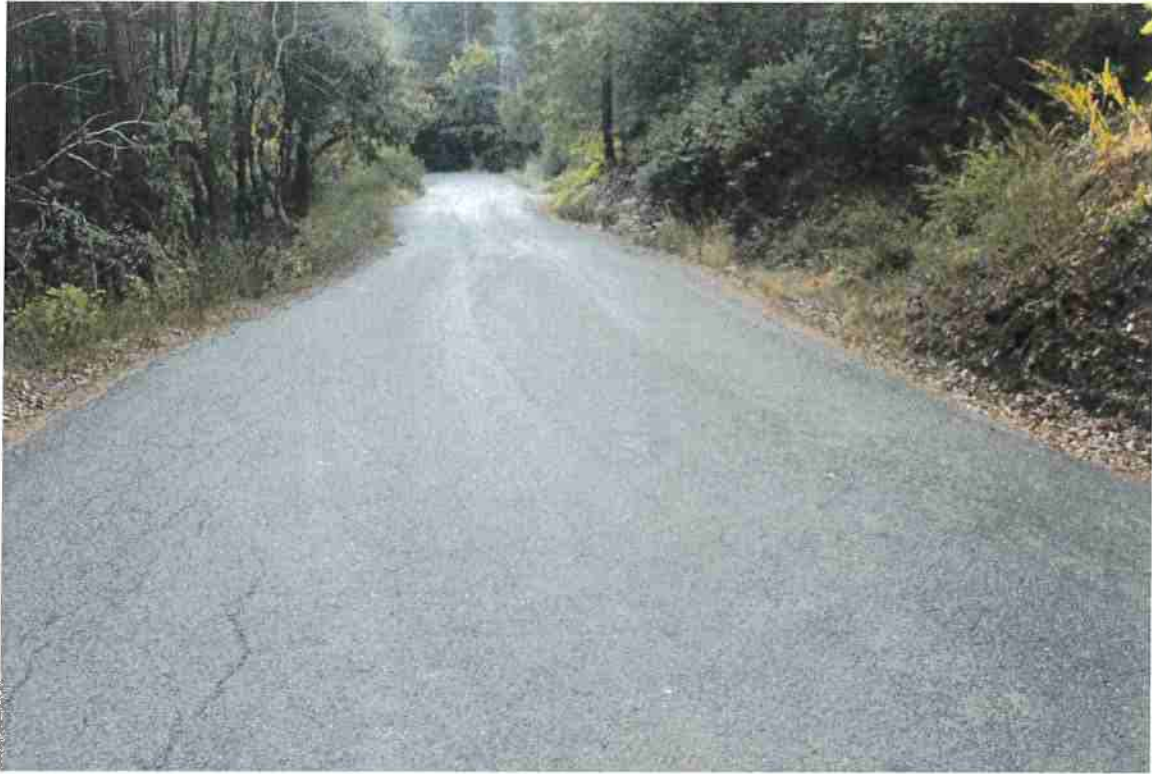
Photo 15. Mile 1.4: 22-ft road width with 1-ft shoulders.
