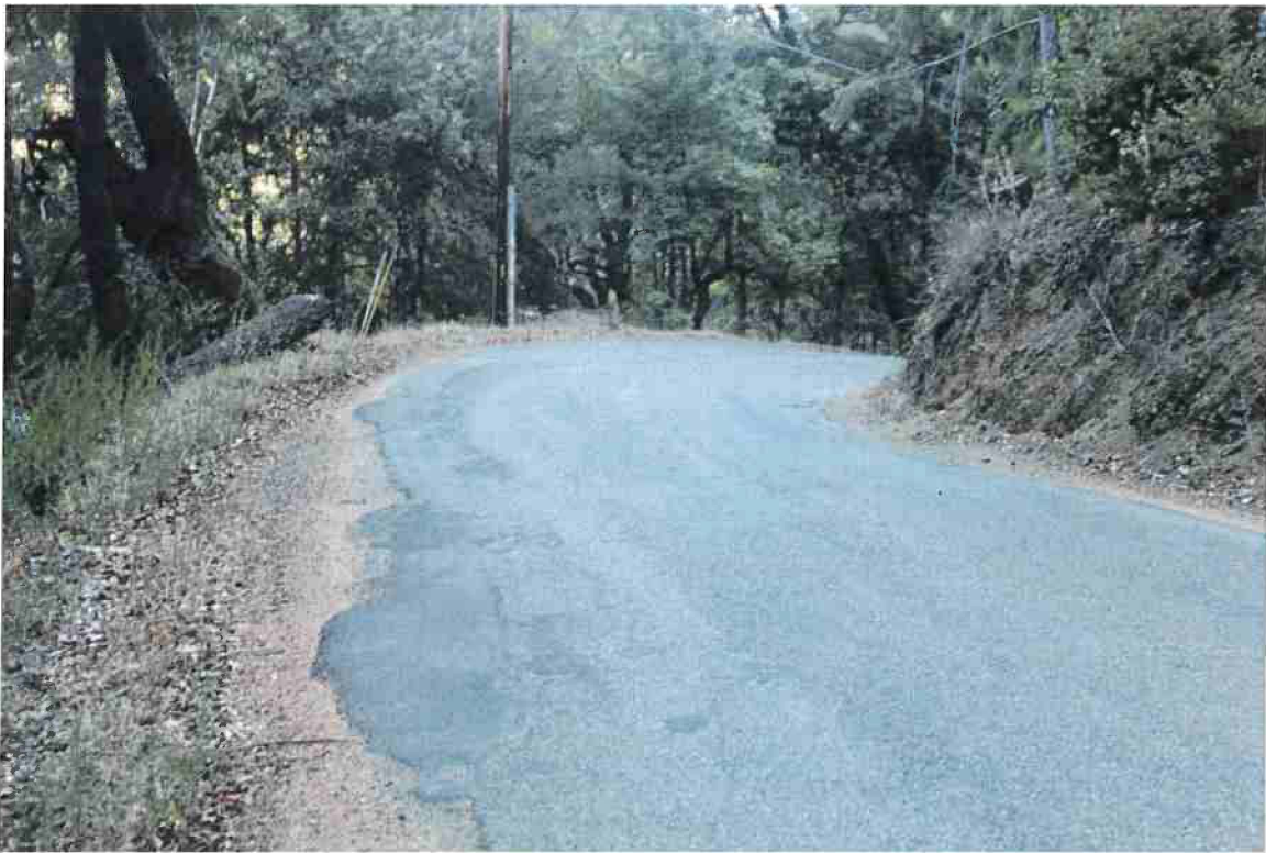
Photo 24. Mile 2.2: 20-ft road width with 1-ft shoulders.
