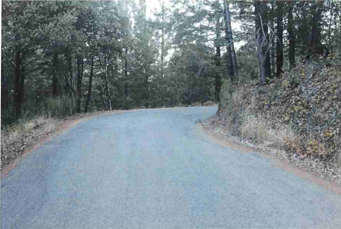
Photo 13. Mile 1.2: 20-ft road width with 1-ft shoulders.
