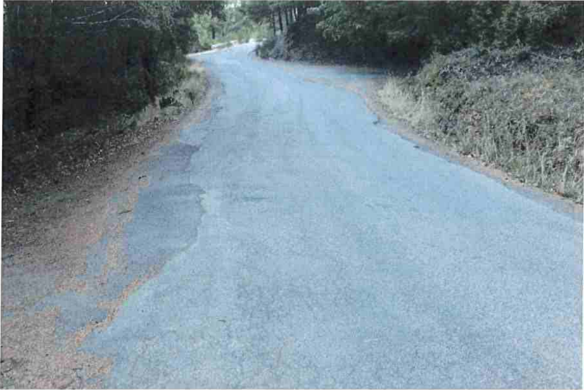
Photo 33. Mile 2.9: 18-ft road width with 1-ft shoulders.
