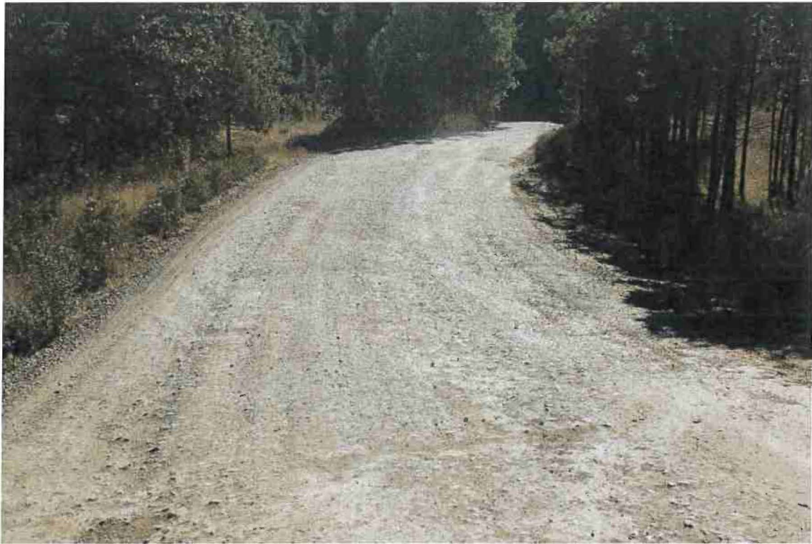
Photo 7. Mile 0.5: 18-ft road width with 1-ft shoulder.
