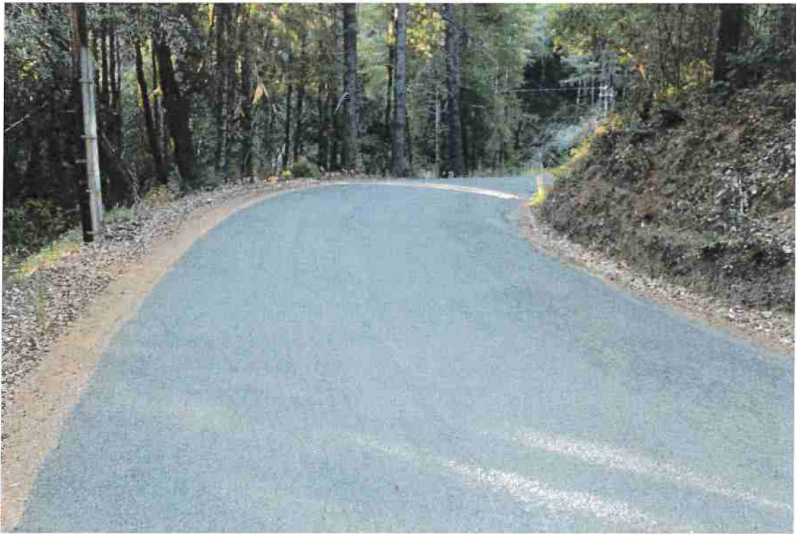
Photo 18. Mile 1.7: 20-ft road width with 1-ft shoulders.
