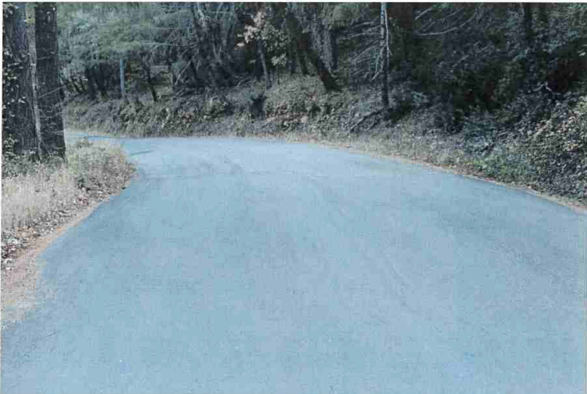
Photo 12. Mile 1.1: 20-ft road width with 2-ft shoulders.
