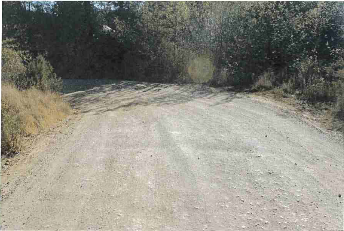
Photo 11. Mile 0.8: 22-ft road width with 1-ft shoulder.
