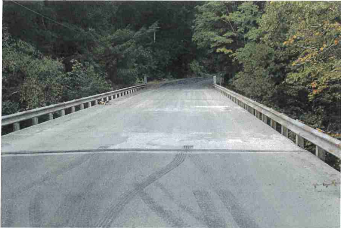
Photo 11. Mile 1.45: 28' width bridge, no shoulders.
