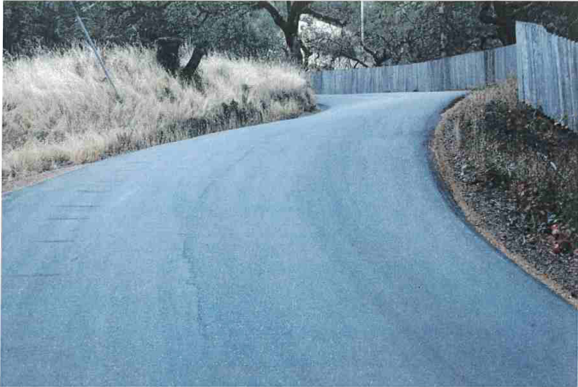
Photo 35. Mile 3.1: 20-ft road width with 1-ft shoulders.
