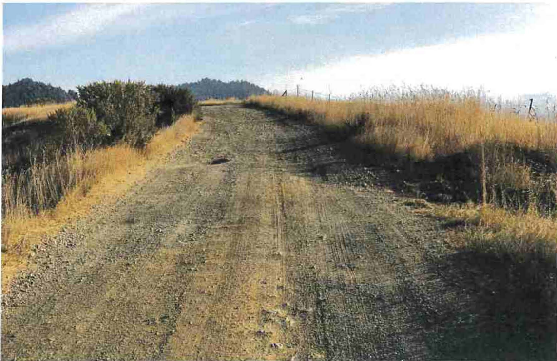
Photo 16. Mile 1.4: 15-ft road width with 2-ft shoulders.
