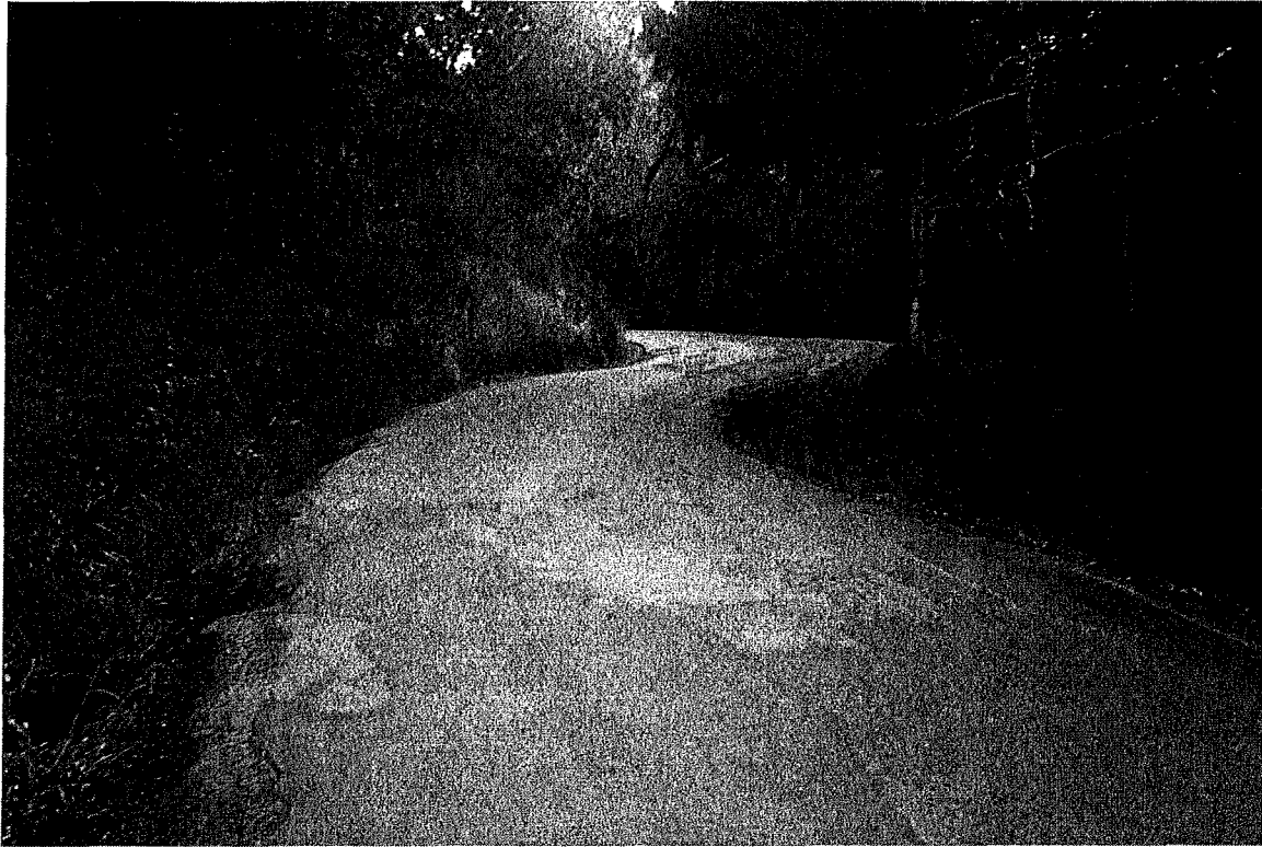
Photo 3. Mile 0.8: relatively narrow section, 16' width, no shoulder, deep ditch.
