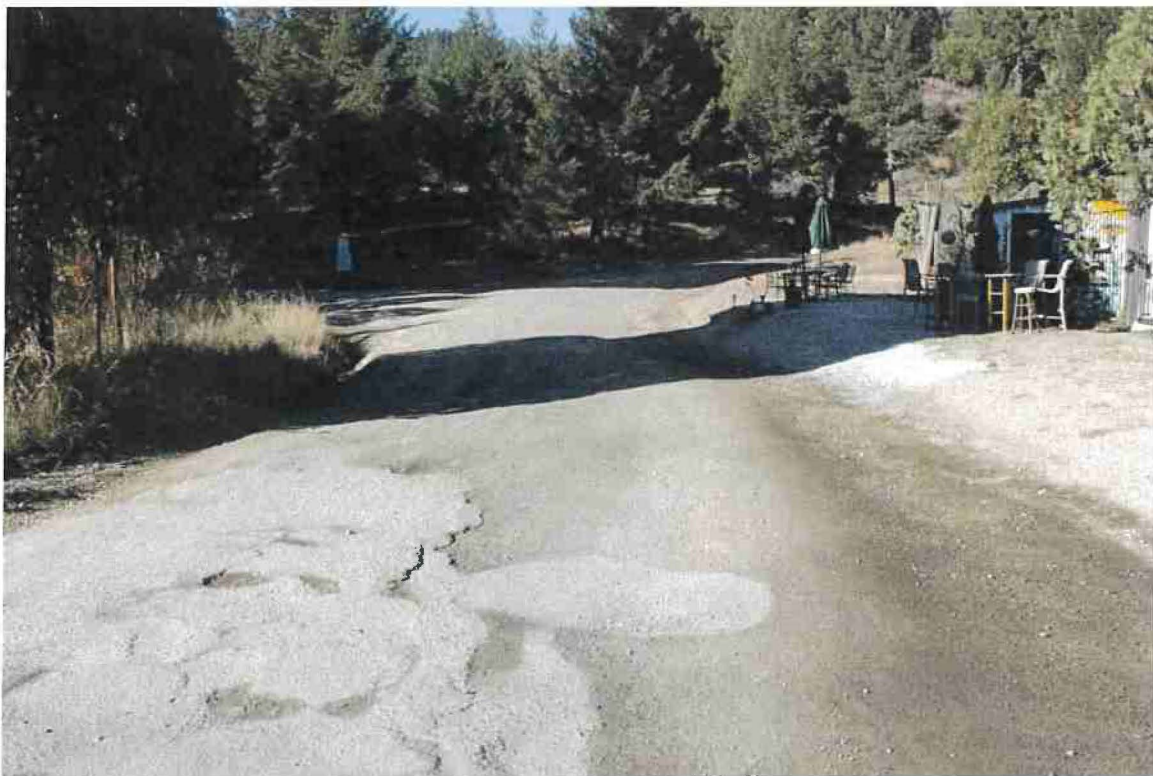
Photo 48. Mile 4.1: 20-ft road width with 2-ft shoulders. Intersection with Upper Thomas Road and end of County-maintained road. End of Segment 2.
