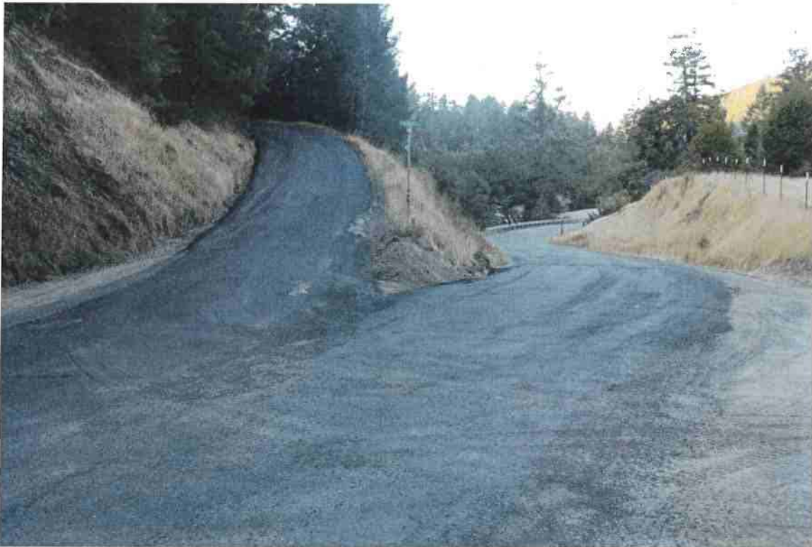
Photo 14. Mile 1.7: Thomas/ Salmon Creek Road split, 32' width, 2' shoulders (end of Segment 1).
