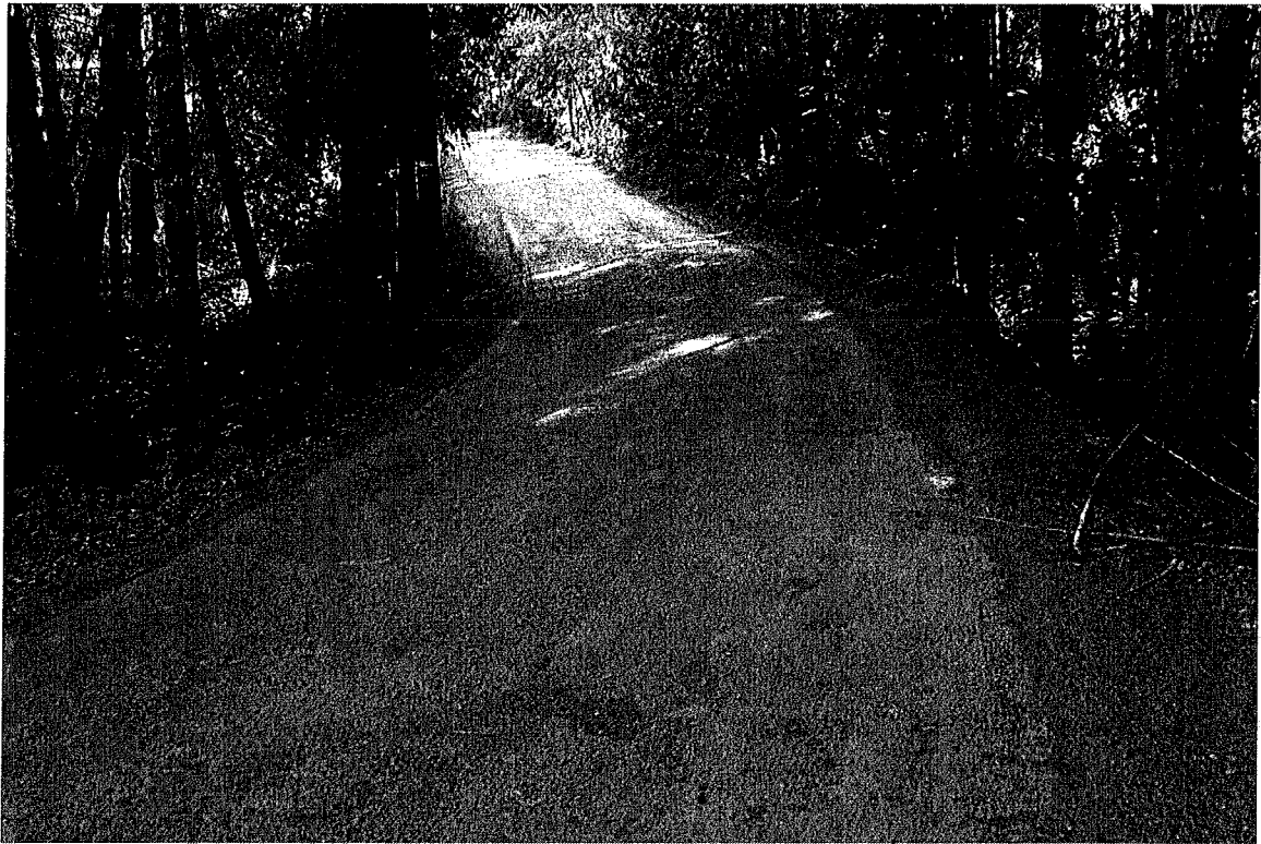
Photo 15. Mile 1.2: 18-ft road width with no shoulder at culvert crossing with decent visibility.
