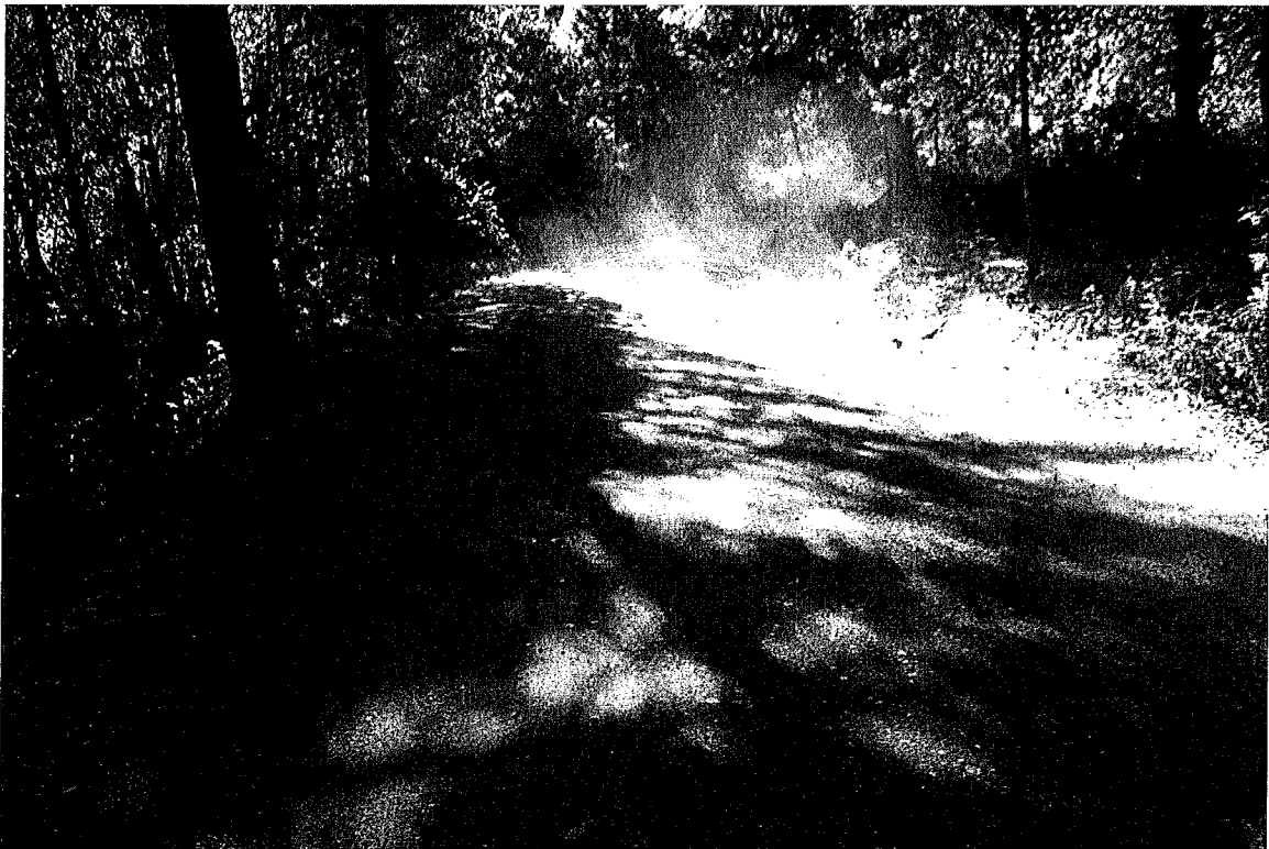
Photo 16. Mile 1.3: 18-ft road width with 2-ft shoulders.
