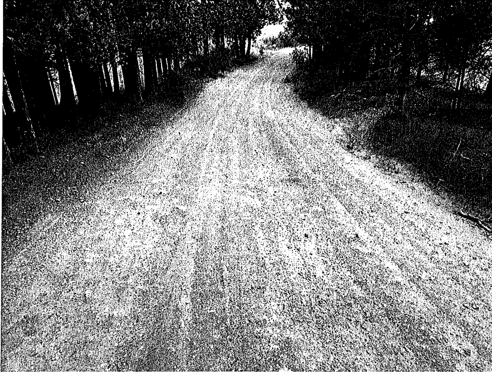
Photo 3. Mile 0.2: 18-ft road width with 1-ft shoulders.
