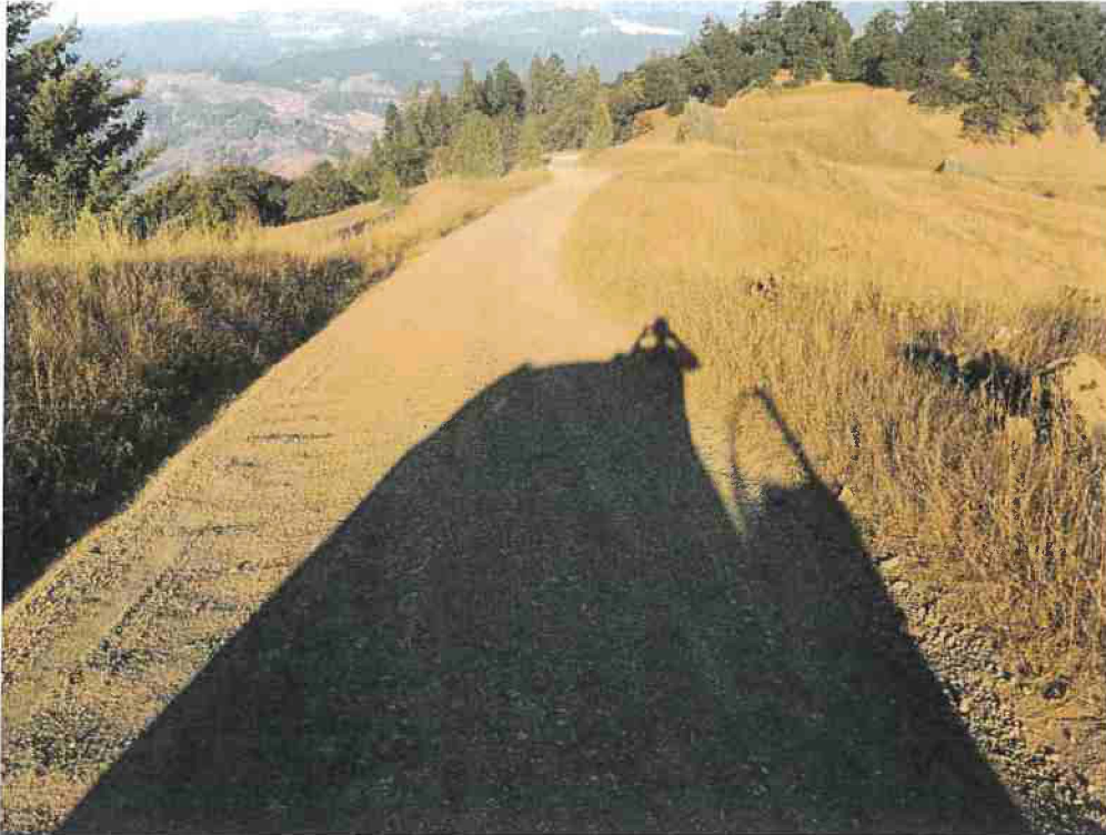
Photo 11. Mile 0.9: 16-ft road width with 2-ft shoulders.
