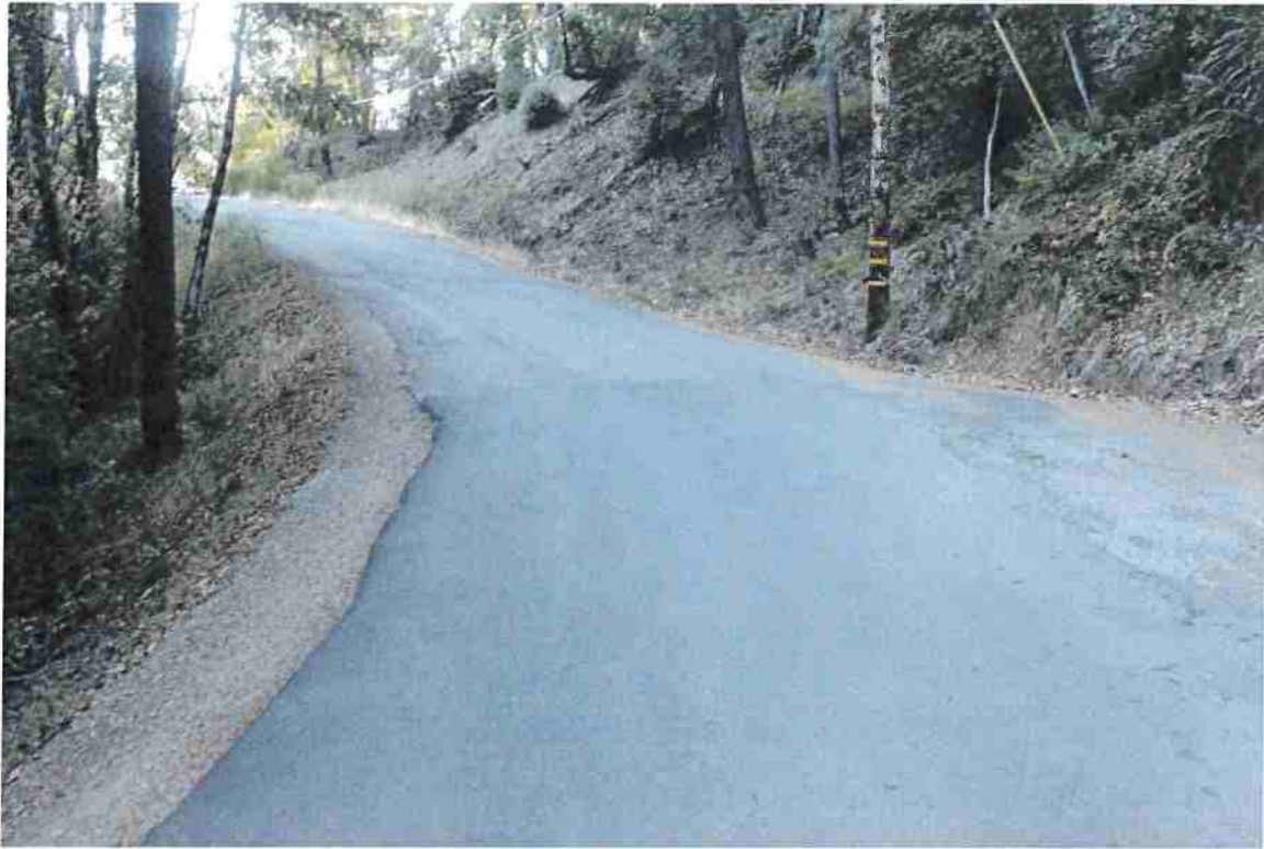
Photo 29. Mile 2.5: 18-ft road width with 2-ft shoulders.
