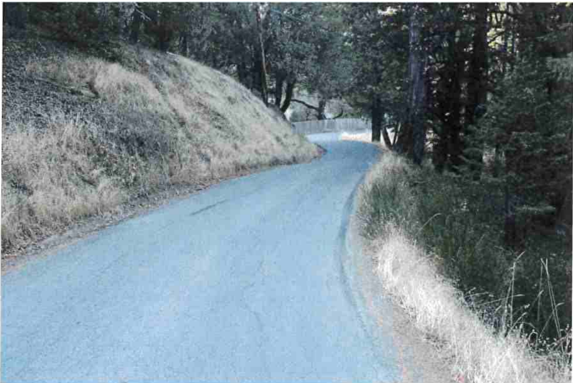
Photo 34. Mile 3.0: 15-ft road width with 1-ft shoulders.
