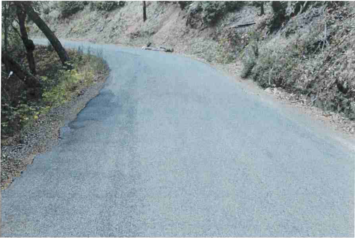
Photo 21. Mile 2.0: 15-ft road width with 1-ft shoulders.
