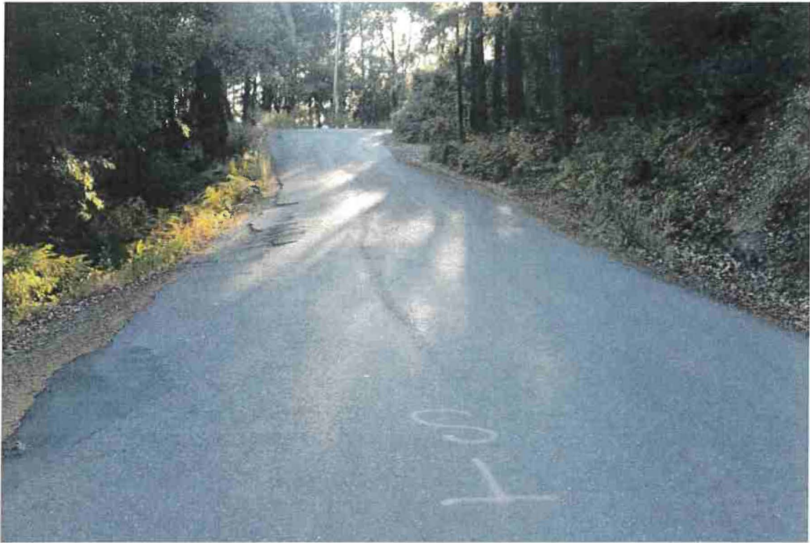
Photo 19. Mile 1.8: 20-ft road width with 2-ft shoulders.
