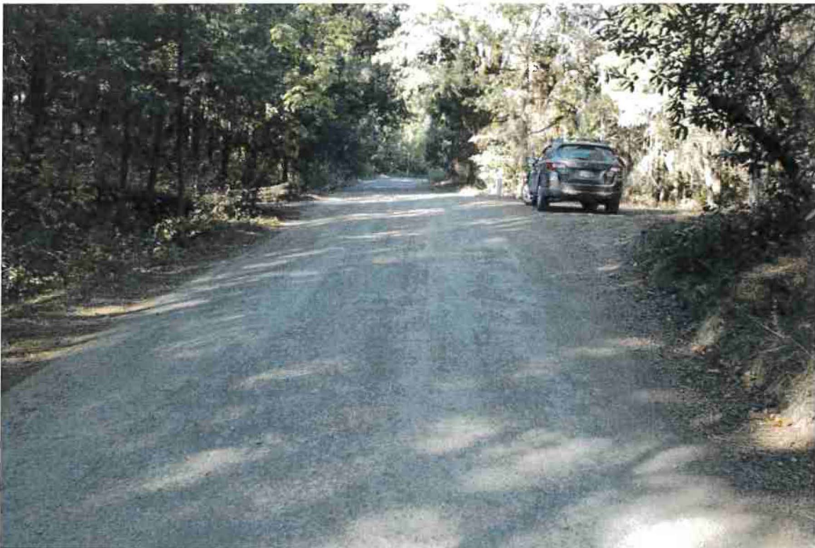
Photo 6. Mile 0.4: 18-ft road width with 1-ft shoulder.
