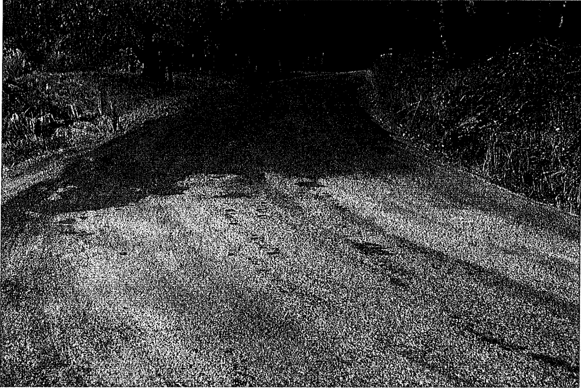
Photo 9. Mile 0.8: 30-ft road width with 1-ft shoulders.
