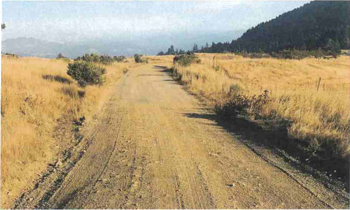
Photo 15. Mile 1.3: 16-ft road width with 2-ft shoulders.
