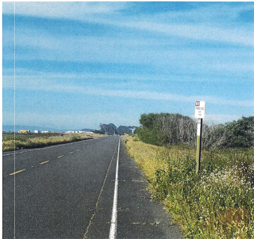
ABOVE: EXAMPLE OF EXISTING NO PARKING SIGN ON NEW NAVY BASE ROAD NO PARKING SIGNS ARE PROPOSED TO BE INSTALLED APPROXIMATELY 3 FEET FROM EDGE OF PAVEMENT. SIGNS TO BE INSTALLED AT THE BEGINNING POINTS AND ENDING POINTS OF THE PARKING ZONES. WHEN A PARKING ZONE IS LONGER THAN 800 FEET, ADDITIONAL SIGNS WILL BE PLACED APPROXIMATELY 400 FEET APART. SIGNS ARE TO BE PLACED IN SUCH A MANNER AS TO BE VISIBLE TO THE PUBLIC TO ENSURE PARKING REGULATIONS ARE OBSERVED. APPROXIMATELY 150 SIGNS WILL BE INSTALLED ALONG 4.642 MILES OF ROAD.
