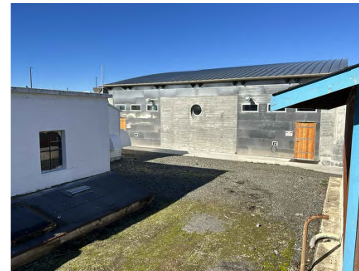
6 EXISTING VAULT, GENERATOR ROOM, AND ARFF STATION SCALE: NTS
