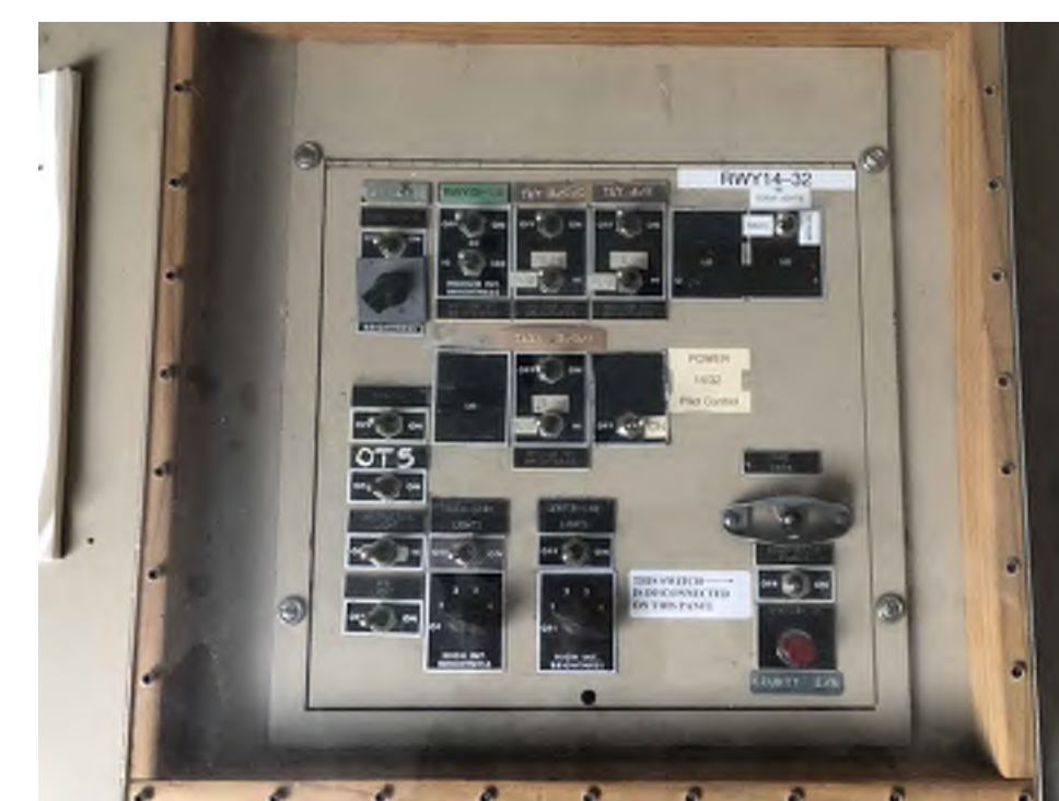
3 PILOT CONTROL SWITCHES SCALE: NTS
