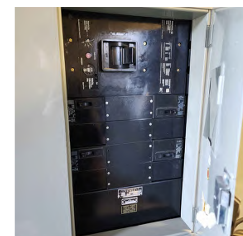
3 MAIN BREAKER PANEL SECTION 1 SCALE: NTS
