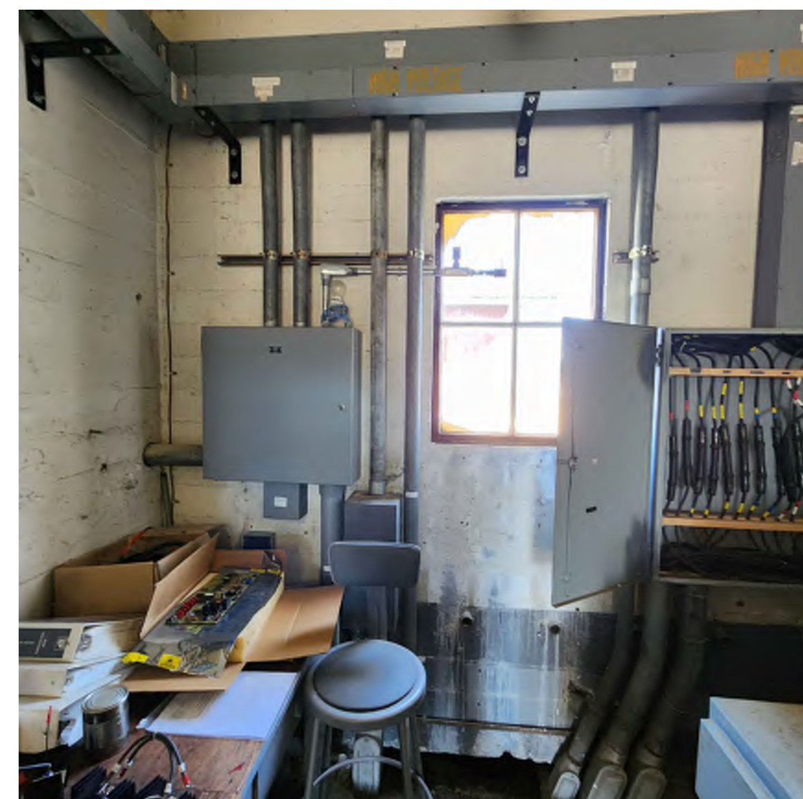
7 EXISTING VAULT INTERIOR SCALE: NTS
