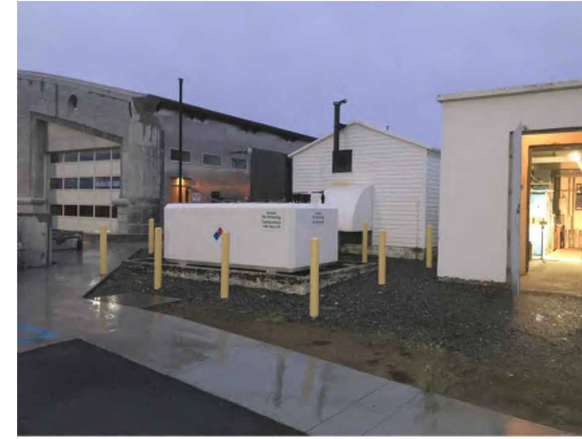
3 EXISTING VAULT ENTRANCE SCALE: NTS
