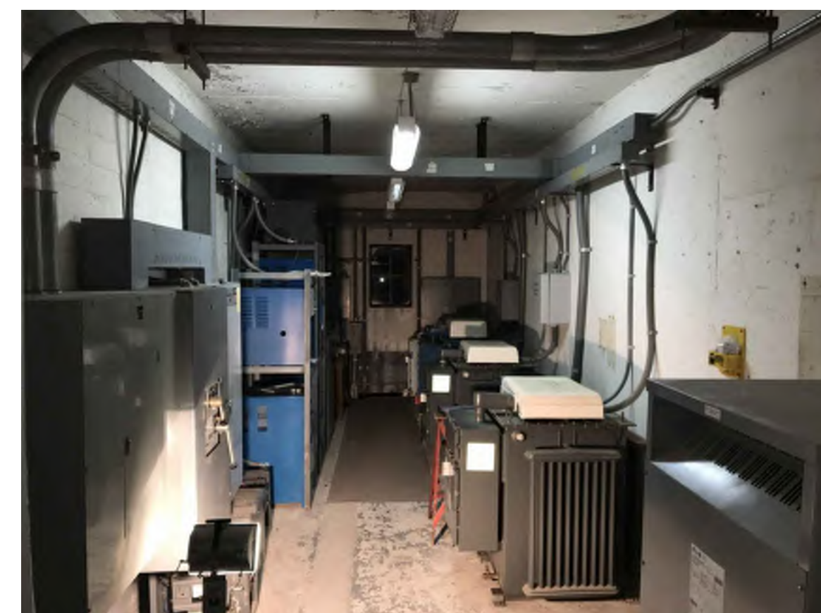
7 EXISTING VAULT INTERIOR SCALE: NTS
