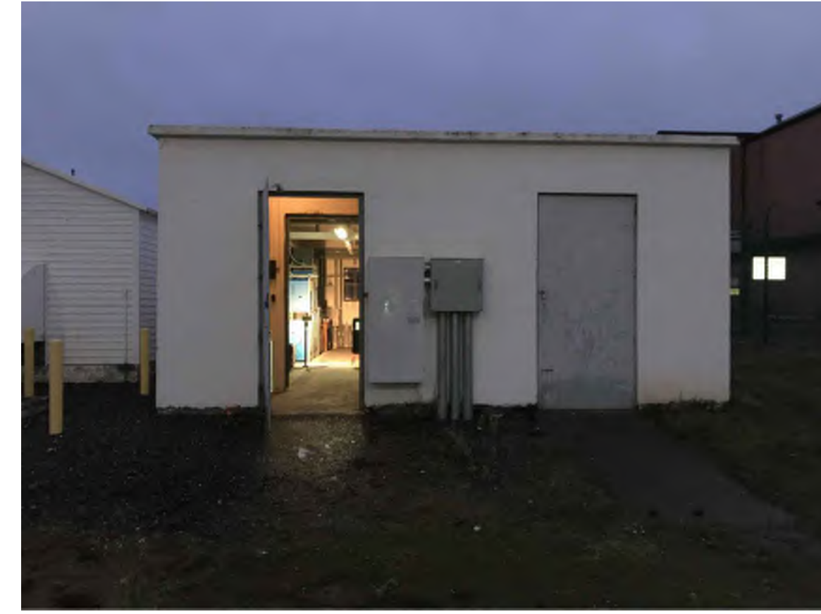
2 EXISTING VAULT ENTRANCE SCALE: NTS
