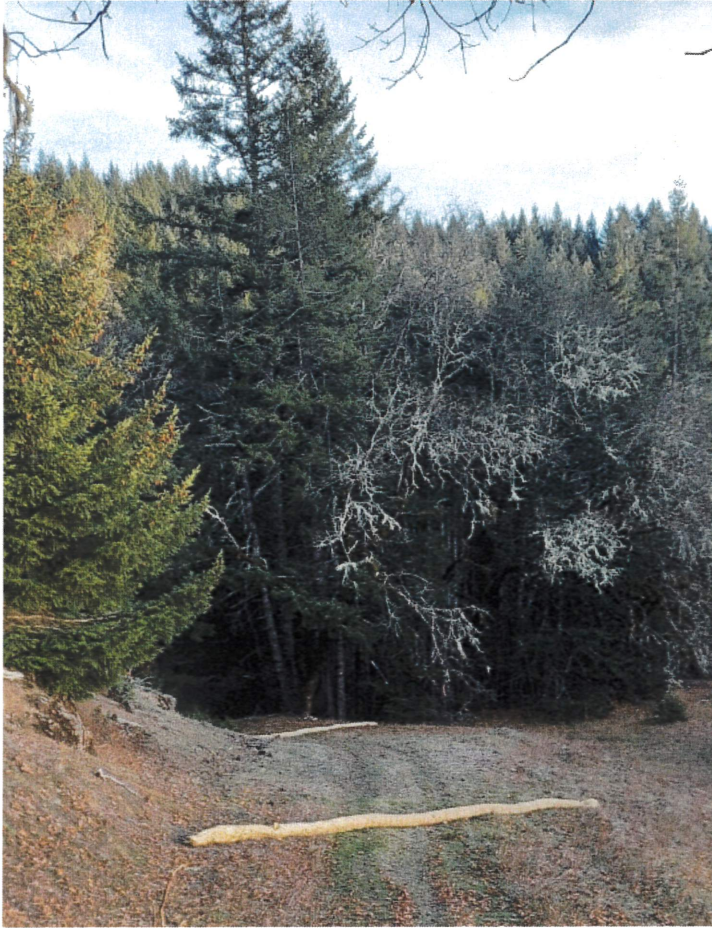
Photo 3 & 4. Photographs of straw waddles installed on the secondary road. The water break spacing meets the specifications pursuant to the Handbook for Forest, Ranch and Rural Roads .
