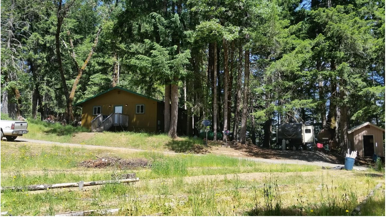
Photo 16. Residential area N side (primary residence), Site A; generator shed to right of photo
