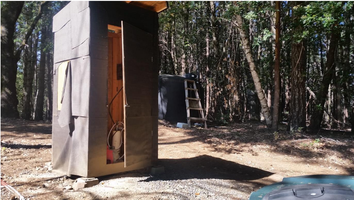
Photo 13. Well, well shed and tanks at Site D
