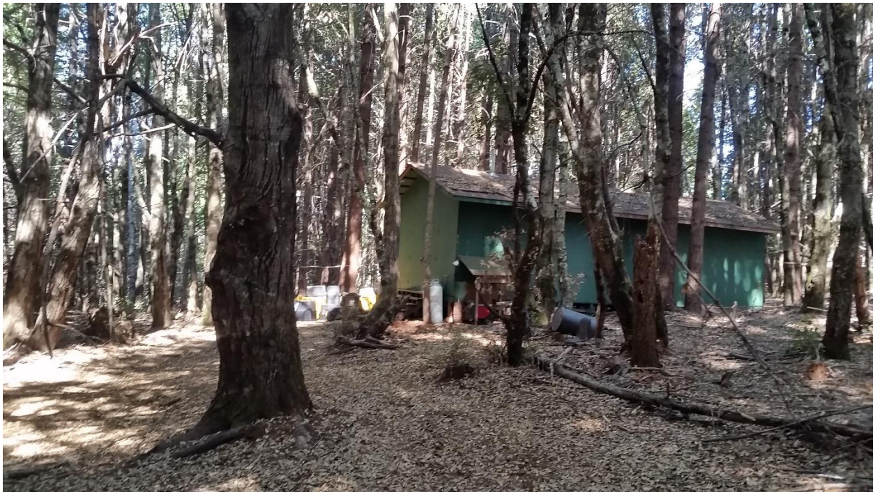
Photo 15. Processing/Drying building at Site E - generator in lean-to.
