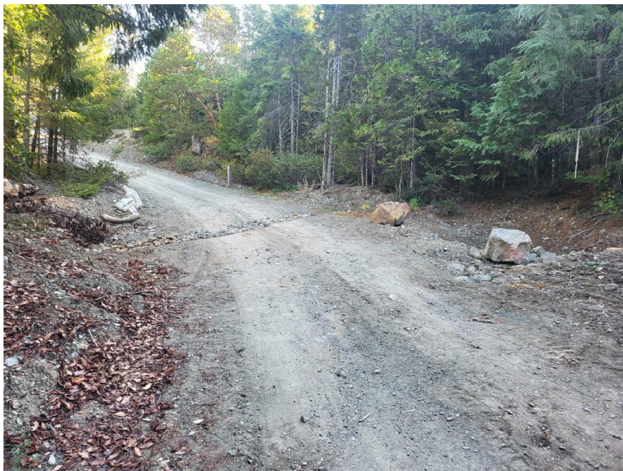
Figure 50: MP20 culvert and water bar.
