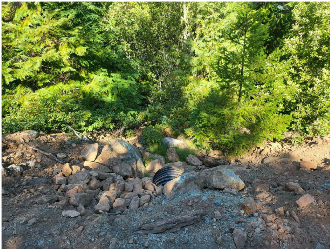
Figure 6: MP3 24" culvert outlet.
