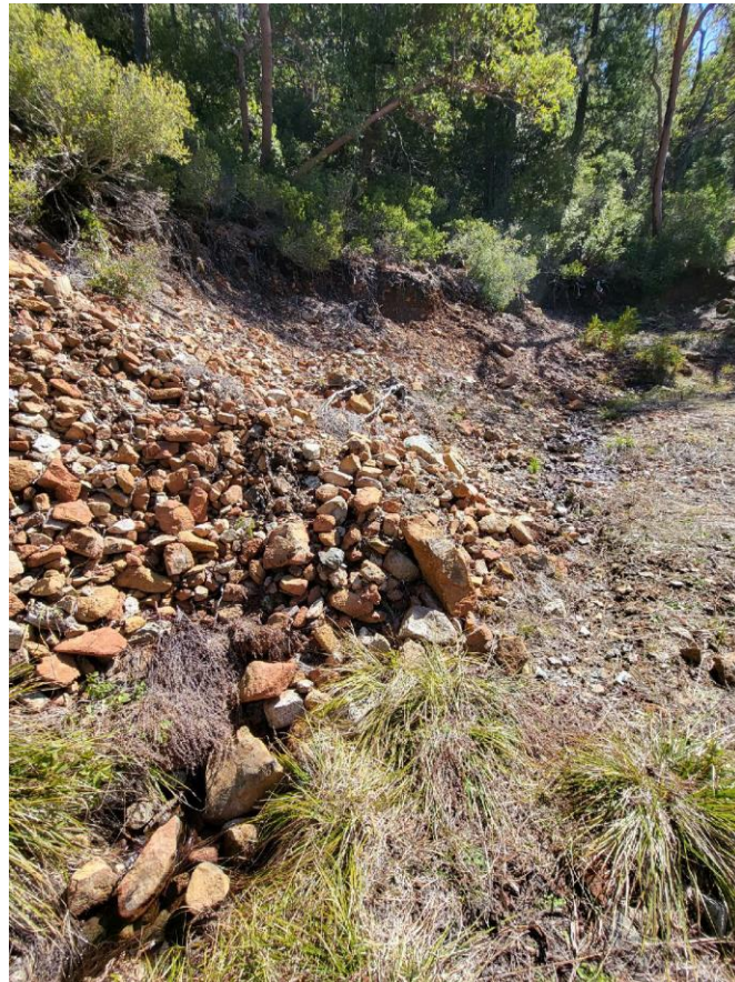
Figure 22: MP8 perched unstable fill removed.
