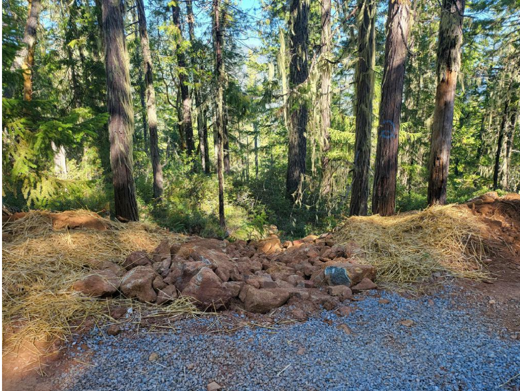
Figure 3: Rock armor placed downstream of MP2.
