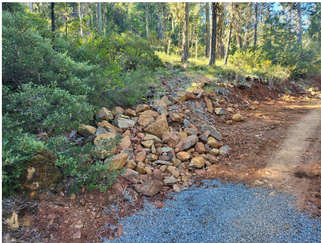
Figure 2: Rock placed upstream of rocked ford crossing.
