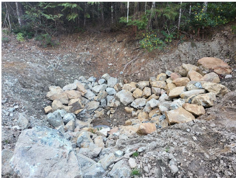
Figure 51: MP20 culvert inlet.
