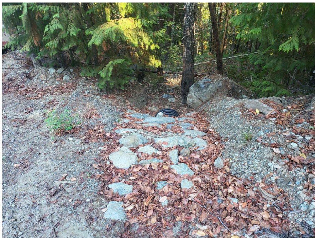
Figure 52: MP20 culvert outlet.
