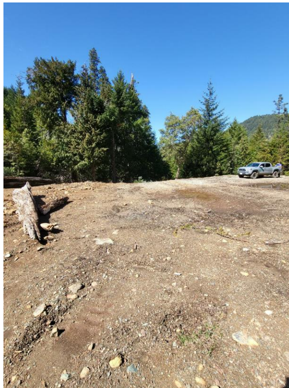
Figure 24: MP8 all trash removed.
