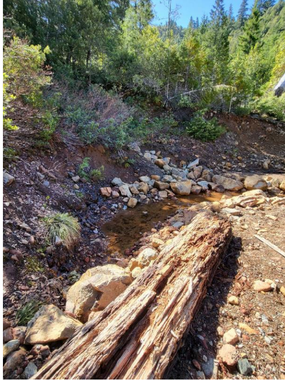
Figure 25: MP8 stream channel excavation to connect spring flow to Class II channel.
