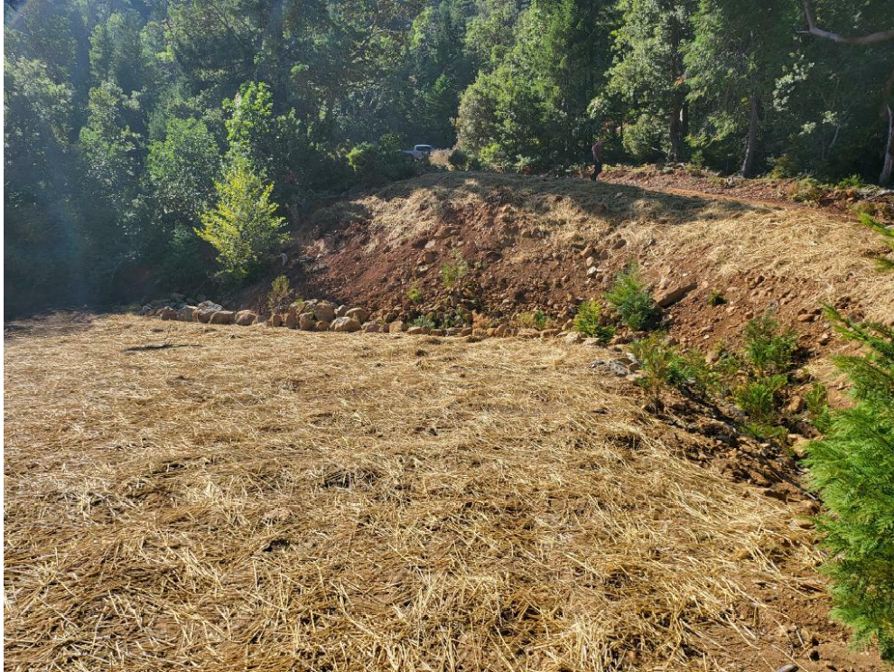
Figure 43: MP13 slope pulled back, stream restored with revegetation efforts currently succeeding as of 10/5/2022.
