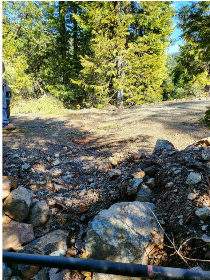
Figure 14: MP6 replaced 24" culvert.
