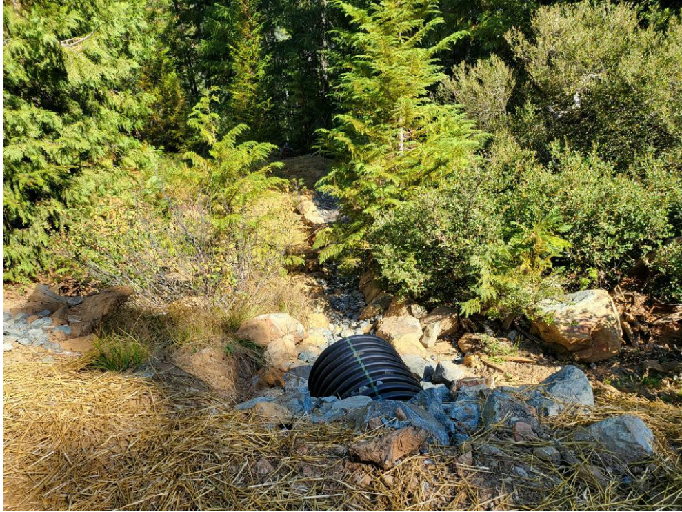
Figure 33: MP10 outlet with reconstructed channel.
