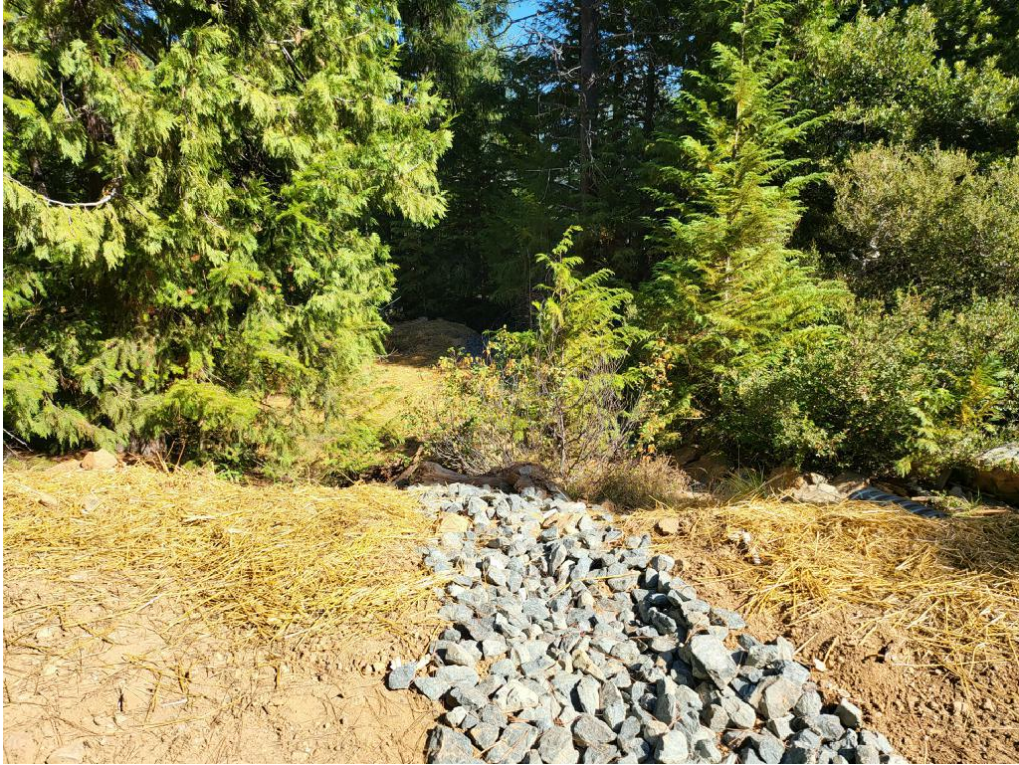
Figure 35: MP10 disconnected road surface from watercourse.
