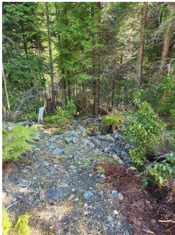
Figure 46: MP14 rock armor.
