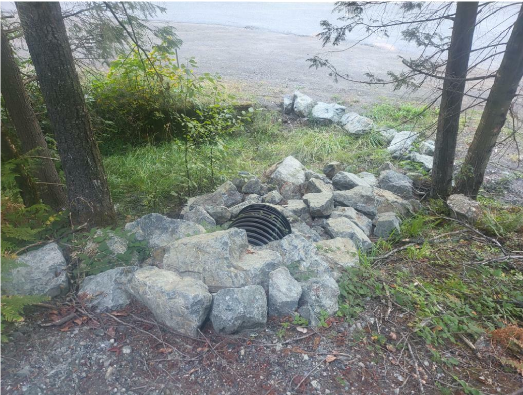
Figure 54: MP21 culvert outlet.
