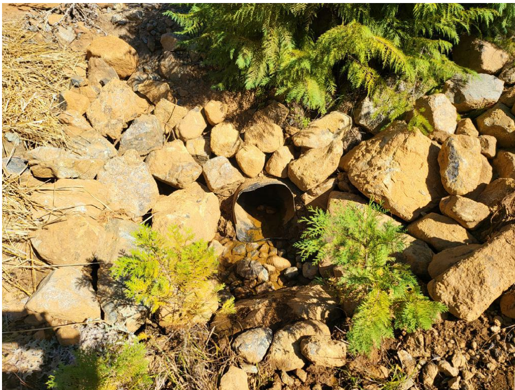
Figure 44: MP13 cleared culvert inlet.
