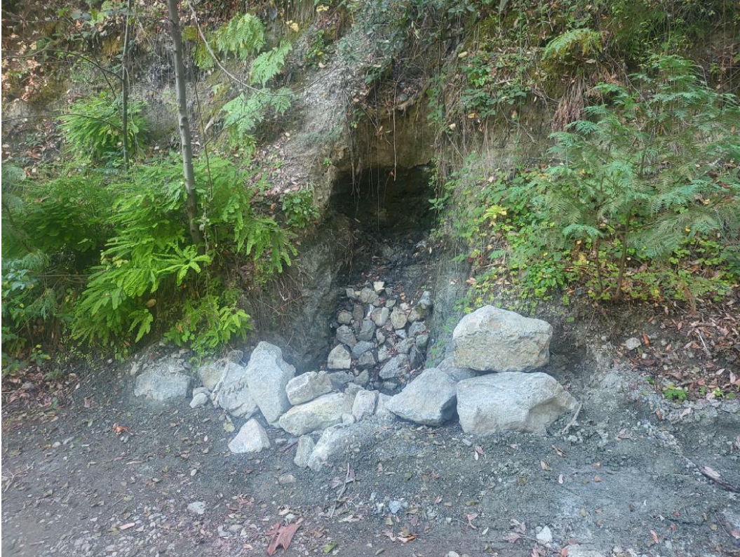
Figure 53: MP21 culvert inlet.
