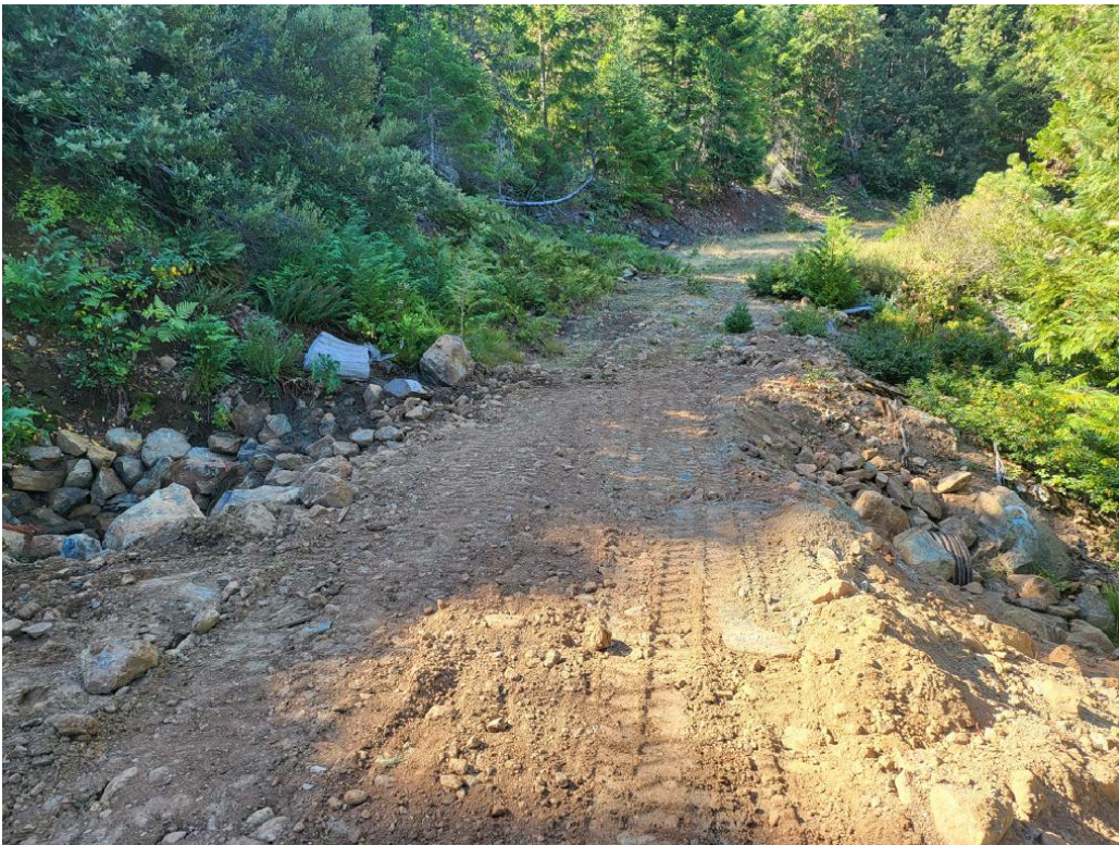
Figure 4: MP3 replaced 24" culvert.
