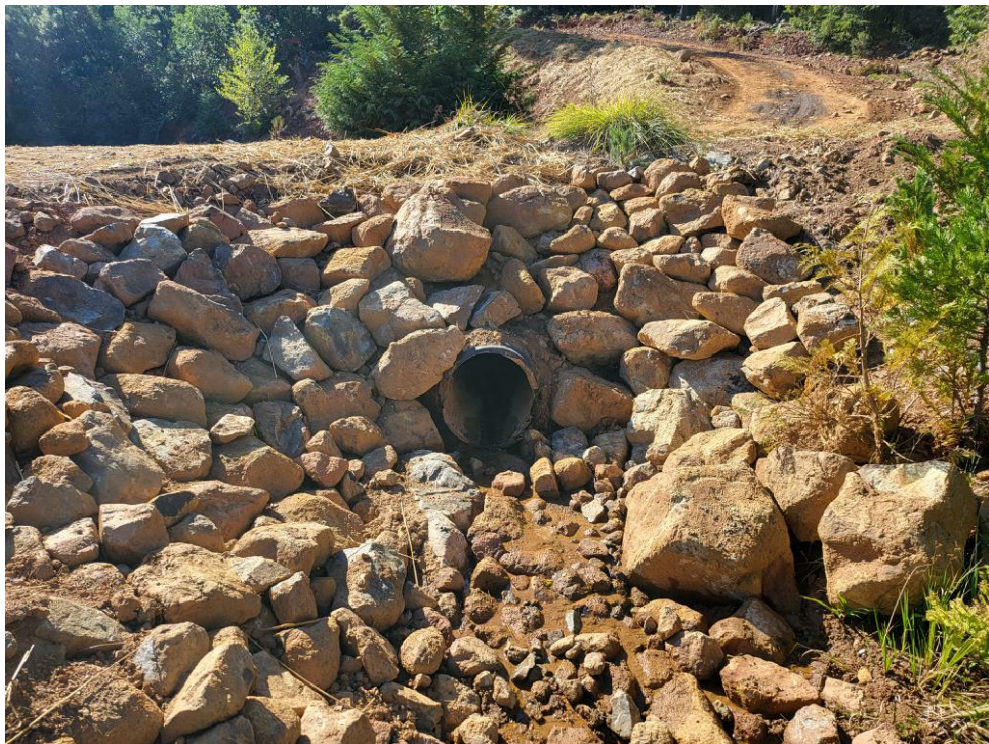
Figure 42: MP13 culvert outlet.
