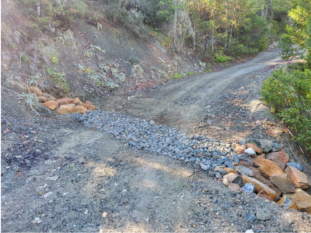
Figure 27: MP9 installed rock armor.
