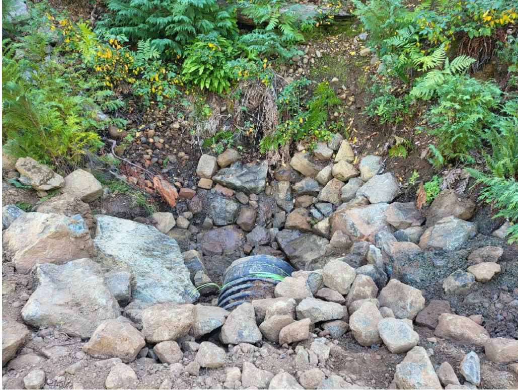
Figure 5: MP3 24" culvert inlet.
