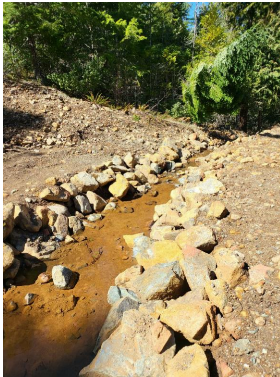
Figure 26: MP8 stream channel excavation to connect spring flow to Class II channel.
