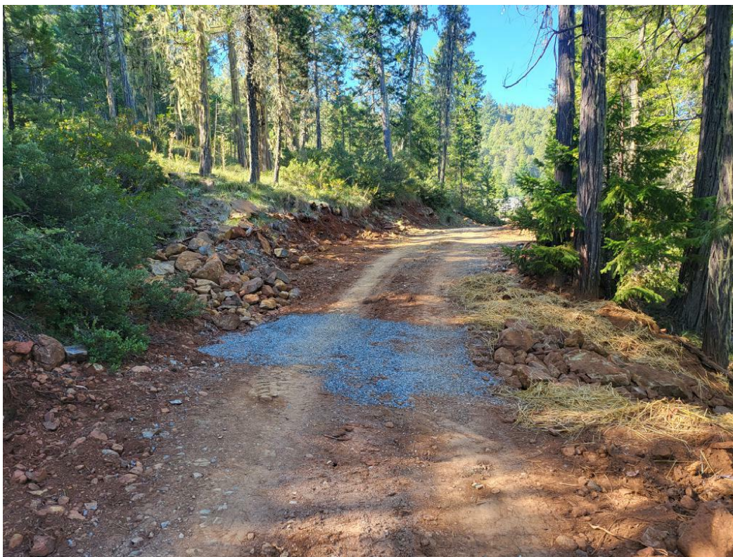
Figure 1: MP2 Installed Rocked Ford.
