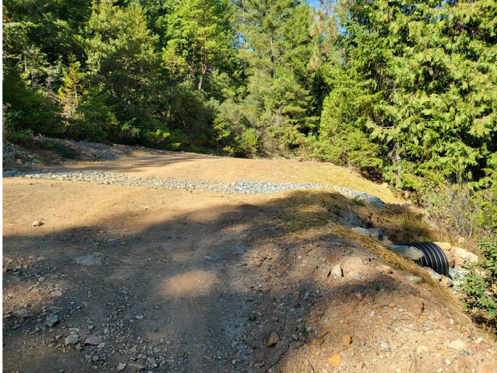
Figure 31: MP10 replaced culvert and rocked road surface.
