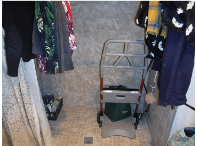
38. Accessible unit shower enclosure.
