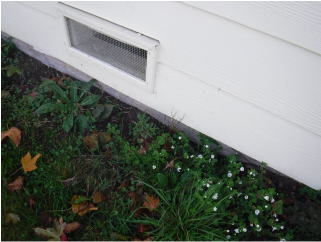
13. Crawl space ventilation and concrete stem wall.
