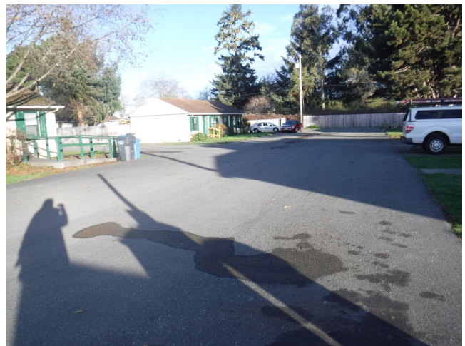
4. Typical condition of the asphalt paving and landscaping.
