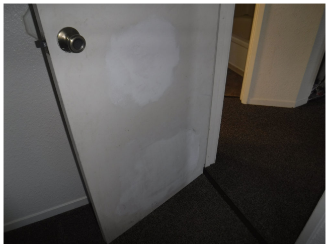
42. Repaired damaged to interior door and carpeting at living areas.
