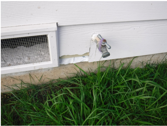
21. Damaged siding.
