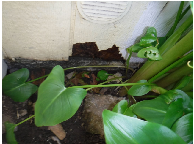
22. Damaged siding
