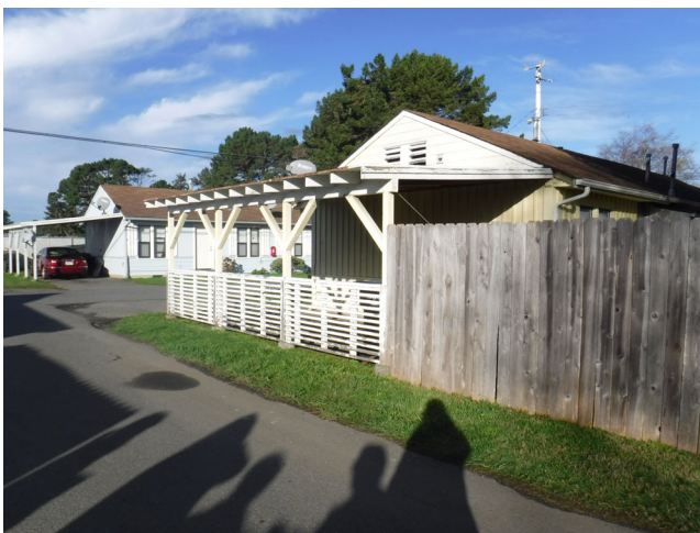
5. Typical carport, fencing, and landscaping.
