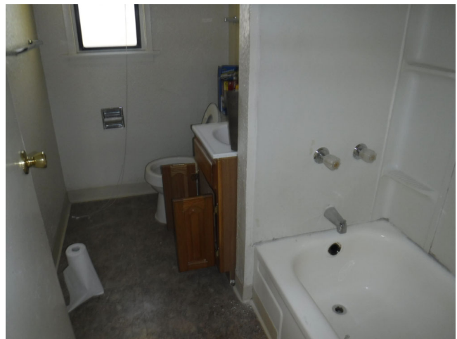
36. Vacant unit bathroom being turned over.
