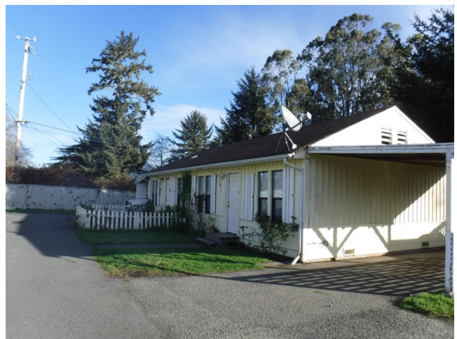
12. Typical building construction
