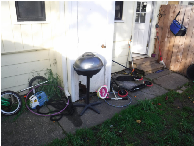
23. Damaged water heater enclosure door and typical rear entry to the units.
