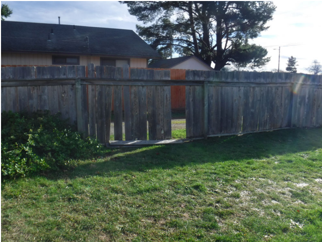
9. Damaged and missing site fencing.
