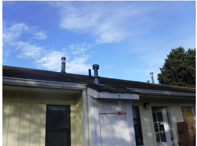
16. Typical older roofing conditions. Note exterior water heater closet.
