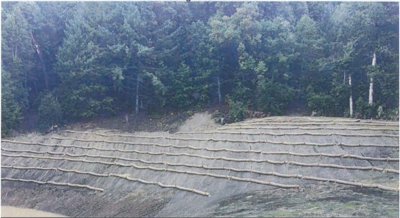
Jute netting & Straw-wattles
