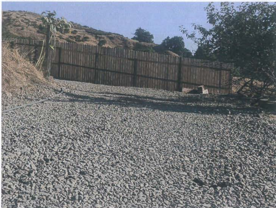
Well rocked permanent road.
