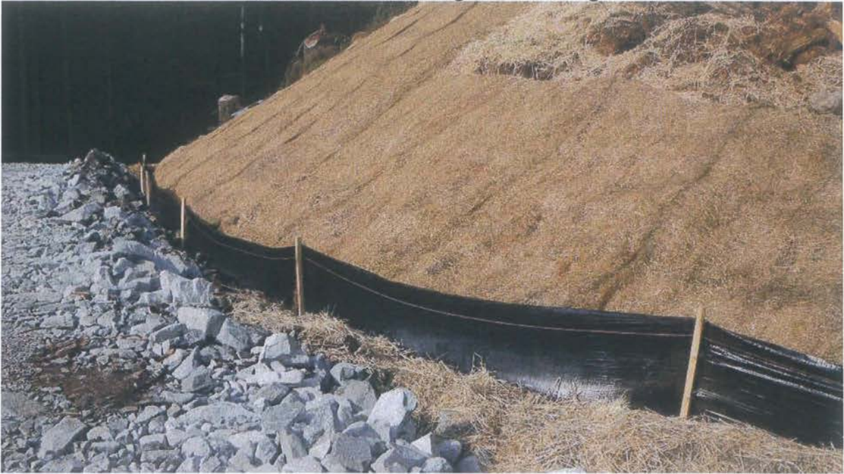
Erosion Control Matting & Silt Fencing
