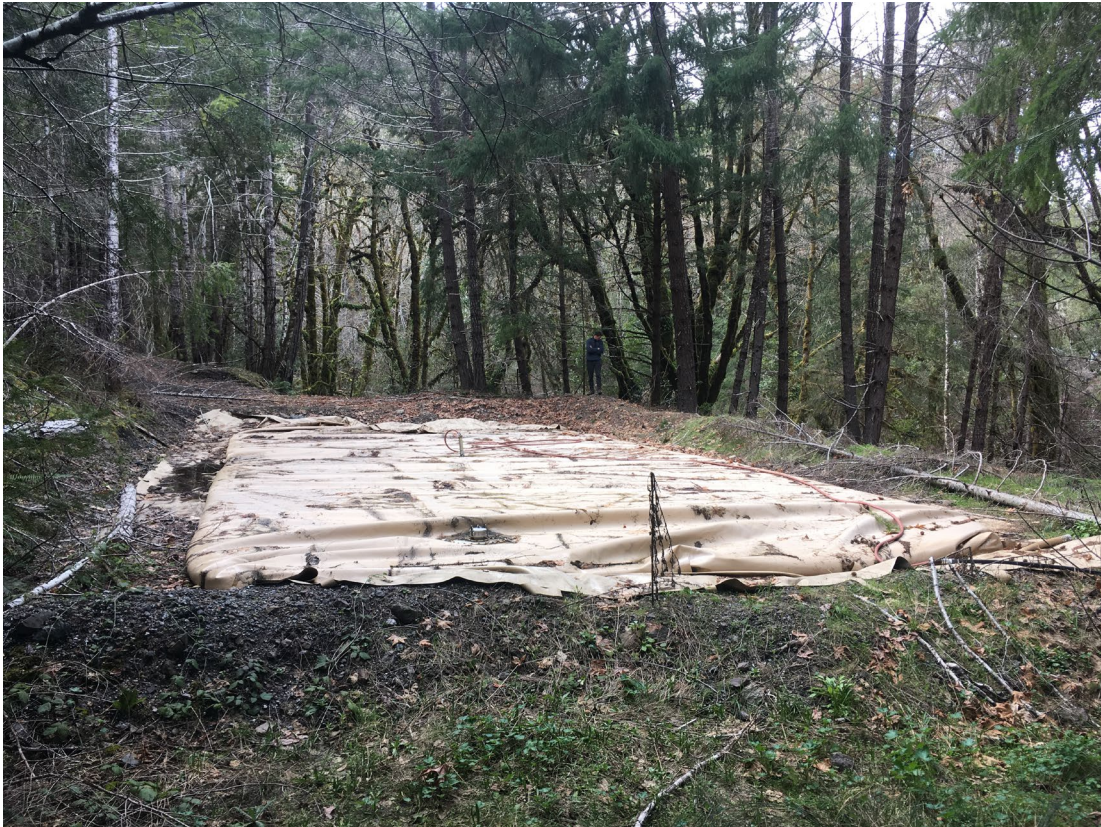
Photo 9. Site B – Looking west from east edge.
