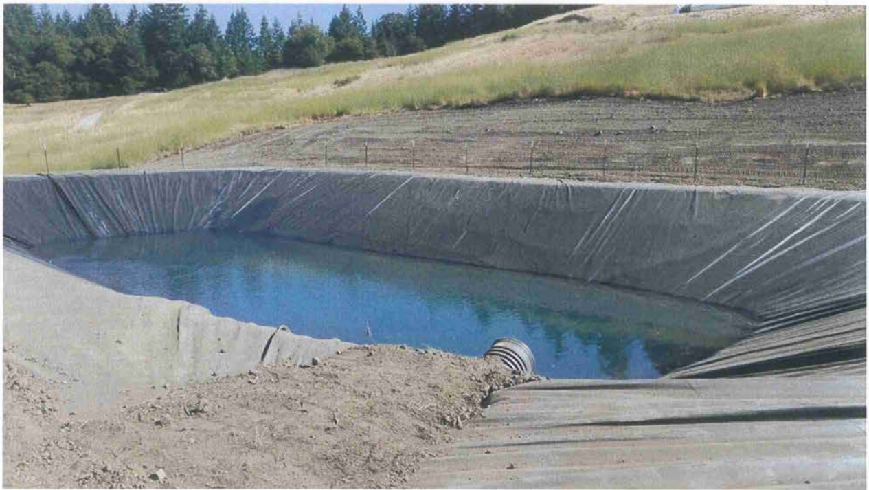
Picture 7: 350,000-gallon rain catchment pond. Photo date 7-06-2017.
