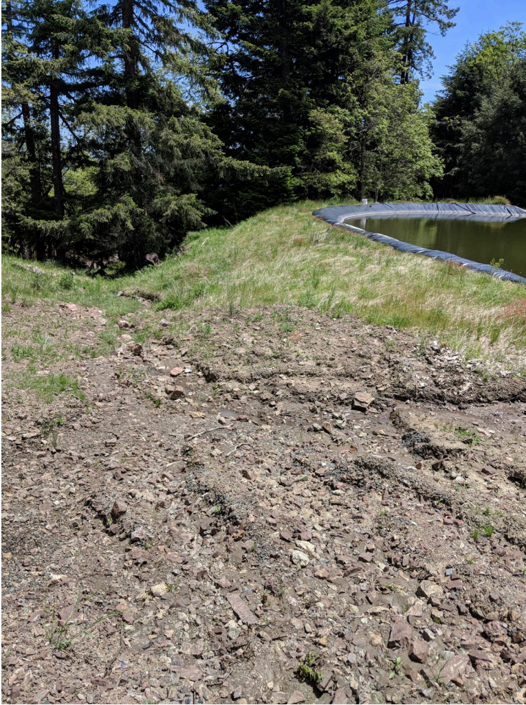
Photo 9. Erosion was observed around the upper pond on the west side of the property and appeared to be causing sedimentation in the stream course. Revegetation is recommended after work on the stream crossing is completed.
