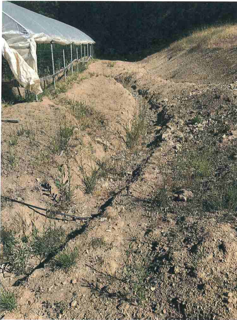
Photo 11. Observation Point 2(b) – drainage ditch constructed to drain cultivation area off of fill slope at Conversion Area #2.
