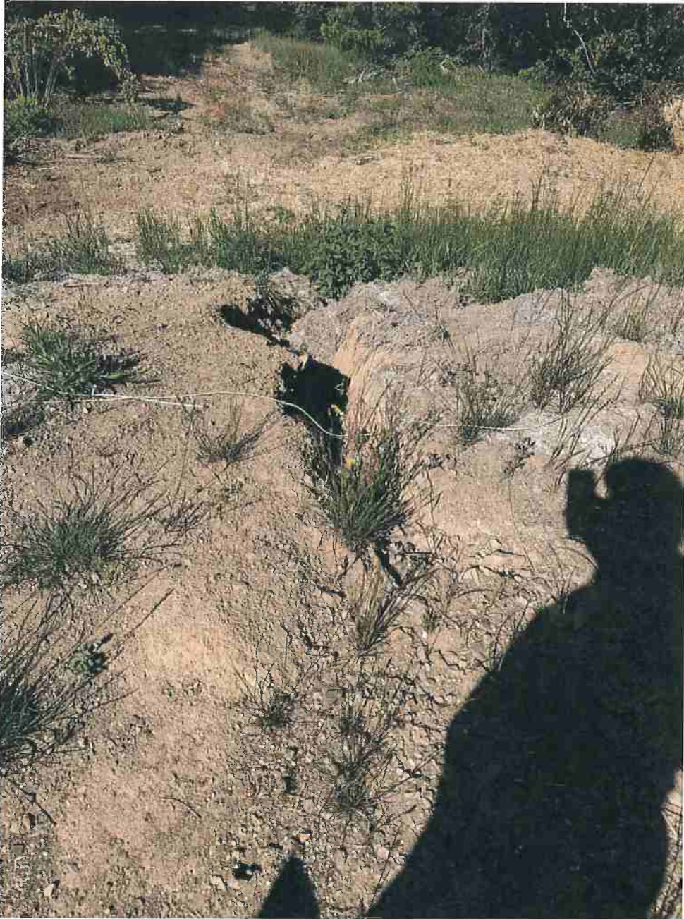
Photo 10. Gullying/rutting occurring along the fill slope of grading above Conversion Area #2 (Observation Point 2(b)) from water running off of the graded area.
