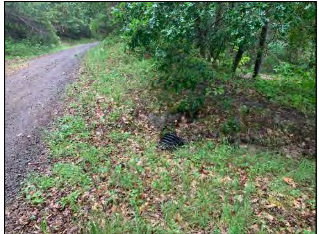
Photo #130 Private Access Rd Looking @ 12" Culvert Out
