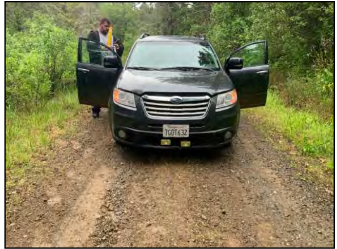
Photo #128 Private Access Rd Width 10'8" Slope 16.3%
