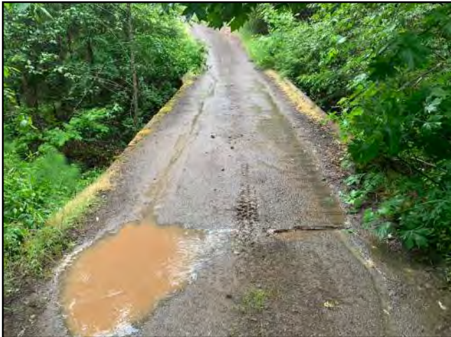
Photo #135 Private Access Rd @ Steel Bridge Looking SW
