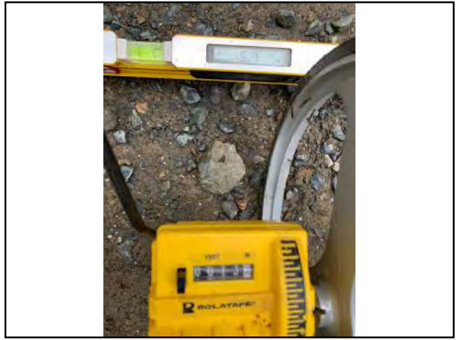
Photo #230 Stewart Ranch Rd Width 13'8" Slope 15.7%
