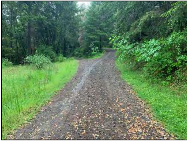
Photo #133 Private Access Rd @ Pullout Looking NE Towards Road Split
