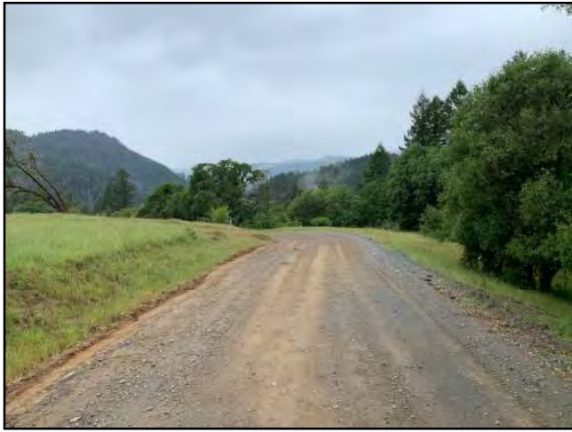
Photo #223 Stewart Ranch Rd @ Curve w/ Pullout Looking NW
