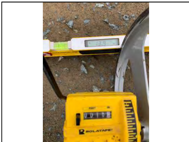
Photo #227 Stewart Ranch Rd Width 16'1" Slope 13.9%
