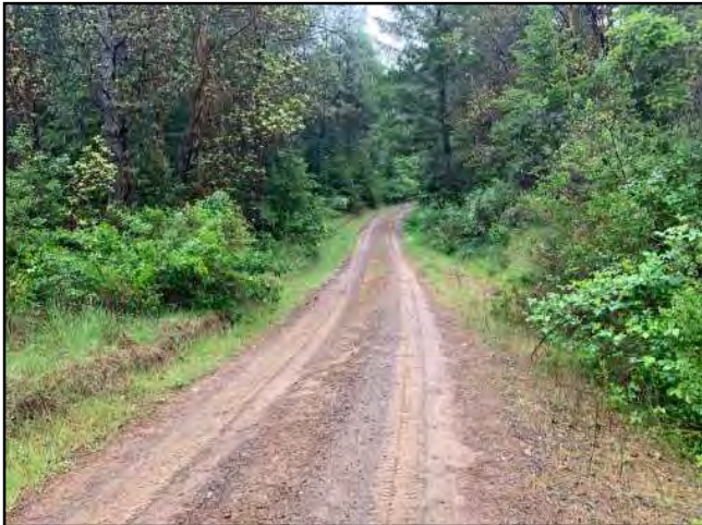
Photo #123 Private Access Rd @ Pullout Looking NE Towards Curve
