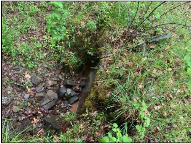
Photo #169 Private Access Rd Looking @ 12" Culvert In
