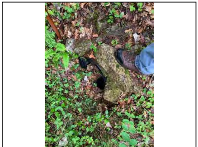
Photo #156 Private Access Rd Looking @ 12" Culvert In
