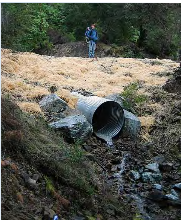
Figure 35. The culvert was replaced with a metal pipe (48 inches in diameter) at the correct slope. The road surface was lowered, reducing the fill volume by 100 cubic yards. The outlet and fill were armored to prevent future diversion. Photo: Jared Gerstein.
