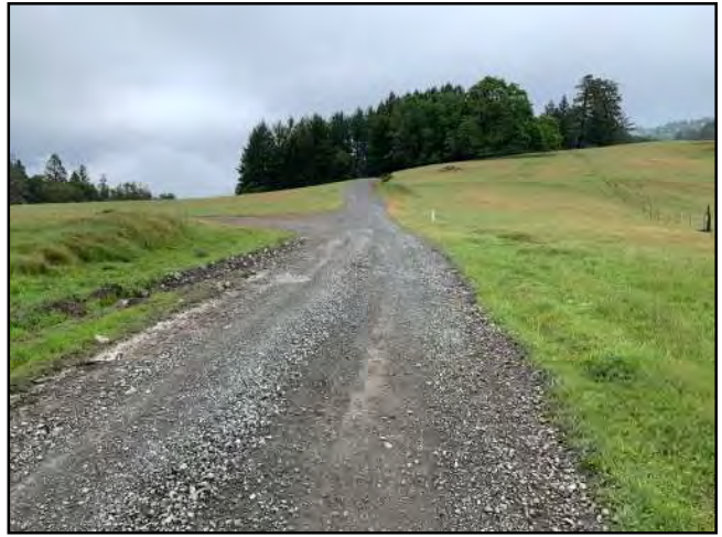
Photo #200 Stewart Ranch Rd Looking NE Back Towards Private Access Rd
