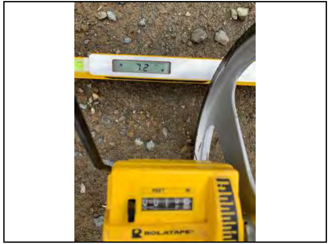
Photo #224 Stewart Ranch Rd Width 16'0" Slope 7.2%
