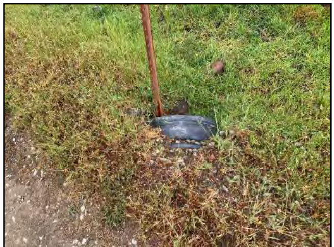
Photo #192 Private Access Rd Looking @ 18" Culvert In
