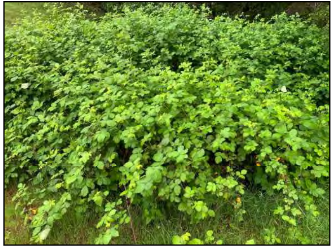
Photo #182 Private Access Rd Looking @ Clogged Culvert In (Size Unknown)
