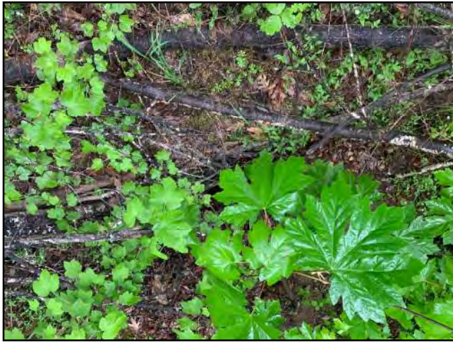
Photo #13 Private Access Rd APN 216-202-009 Looking @ Clogged Culvert In(Size Unknown)
