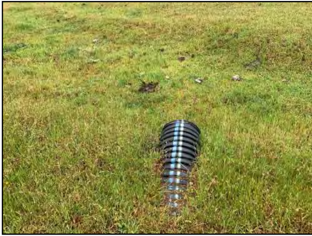
Photo #199 Private Access Rd Looking @ 12” Culvert Out
