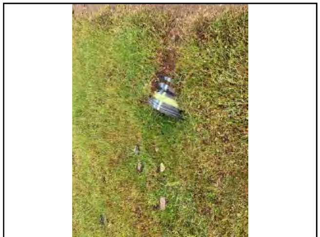
Photo #198 Private Access Rd Looking @ 12” Culvert In
