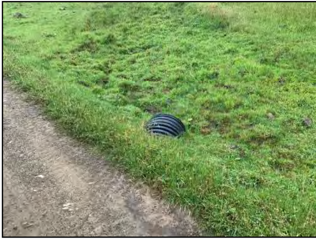
Photo #193 Private Access Rd Looking @ 18” Culvert Out
