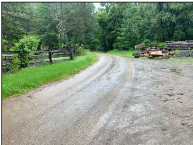
Photo #143 Private Access Rd @ Turnaround Area Looking NE
