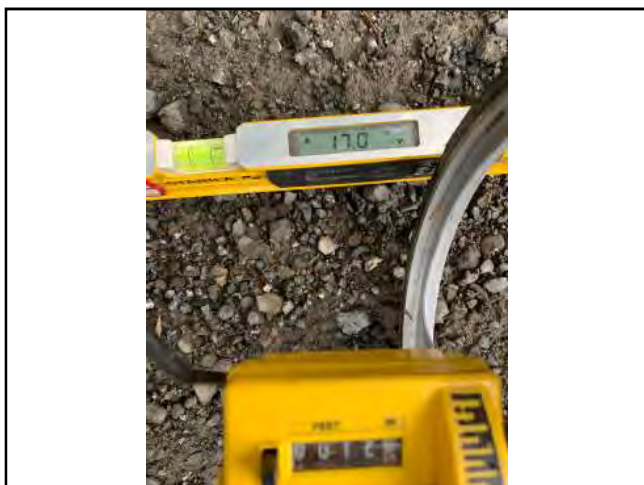
Photo #239 Stewart Ranch Rd Width 12'2" Slope 17.0%
