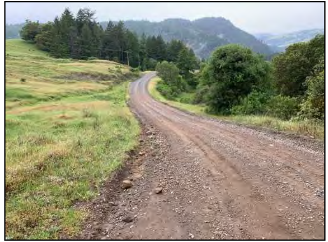
Photo #218 Stewart Ranch Rd @ Curve w/ Pullout Looking NW
