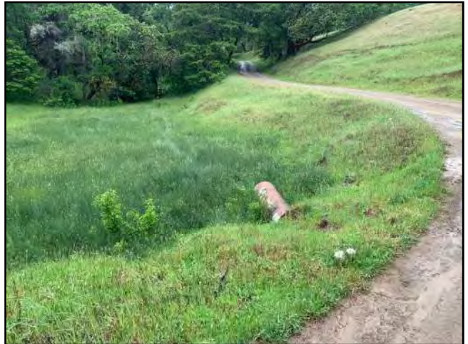
Photo #184 Private Access Rd Looking @ 18" Culvert Out
