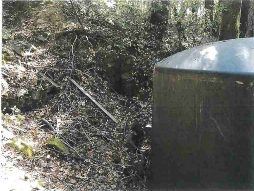
Photo 3. Water tank at shallow well.
