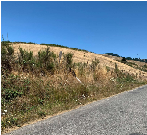
Sign post in ditch
