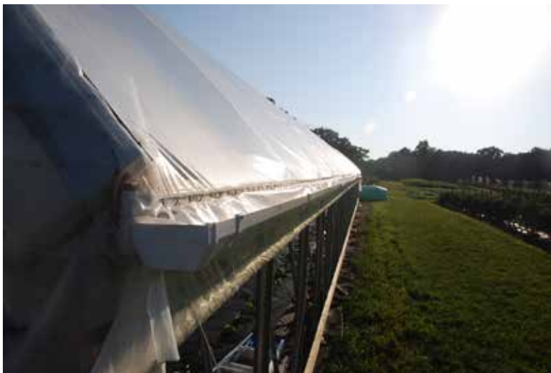
Hoop house Figure C: Gutter drains to tank
