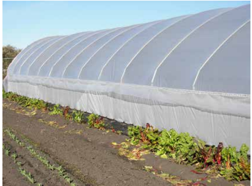
Hoop house Figure A: Filter fabric along roofline
