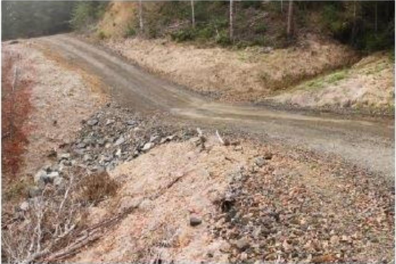
**FIGURE 120.** *This armored fill crossing of a steep, ephemeral stream was constructed to provide a low maintenance crossing. The crossing has been deeply dipped to reduce the volume of road fill and to eliminate the potential for stream diversion. The fill slope has been heavily armored through the axis of the crossing to contain flood flows and prevent down-cutting. Armored fills cannot be used on fish bearing streams.*
