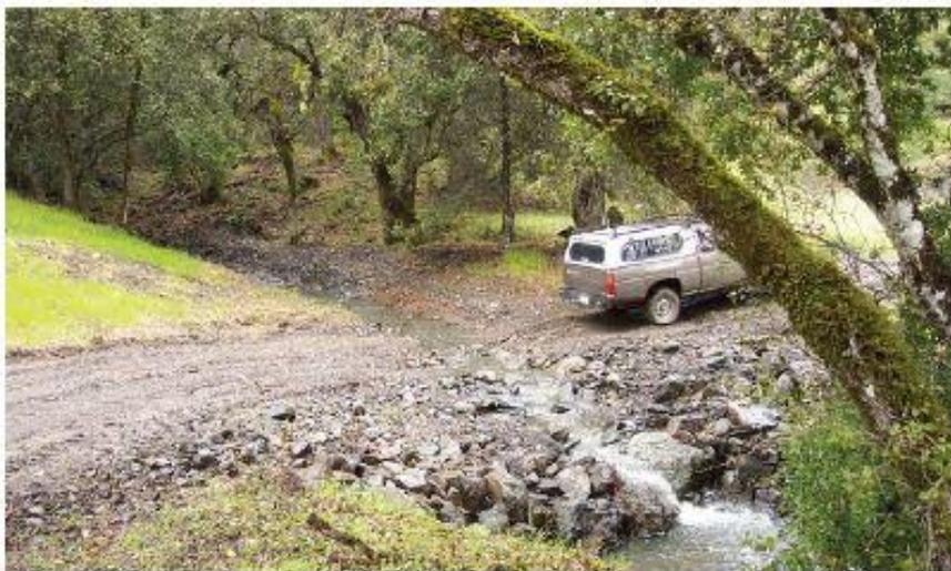
**FIGURE 121F.** The same armored fill as it appeared after the first winter flood flows. No maintenance was required to reopen the road. It is also clear that no stream diversion is possible at this stream crossing site, and the volume of fill within the crossing has been reduced to the minimum amount needed to maintain a relatively smooth driving surface on this low volume road.
