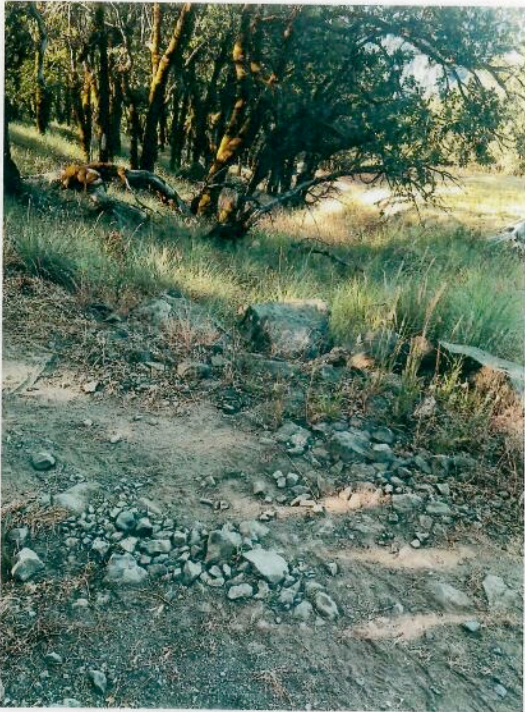
Outlet of Rock Ford – Crossing #1. Note pulverized rock and dust, which shall be addressed by adding more surface rock to the approaches. Photo date: 7-16-2019
