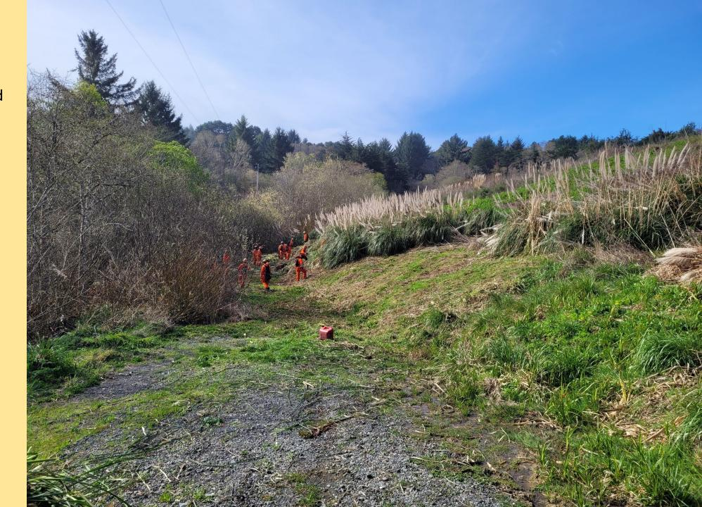
An up-close photo showing how much the willows have encroached onto the cap and hid features like this stand-up pipe. Once construction started for the cap remedial project, we found that the subterranean leachate collection system extends, farther than anticipated, towards the riparian corridor. Removal of the smaller willows to keep roots from potentially breaking pipes that convey the leachate to the leachfield was conducted during the construction phase under the supervision of David Orluck.
