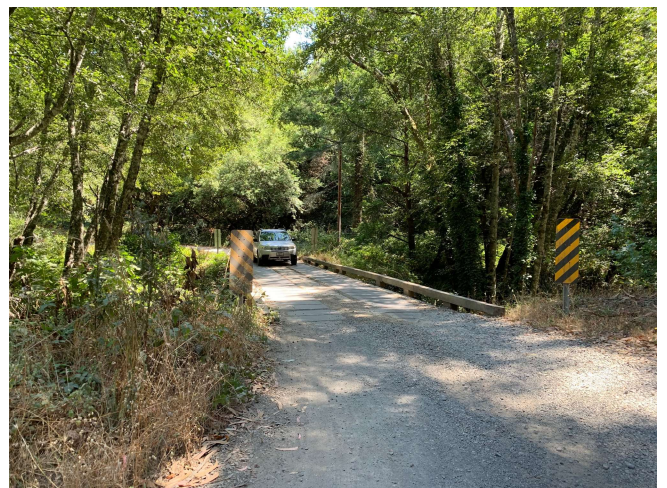
Low curb on one-lane bridge
