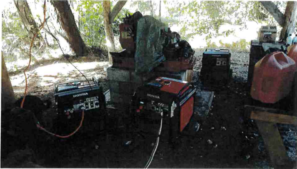
Picture 10: This is a photo of the generator area. The discharger utilizes three Honda generators to provide power to the residence and cultivation sites. Five gallon fuel canisters used for temporary fuel storage can be seen in this photo. The discharger will contain these canisters in plastic tubs to ensure containment. Photo date: 09/13/2016.
