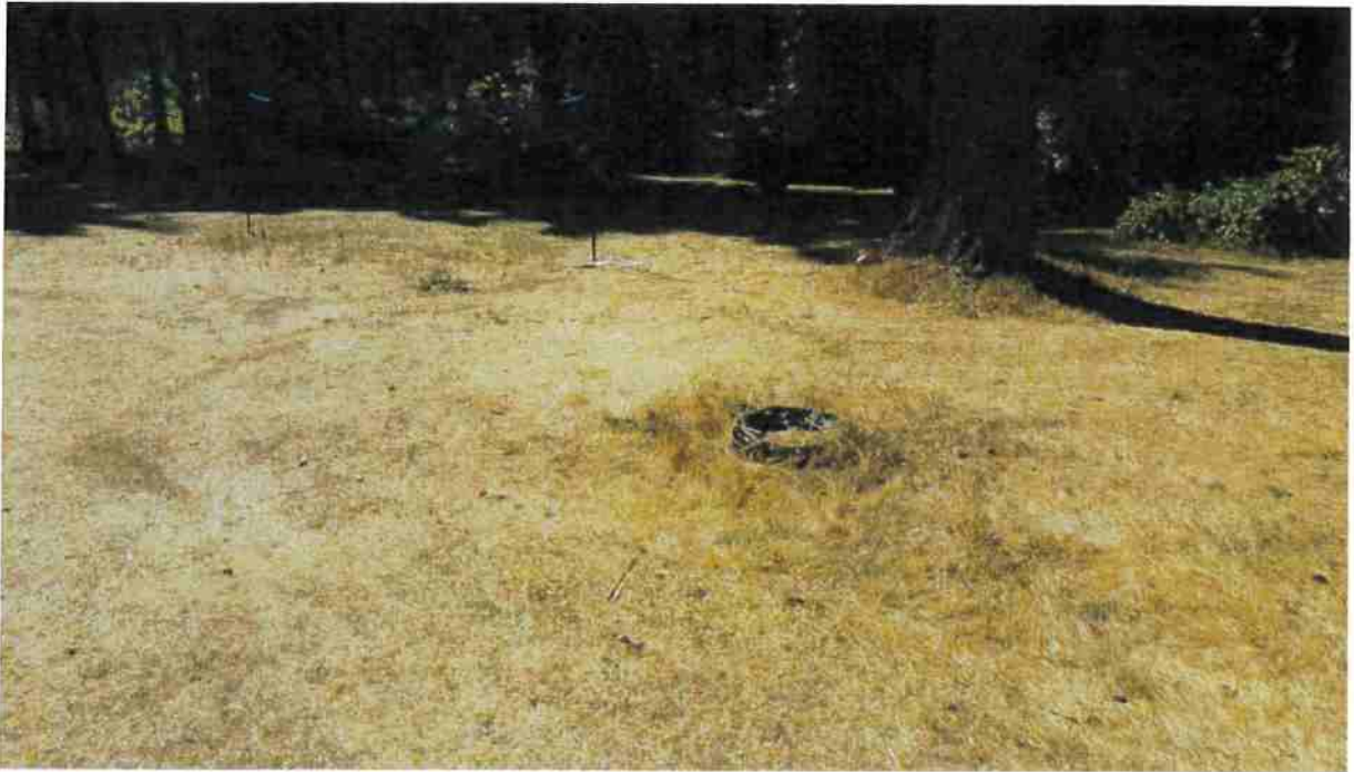
Picture 11: This is a photo of the aeration cap and leach field for the septic system associated with the residence. The tire marks the location of the septic tank while the two leach fields are located in the right side of the photo. Photo date: 09/13/2016.
