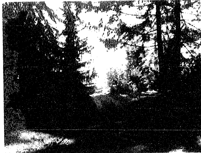
Figure RP 12. Photograph showing brush encroaching into the road that needs to be removed to provide clearance for larger vehicles, to reduce fire hazard and provide better visibility.
