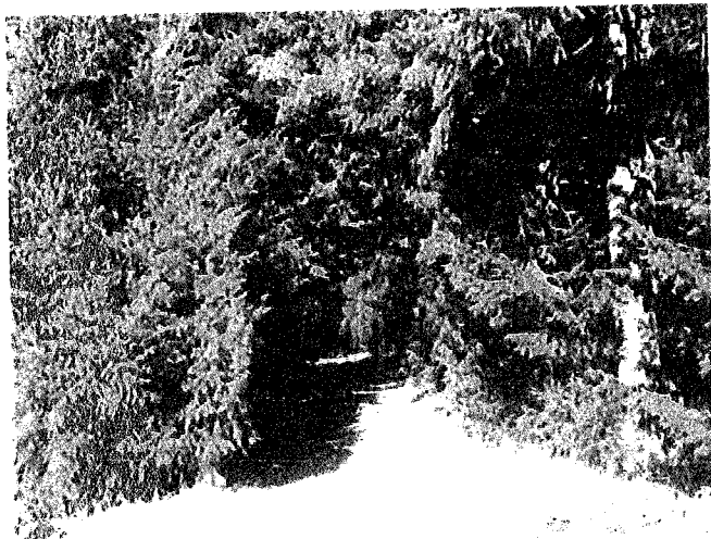
Figure RP 10. Photograph showing brush encroaching into the road that needs to be removed to provide clearance for larger vehicles reduce fire hazard and provide better visibility.
