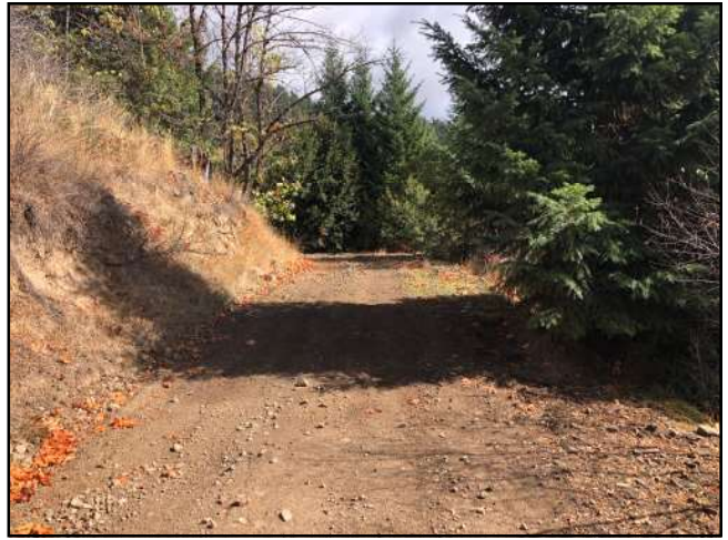
Photo #235 Private Access Rd @ Pullout Looking NE @ Curve
