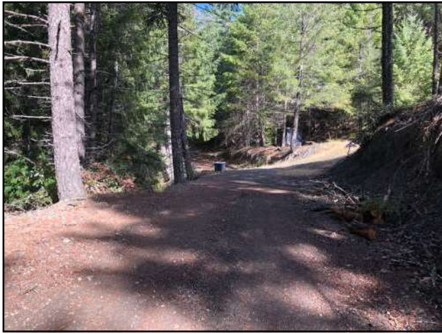
Photo #199 Private Access Rd @ Curve w/ Pullout Looking NE
