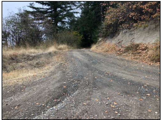
Photo #271 Private Access Rd @ Curve w/ Pullout Looking NW
