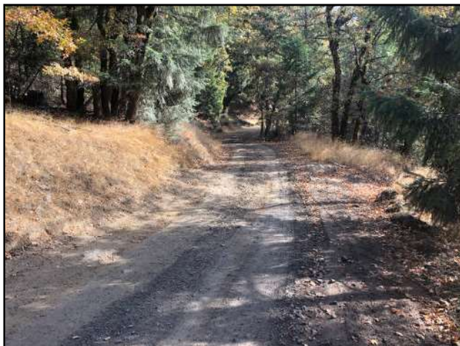
Photo #113 Private Access Rd @ Curve w/ Pullout Looking NW
