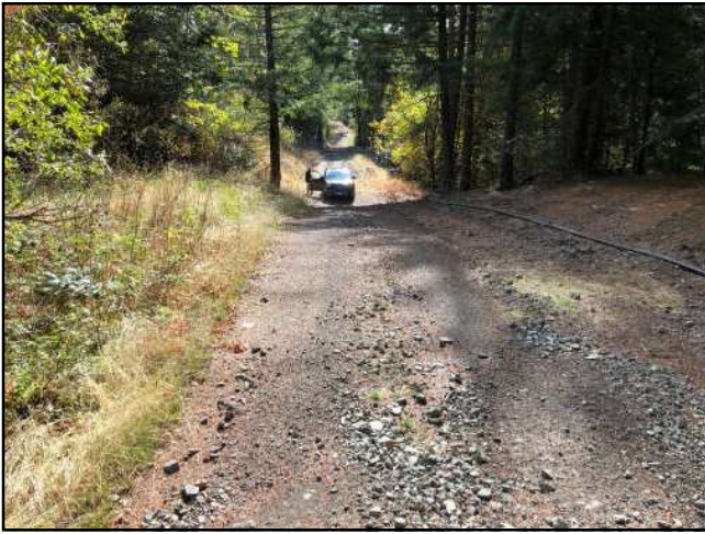
Photo #193 Private Access Rd @ Turnaround Area Looking SE
