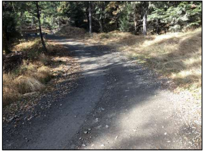
Photo #116 Private Access Rd @ Curve w/ Pullout Looking NW
