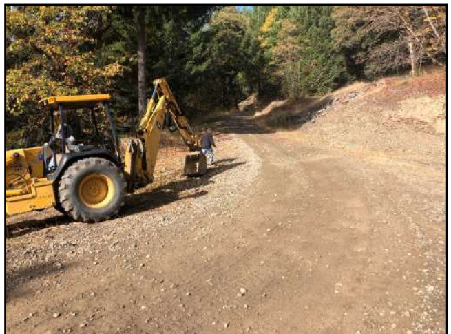
Photo #108 Private Access Rd @ Curve w/ Pullout Looking NW
