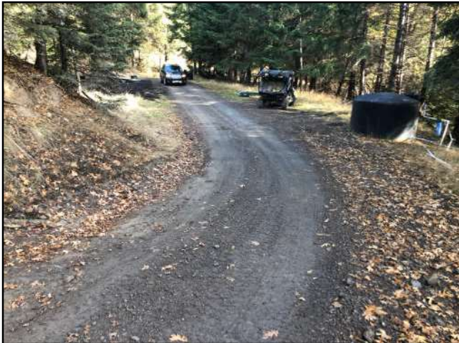
Photo #123 Private Access Rd @ Curve w/ Pullout Looking NE
