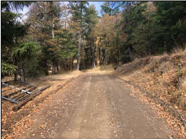
Photo #87 Private Access Rd @ Curve w/ Pullout Looking NW
