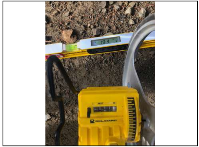
Photo #86 Private Access Rd Slope 19.3% Width 11'8"
