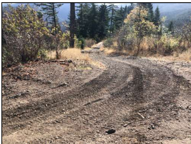
Photo #220 Private Access Rd @ Curve w/ Pullout Looking SW
