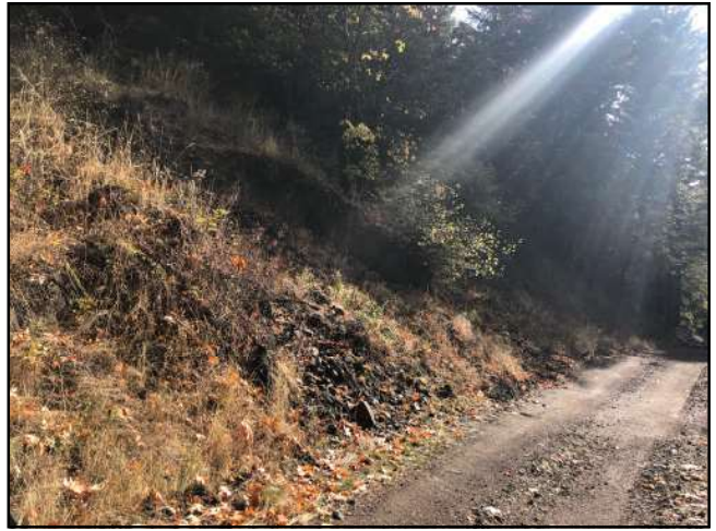
Photo #188 Private Access Rd @ Pullout Looking SE @ Hillside Slip
