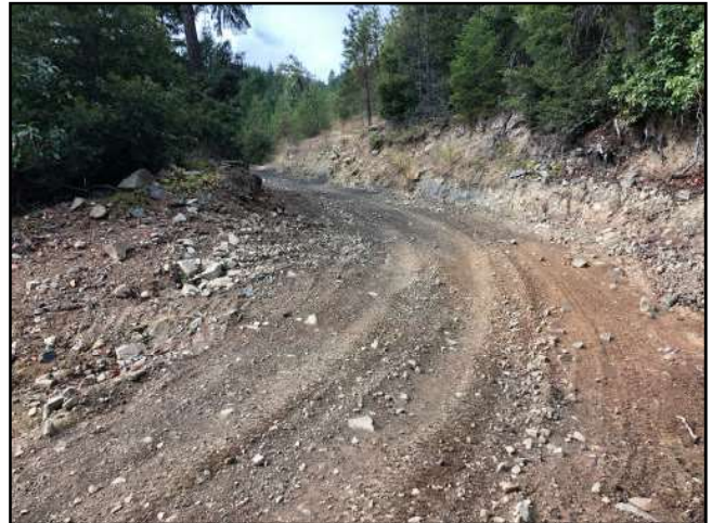
Photo #255 Private Access Rd @ Curve w/ Pullout Looking NE
