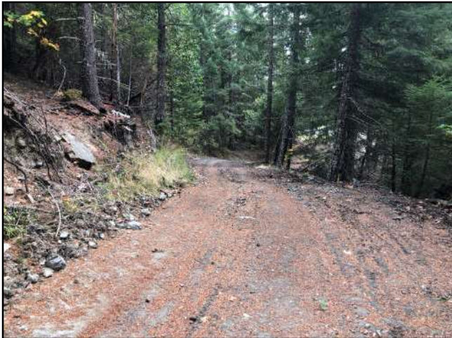
Photo #266 Private Access Rd @ Curve w/ Pullout Looking NE
