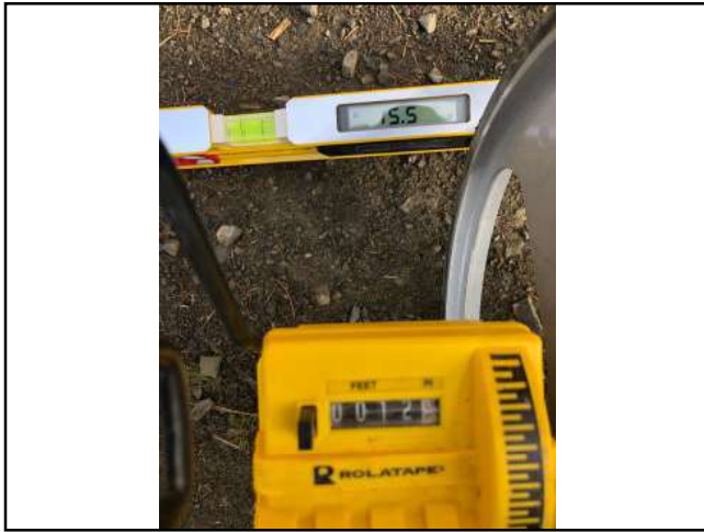
Photo #145 Private Drive Slope 15.5% Width 12'3"
