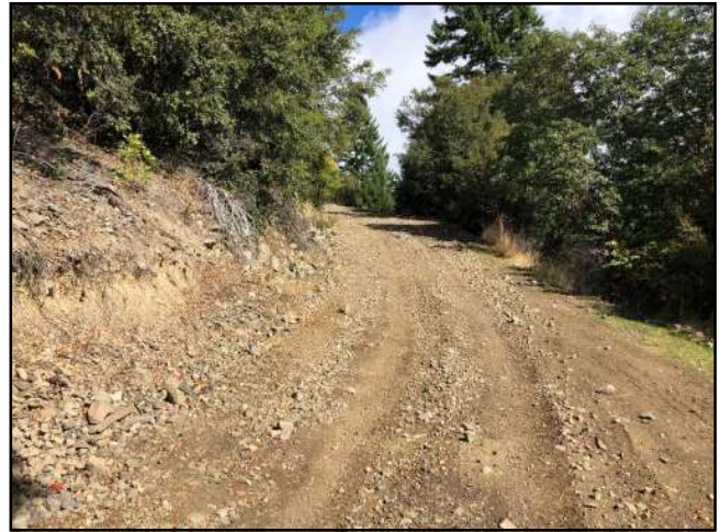
Photo #229 Private Access Rd @ Curve w/ Pullout Looking NE
