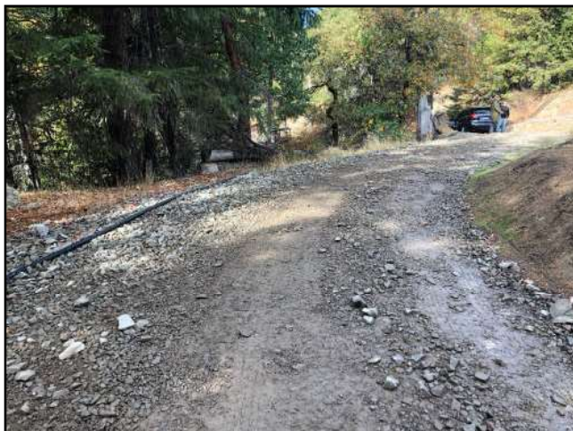
Photo #161 Private Access Rd @ Curve w/ Pullout Looking NW
