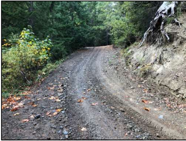
Photo #258 Private Access Rd @ Curve w/ Pullout Looking NW
