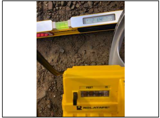
Photo #110 Private Access Rd Slope 21.4% Width 11'2"
