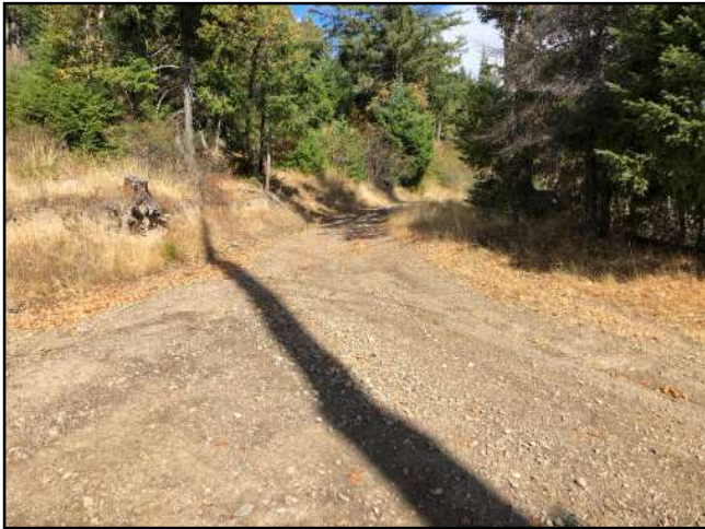
Photo #207 Private Access Rd @ Curve w/ Pullout Looking NW
