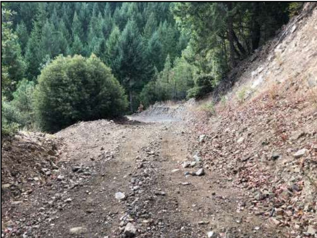
Photo #254 Private Access Rd @ Curve w/ Pullout Looking NW
