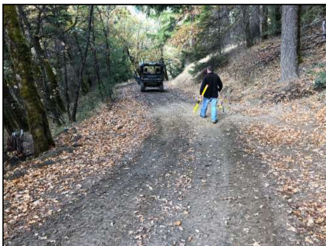
Photo #155 Private Access Rd @ Curve w/ Pullout Looking NW
