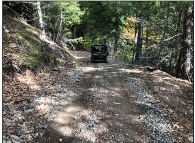
Photo #261 Private Access Rd @ Curve w/ Pullout Looking NE
