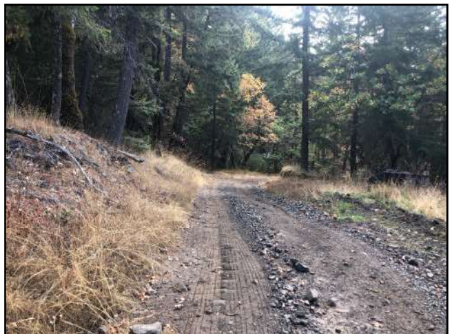
Photo #84 Private Access Rd @ Curve w/ Pullout Looking NW
