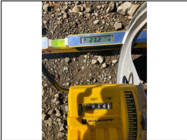
Photo #218 Private Access Rd Slope 23.2% Width 12'8"
