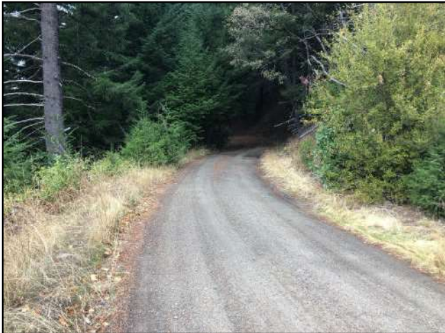
Photo #278 Private Access Rd @ Curve w/ Pullout Looking NW
