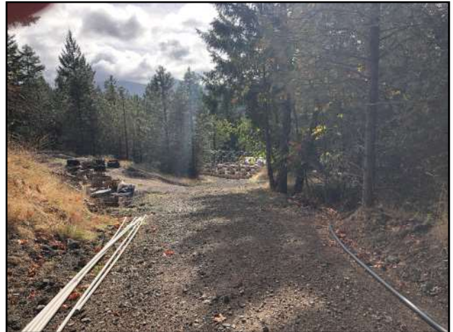
Photo #178 Private Access Rd @ Pullout Looking SE @ Cultivation Area
