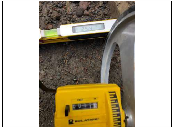
Photo #259 Private Access Rd Slope 25.4% Width 11'1"
