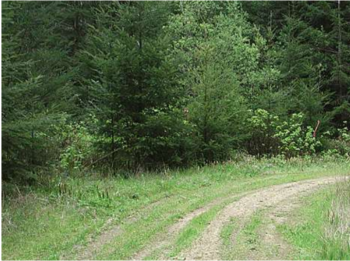
Figure 12. Grass cover on the surface of a road used for dry-season access. Source: Julie Bawcom, California Geological Survey.
