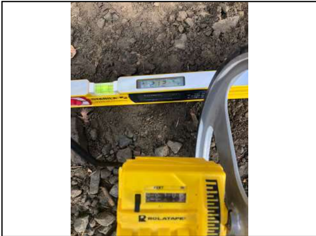
Photo #99 Driveway Slope 21.2% Width 10'9"
