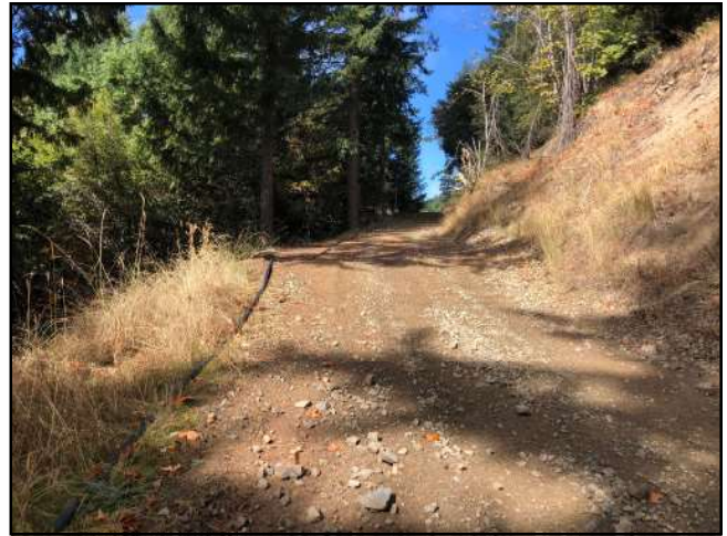
Photo #182 Private Access Rd @ Pullout Looking NW @ Curve
