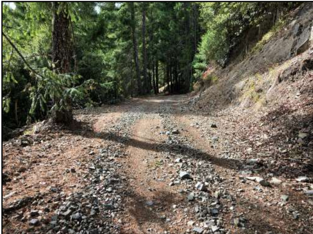
Photo #260 Private Access Rd @ Curve w/ Pullout Looking NW
