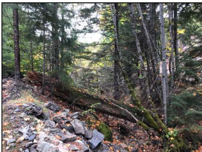
Photo #268 Private Access Rd Looking @ Hillside Slip w/ Falle Tree
