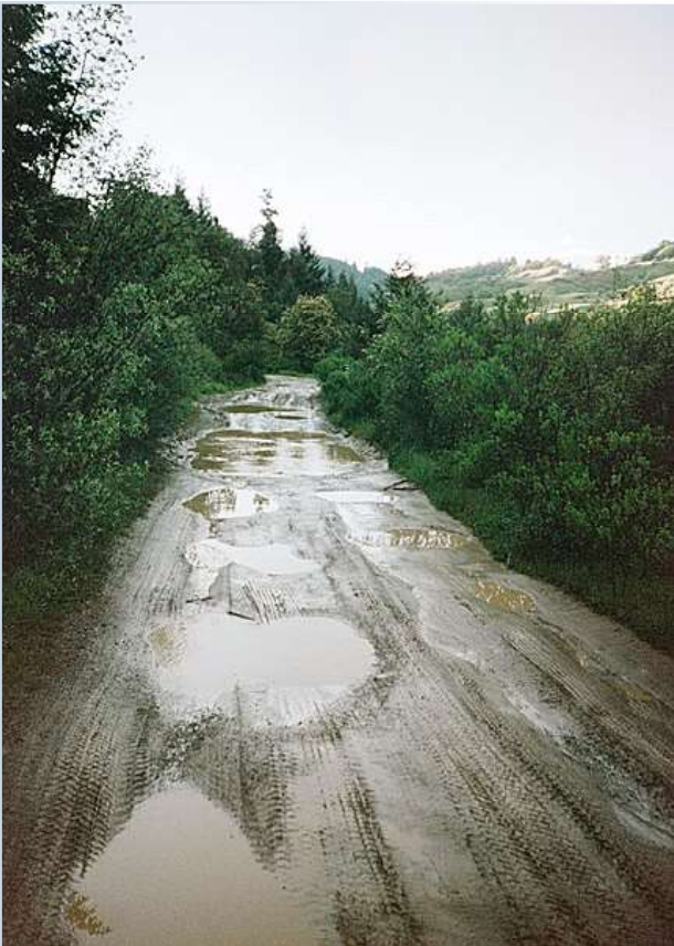
Figure 18. Water collecting on a forest road because of poor drainage. Photo: Jared Gerstein.
