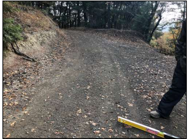
Photo #152 Private Access Rd @ Curve w/ Pullout Looking NW
