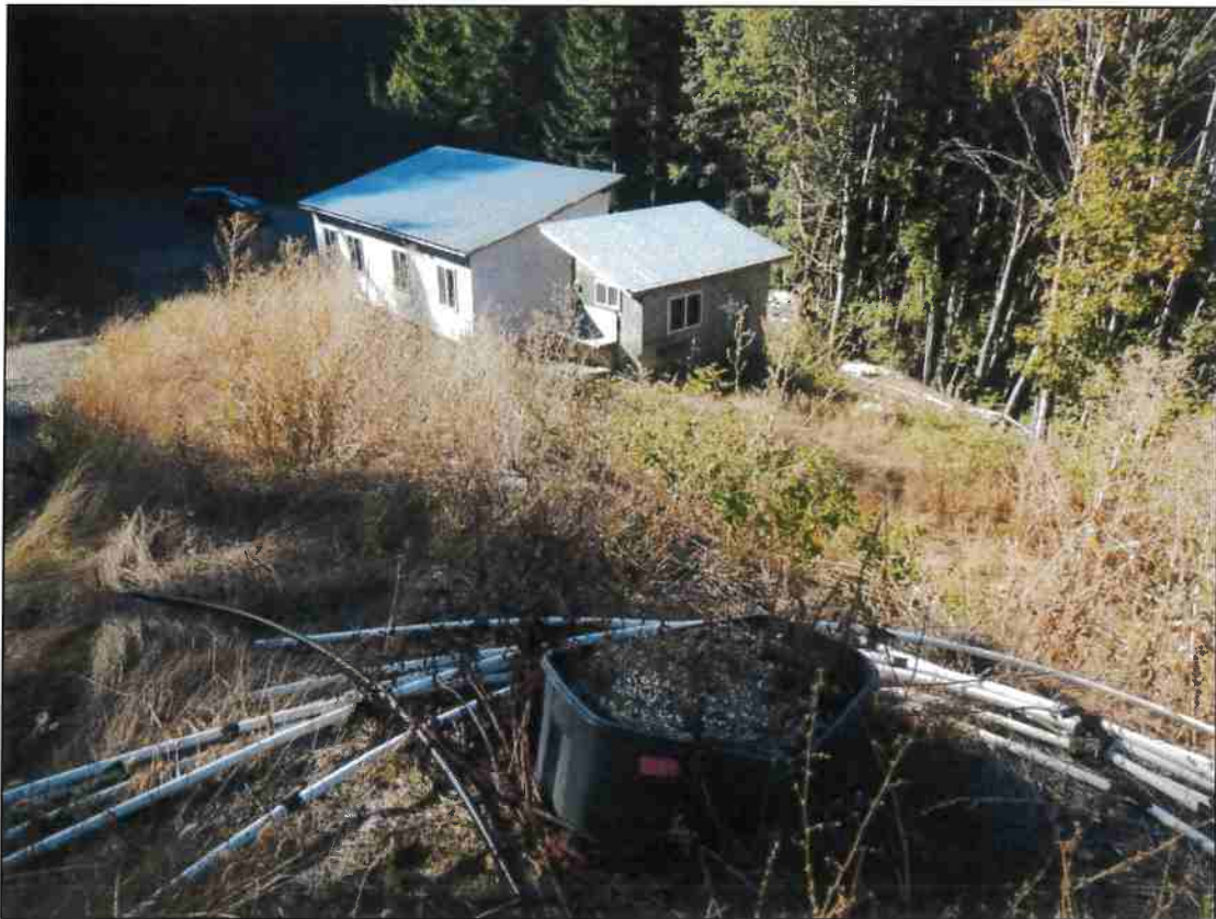
Photo 2. The other two (2) unpermitted structures within the Project Site to be removed. Referred to as "Processing Building" and "Storage Shed" in Appendix B: Map 1.
