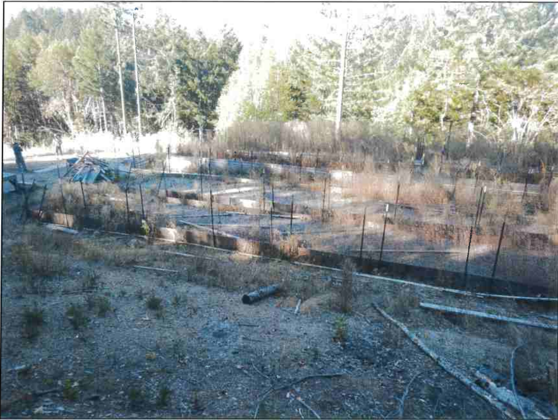
Photo 3. A portion of the constructed raised beds within the Project Site.
