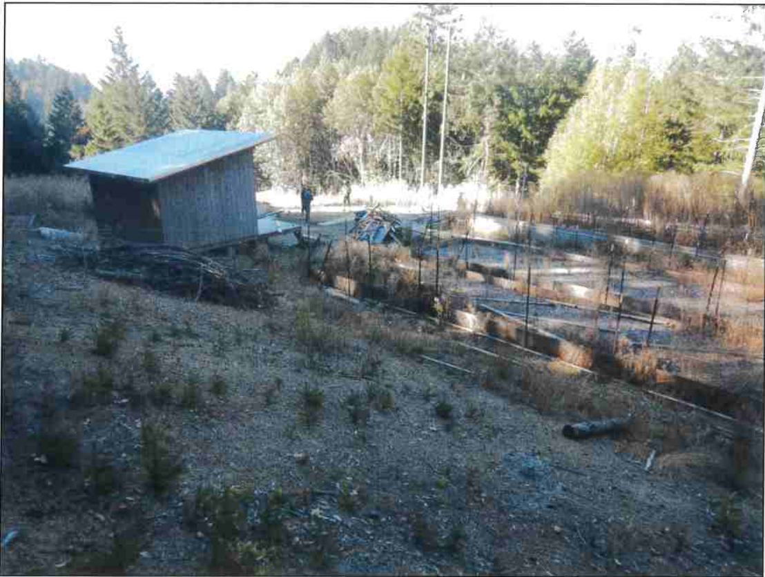
Photo 1. The small unpermitted structure upslope from the other two (2) structures within the Project Site to be removed.
