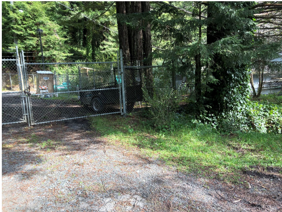
Photo 8: Terminus at City of Trinidad WTP (Approximate location of new flushing hydrant, internal pump pipe riser, and electric panel).
