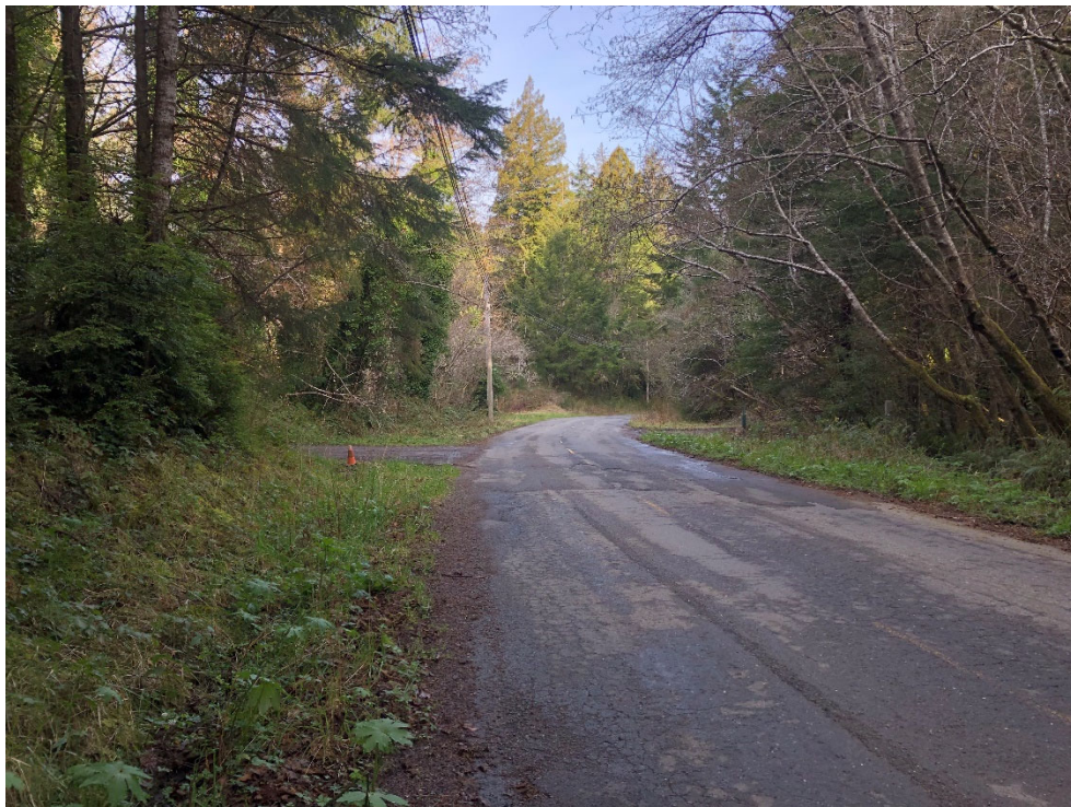
Photo 4: Shoulder Ditch (approximately 400 linear feet of seasonal wetlands).
