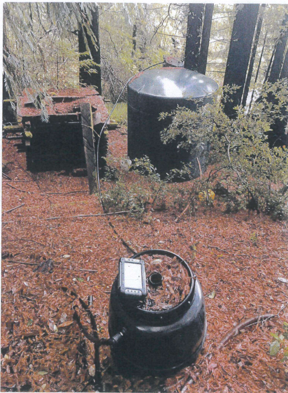
Picture 4: Pickle barrel (sediment trap) and 3,000 gallon hard plastic storage tank, which serves the house. Photo Date 10-17-16.
