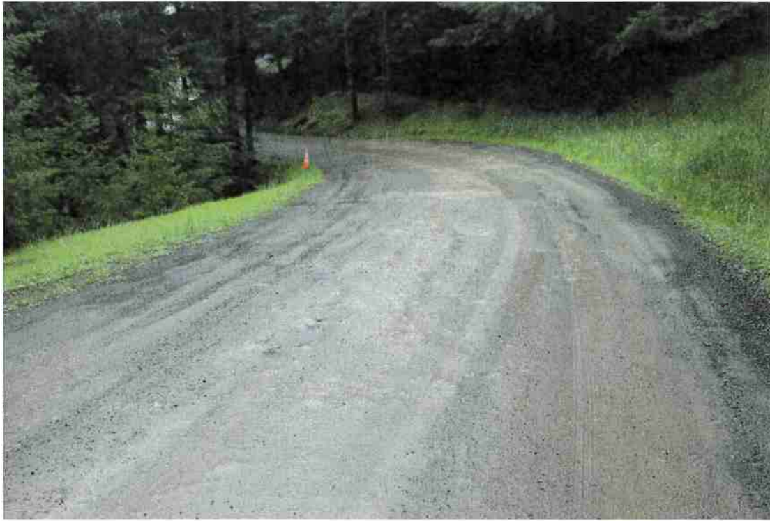
Photo 5. Mile 5.6: 20-ft road width with 2-ft shoulder.
