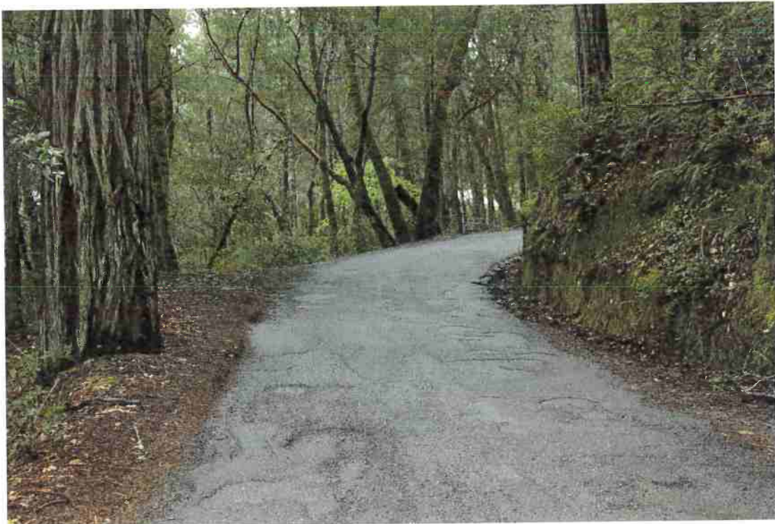
Photo 3. Mile 0.3: Pinch Point 2 with tree; 15-ft pavement width and 1-ft shoulders.
