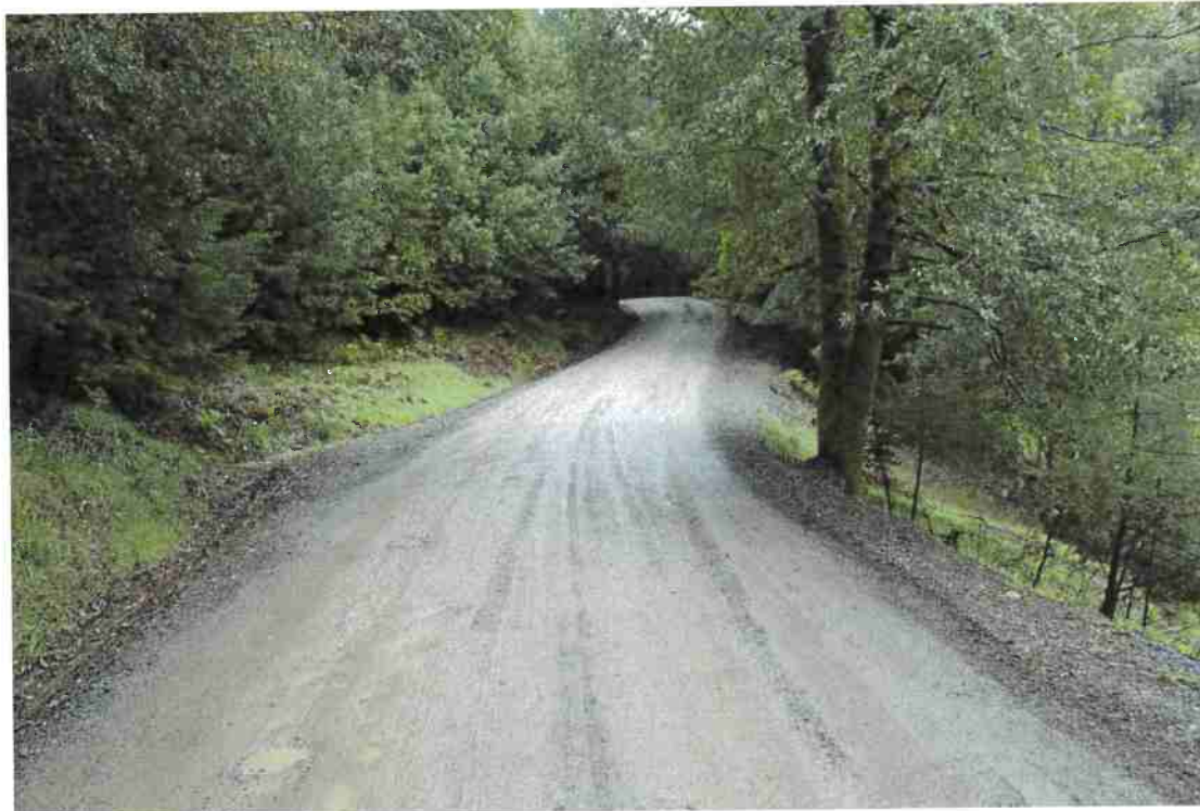
Photo 12. Mile 3.7: Typical 20-ft-wide road segment.
