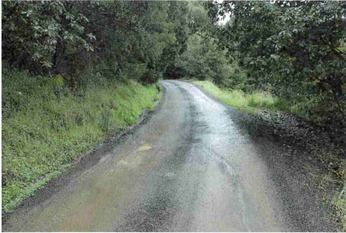
Photo 11. Mile 6.5: 12-ft road width with 1-ft shoulder.
