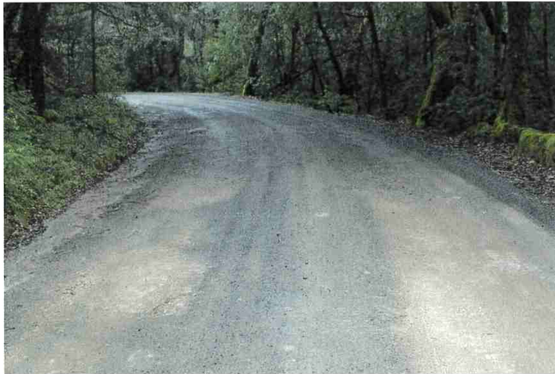
Photo 4. Mile 6.1: 18-ft road width with 1-ft shoulders.
