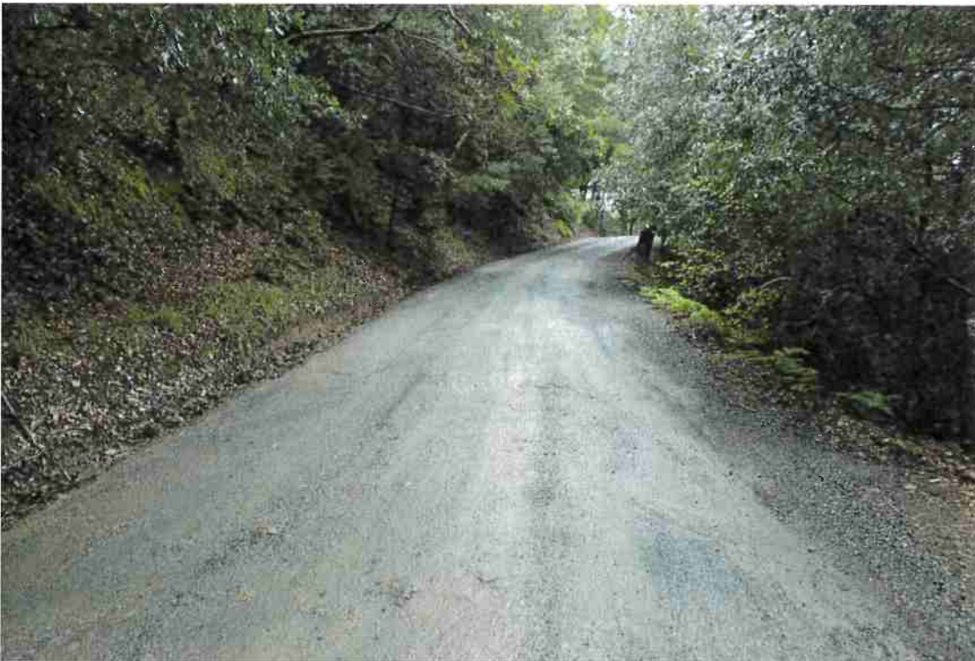
Photo 2. Mile 5.3: 18-ft road width with 2-ft shoulders.
