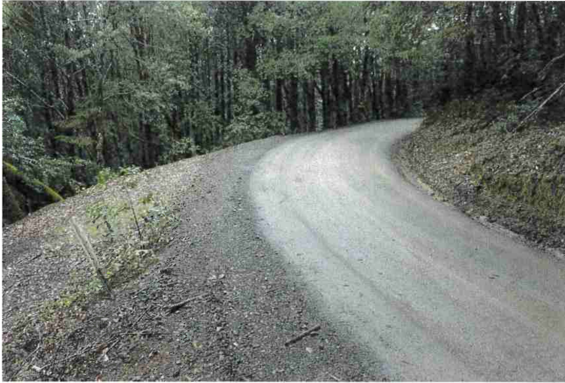
Photo 13. Mile 5.2: Typical 16-ft-wide road segment with blind corner—end of County-maintained road.
