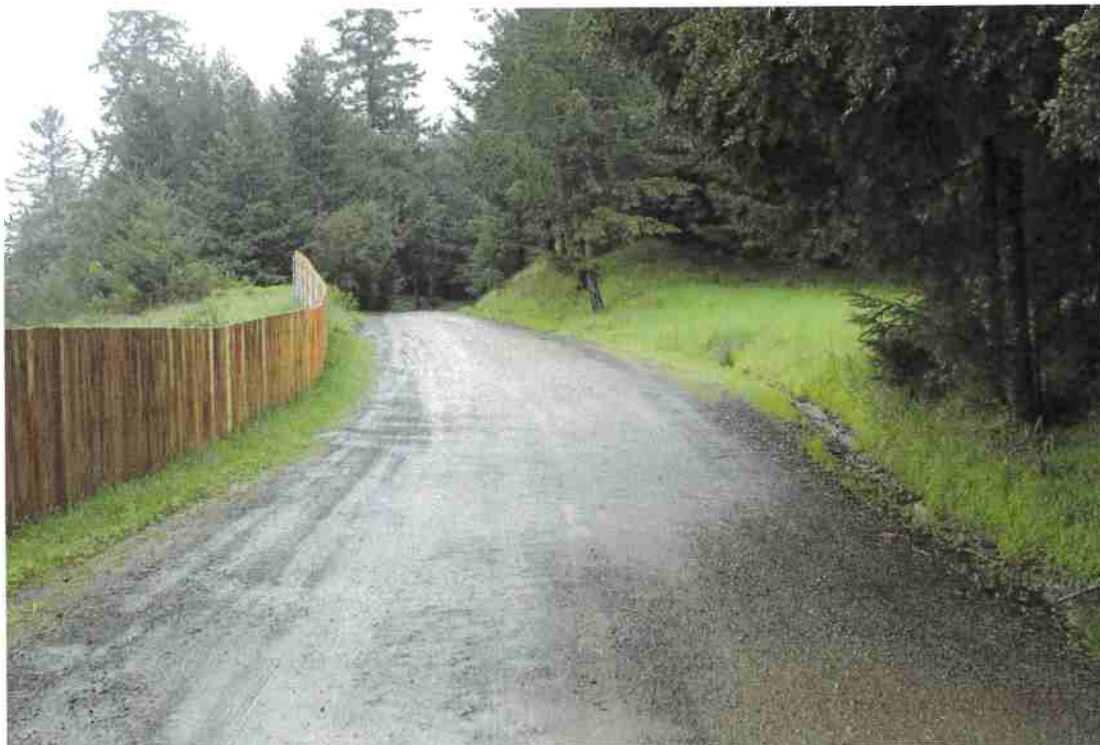
Photo 4. Mile 5.5: 20-ft road width with 2-ft shoulder.
