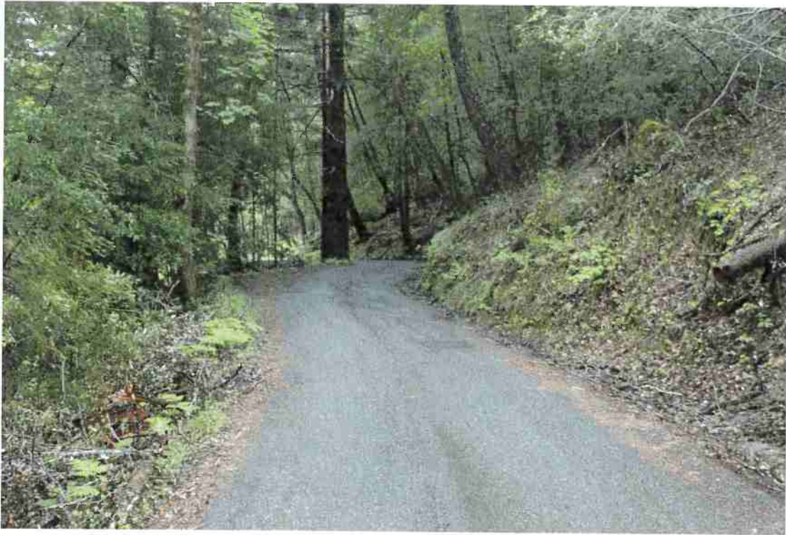
Photo 1. Mile 0.15: Pinch Point 1 with tree; 12-ft pavement width and 1-ft shoulders.
