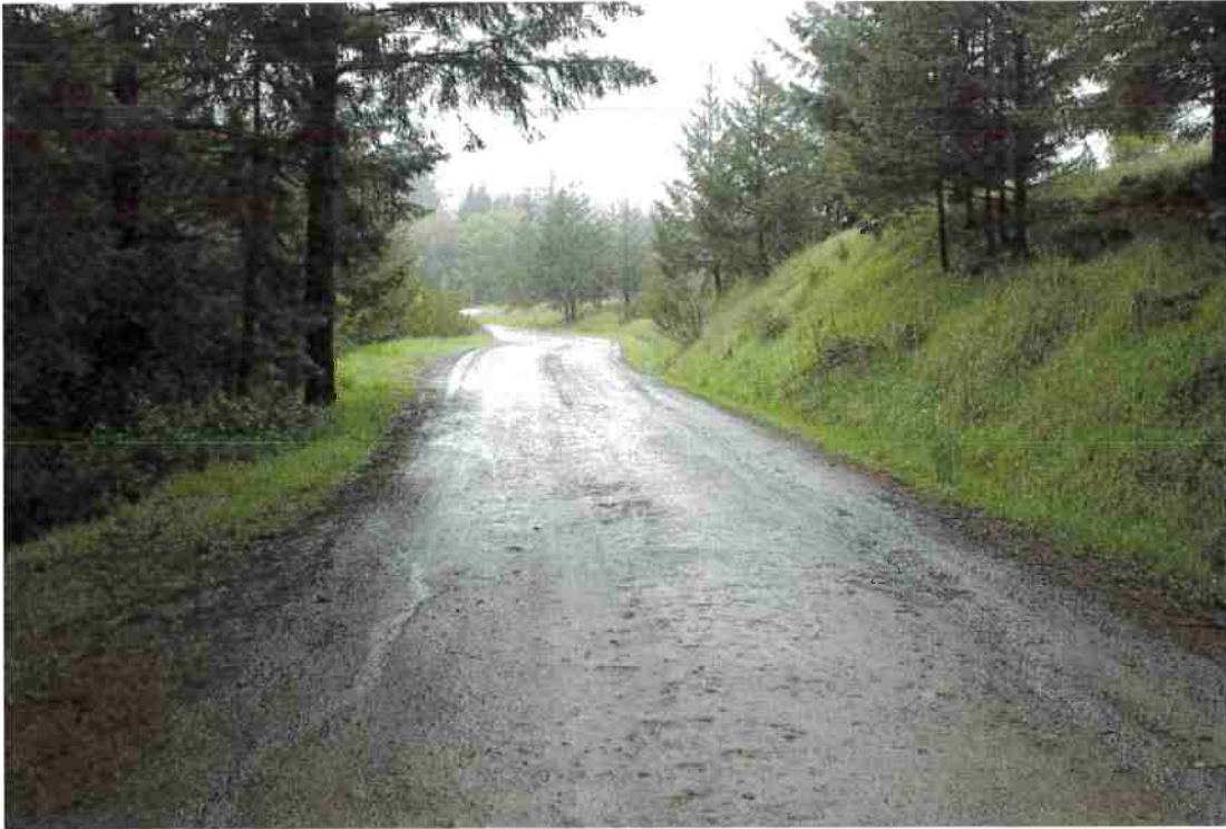
Photo 7. Mile 5.7: 20-ft road width with 2-ft shoulder.
