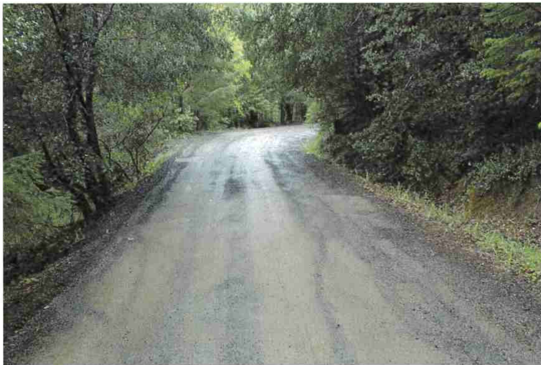
Photo 10. Mile 6.4: 16-ft road width with 1-ft shoulder.
