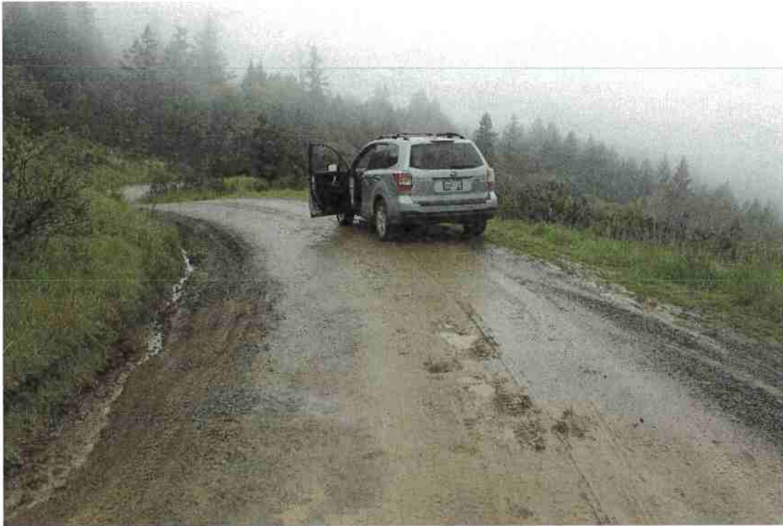
Photo 1. Mile 5.8: 16-ft road width with 1-ft shoulder (begin of segment).
