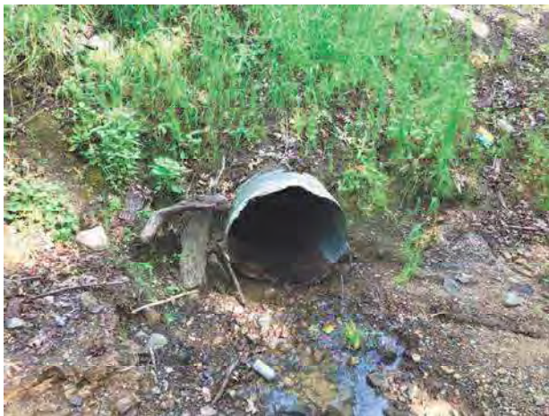
Photo #275, location 69 west end of 30" cmp outlet.
