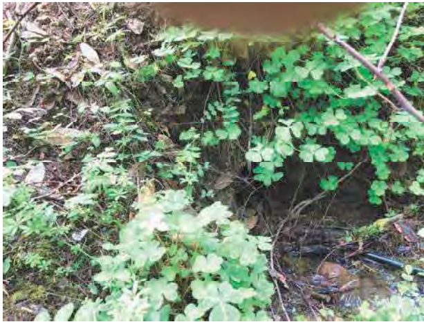
Photo #209, location 51 south side road 18" cmp outlet.
