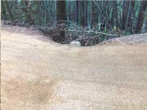
Photo #204, location 50 north side of road 18" cmp outlet.
