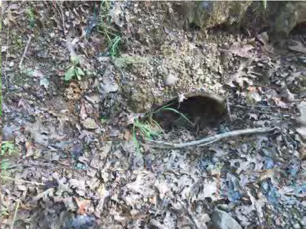
Photo #276, location 69 east end of 30" cmp inlet.
