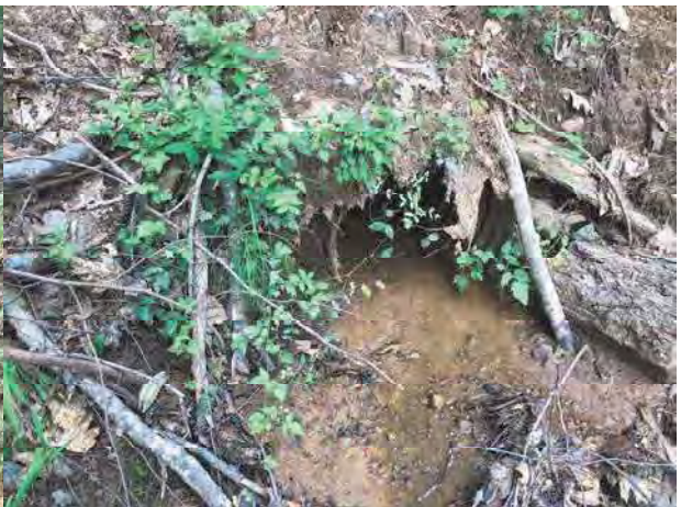
Photo #224, location 55 north side of road 18" cmp outlet.
