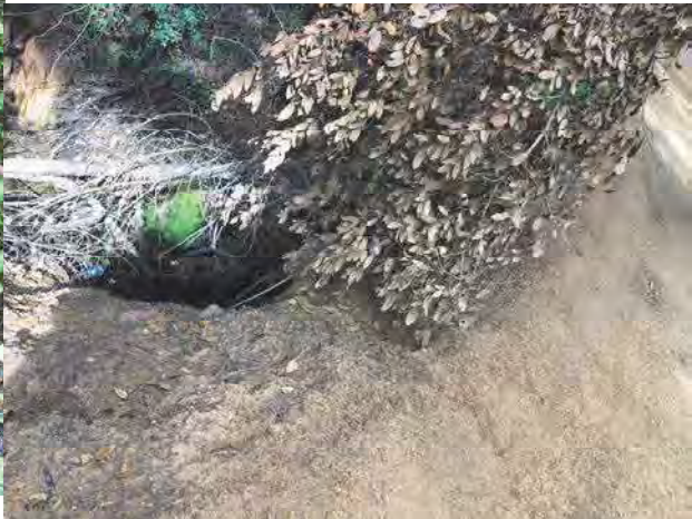
Photo #210, location 51 north side road 18" cmp inlet.
