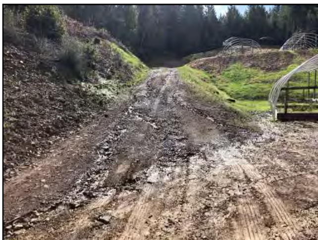
Photo #23 Private Driveway @ Cultivation Area On APN 216-381-021 Looking SE
