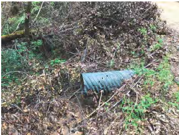
Photo #196, location 49 south end 18" cmp outlet.
