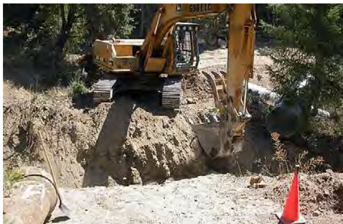
Figure 32. Excavator removing a crossing, including culvert and fill. Photo: Jared Gerstein.
