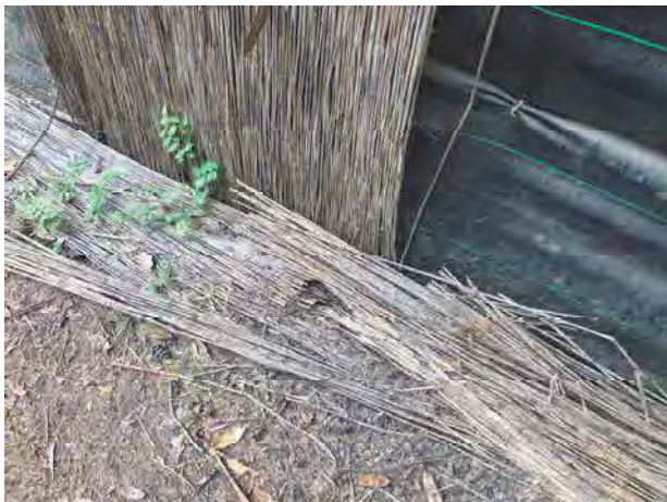
Photo #186, location 45 north west side of road near 18" cmp outlet.
