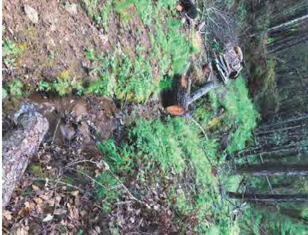
Photo #225, location 55 north side of road 18” cmp outlet.
