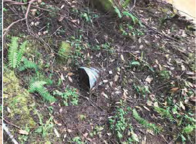
Photo #195, location 49 in north end 18" cmp inlet.
