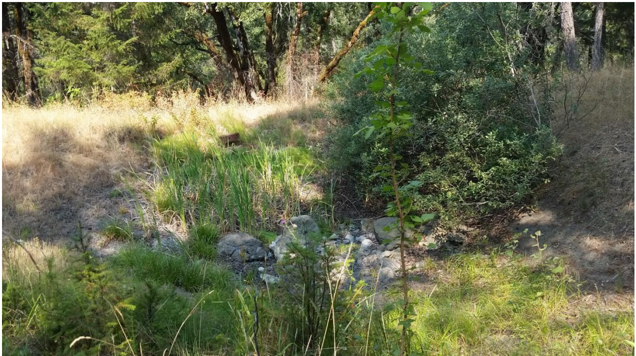
Picture 9. View of pond depression and overflow pipe/grate (dark square upper center left) near top of berm
