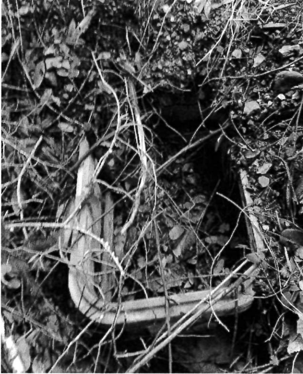
Ditch Relief Culvert 2: Plugged trash rack on a 12" diameter inside ditch relief culvert inlet. Remove debris from the trash rack and the culvert inlet rock armor the inlet and outlet per attached specifications. If the Discharger cannot remove the debris from the trash rack, the inlet, or the culvert is plugged, the Discharger shall replace the 12" diameter DRC with an 18" diameter ditch relief culvert per attached specifications.
