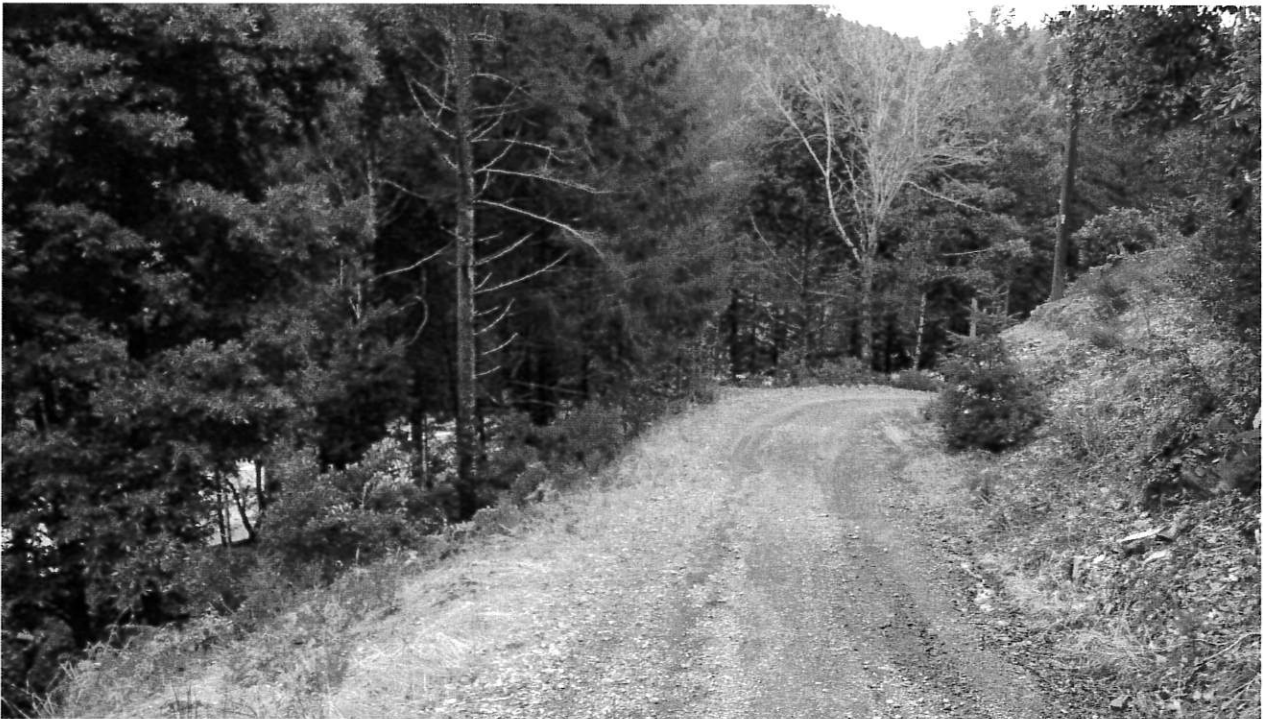
Road Point 1: Inside ditch flows are over-whelming the ditch relief culvert at DRC 1. Install a rolling dip per attached speciation's to reduce flows reaching DRC 1.
