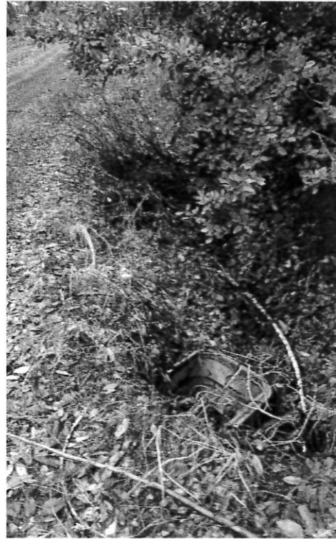
Ditch Relief Culvert 2: Plugged trash rack on a 12" diameter inside ditch relief culvert inlet. Remove debris from the trash rack and the culvert inlet rock armor the inlet and outlet per attached specifications. If the Discharger cannot remove the debris from the trash rack, the inlet, or the culvert is plugged, the Discharger shall replace the 12" diameter DRC with an 18" diameter ditch relief culvert per attached specifications.
