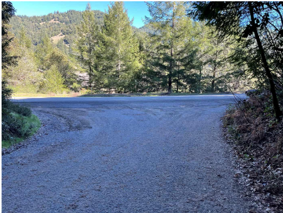
Figure 4: RP 1. Intersection of Highway 101 and Milky Way Loop, Paved apron 36' in width. Image taken at facing east.
