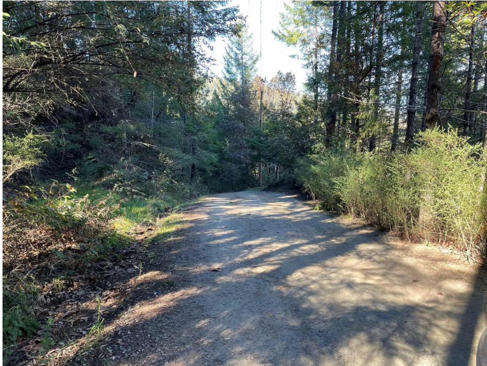
Figure 14: RP 6. Milky Way Loop – 14-16' dirt/gravel road width. shown facing north; towards Highway 101.
