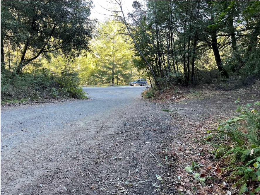
Figure 6: RP2: Milky Way Loop - 16' paved road width; location of 10' turnout. Image shown facing east; towards Highway 101.
