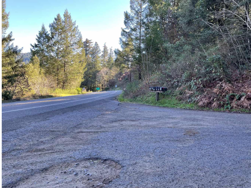
Figure 3: RP 1. Intersection of Highway 101 and Milky Way Loop, Paved apron 36' in width. Image taken facing south.
