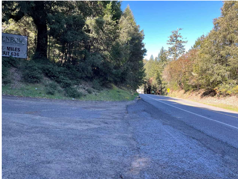
Figure 2: RP 1. Intersection of Highway 101 and Milky Way Loop, Paved apron 36' in width. Image taken at facing north.
