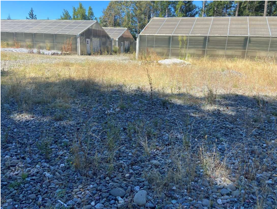
Photo 4 – Heavy rock layer over post-2015 conversion area.
