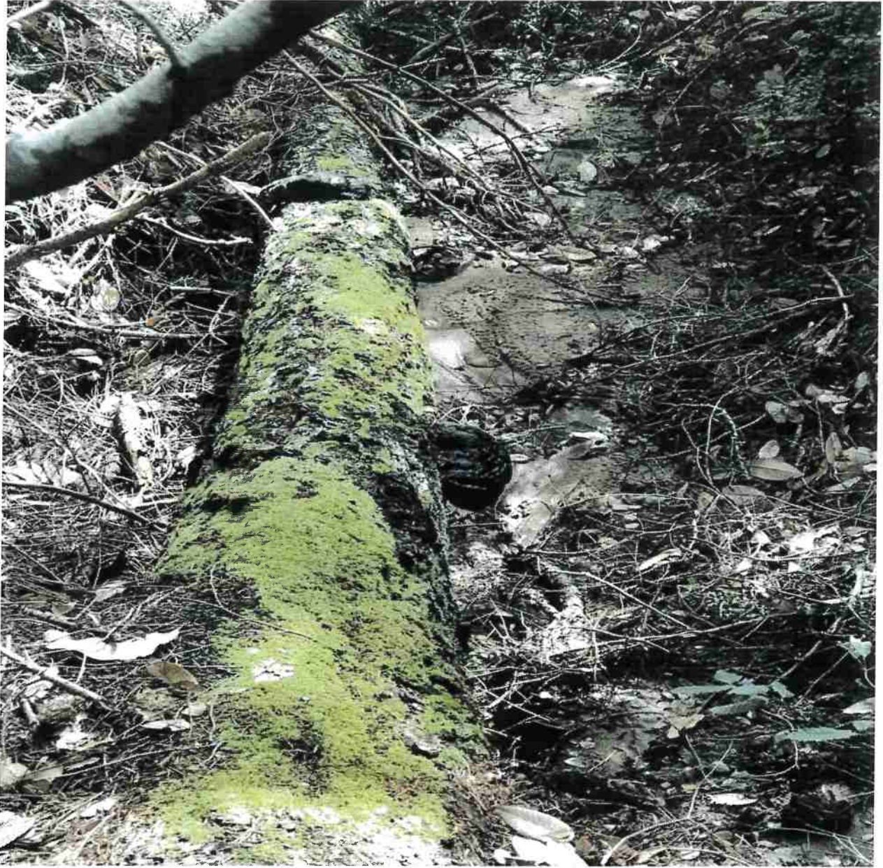
Ditch obstructed with sediment and debris
