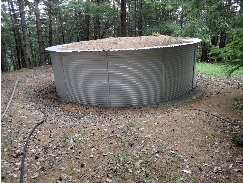
Photo 19 - The 25,000 gallon water tank constructed on an engineered graded pad (pers. comm. Landowner, 2017).
