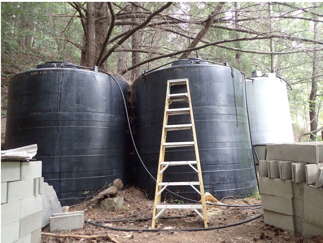
Photo 16 - View of the three water tanks that are within the 50 foot riparian buffer of the spring.
