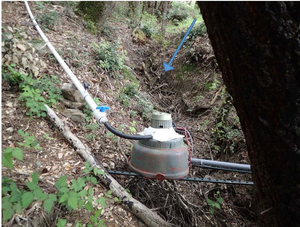
Photo 17 - View of the Pelton wheel above a Class II watercourse; note the arrow pointing at the watercourse.
