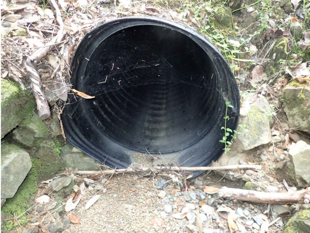
Photo 9 - SC #3; View of the inlet with rock armored fill.
