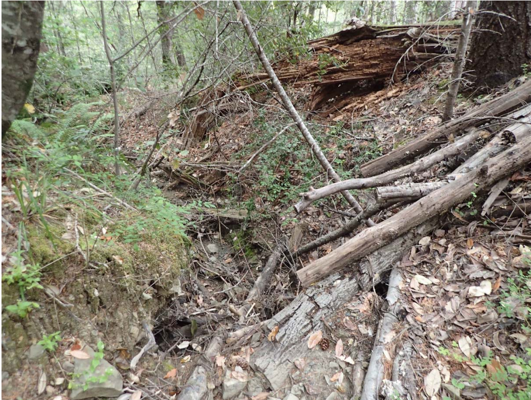
Photo 11 - SC #3; View looking downstream of the outlet
