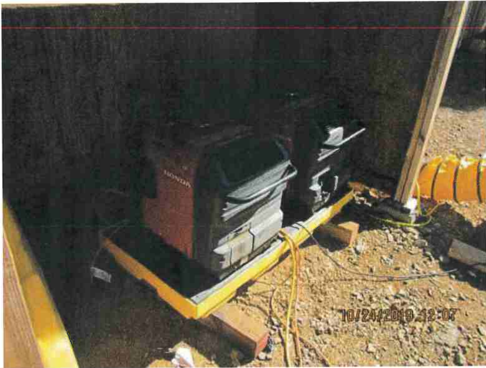
Photo 15. Generator in secondary containment
