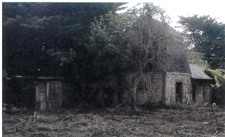
Figure 5.2 Barn, South Elevation
