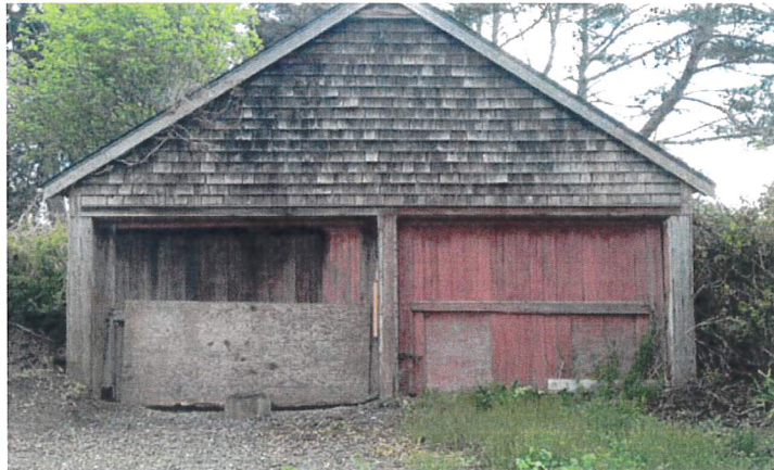
Figure 3.1 Garage, South Elevation
