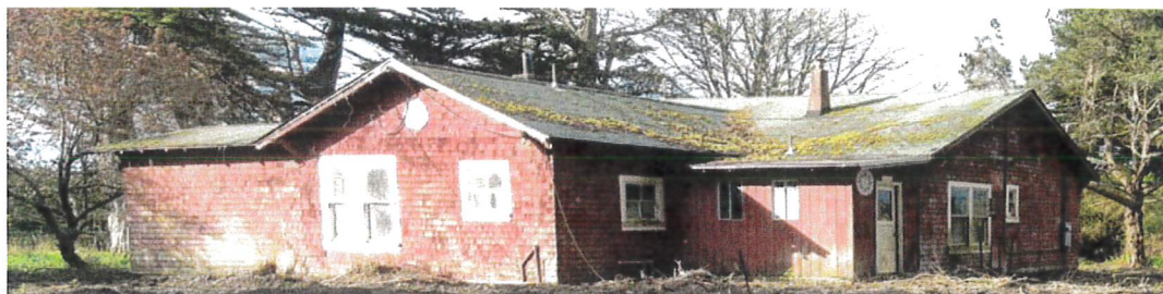
Figure 1.5 Single Family House, North Elevation
