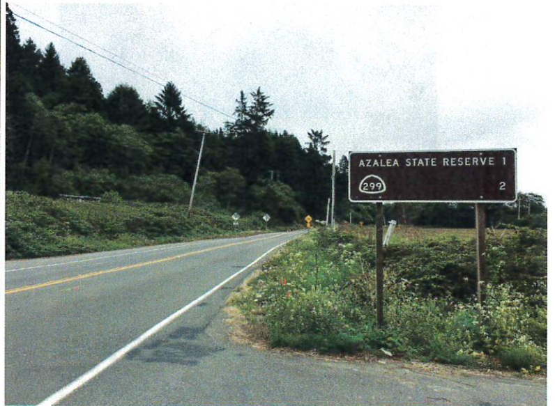
North Bank Road (Highway 200) heading east has no walking or bicycling facilities and very narrow shoulder.
