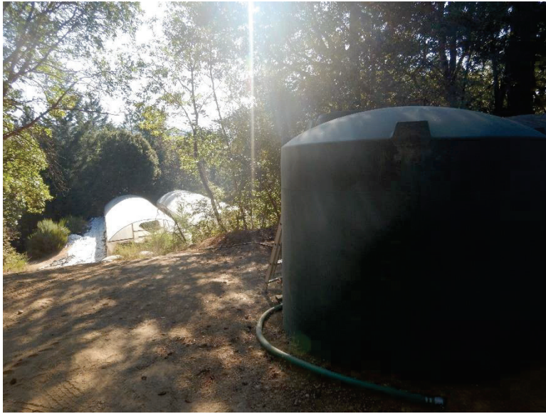
Photo 1 – Upper Cultivation Area: Water storage tank with hose attachment for water delivery truck. View of hoop houses in background
