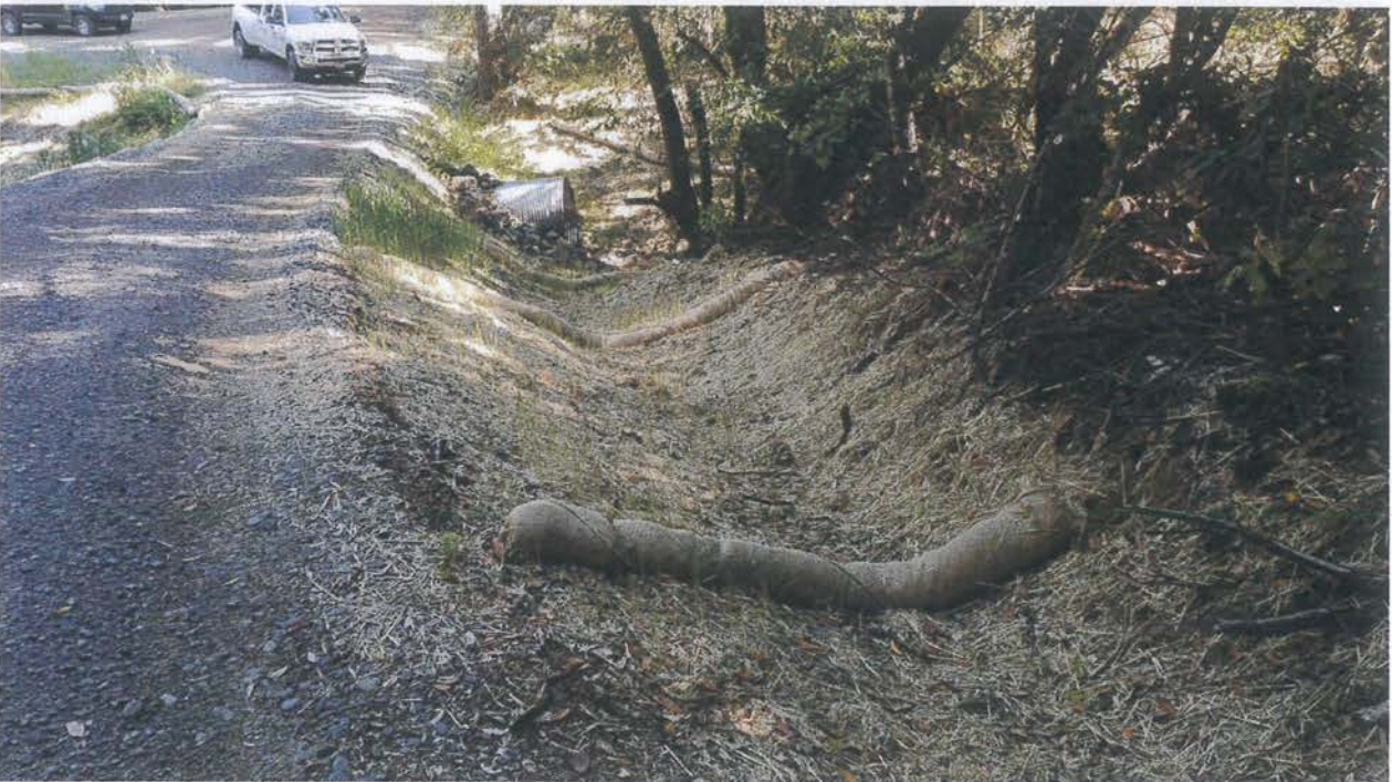
Photo looking down at the inlet of Site 09.
