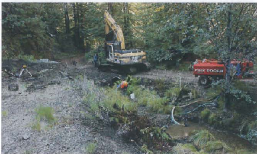
FIGURE 199. For larger streams, pump trucks, large pumps or multiple small pumps can be used to pump streamflow around project work sites. Here, a pump truck is used to temporarily divert flow in a fish bearing stream where dual culverts are being replaced with a railcar bridge. Young fish were removed from this fish bearing stream before project work started.
