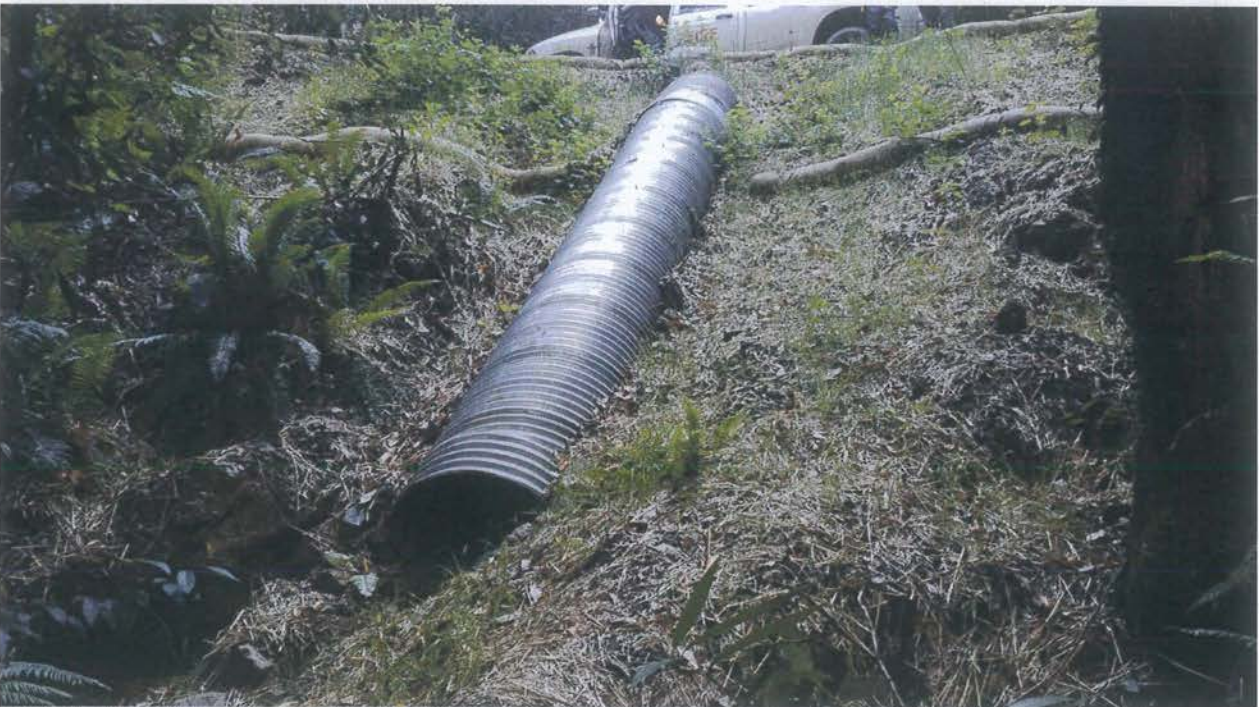
Photo looking at the downspout of Site 03.
