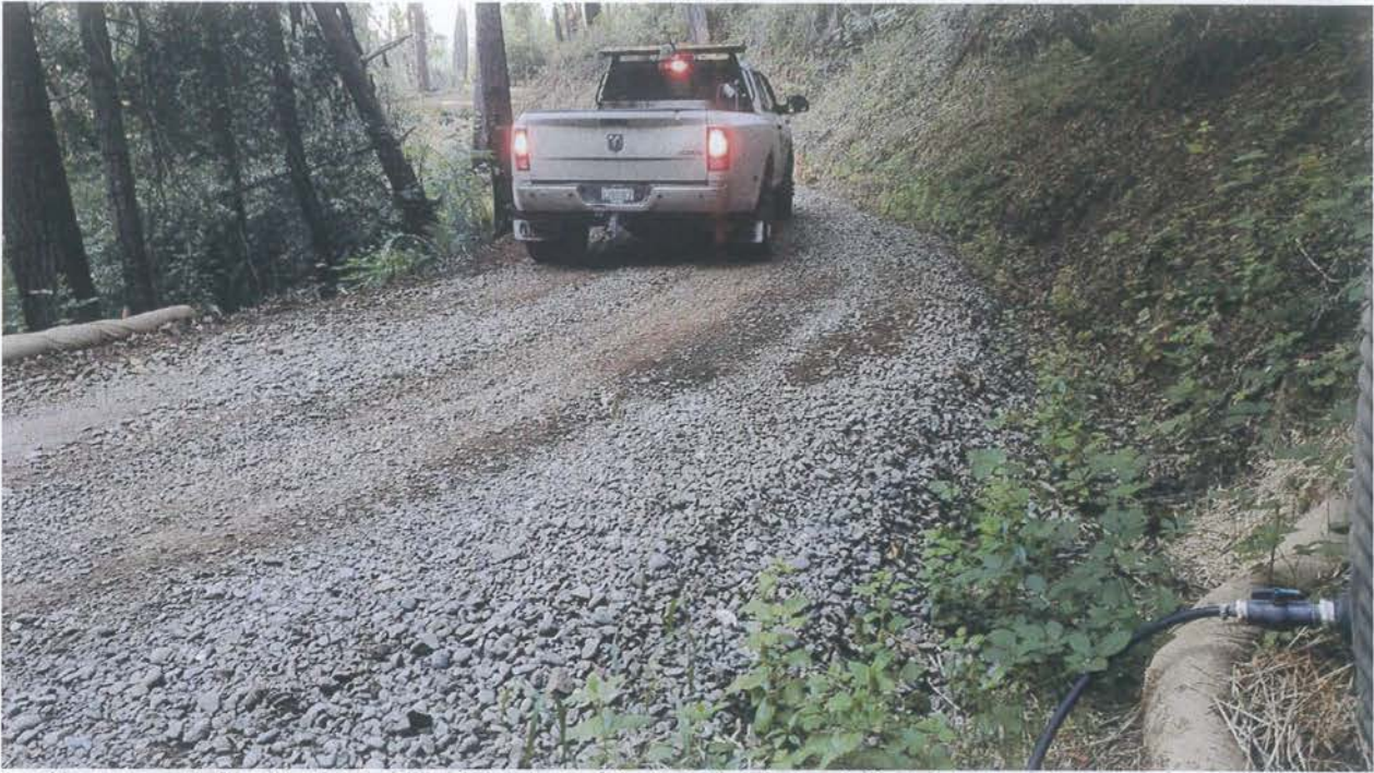
Looking up grade from the inlet of Site 03 at the inside ditch that drains to the inlet.
