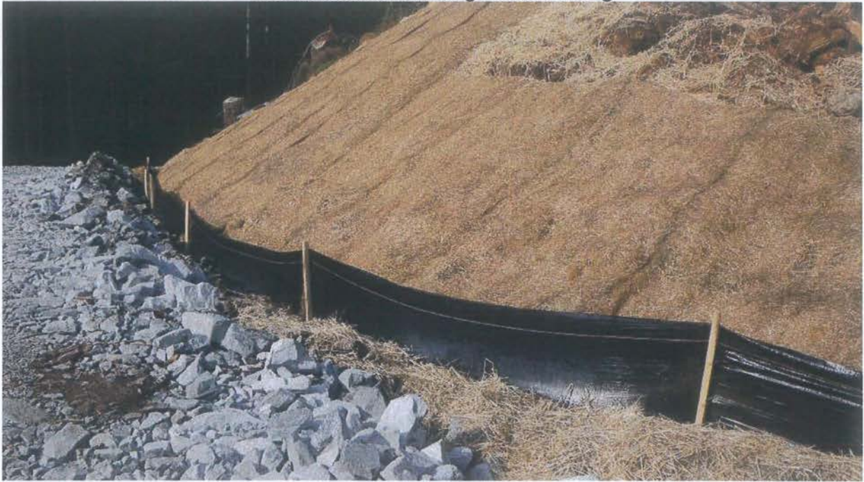
Erosion Control Matting & Silt Fencing
