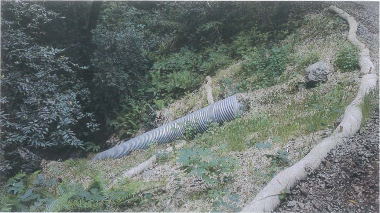
Photo looking at the downspout of Site 03.
