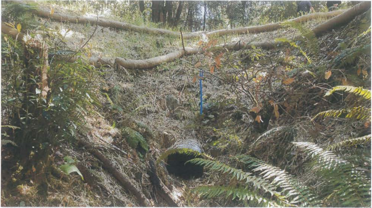
Photo of the outlet of Site 13.
