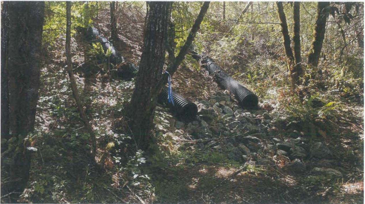
Photo looking at the outlet of Site 10.
