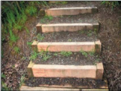
Example of a cribbed staircase
