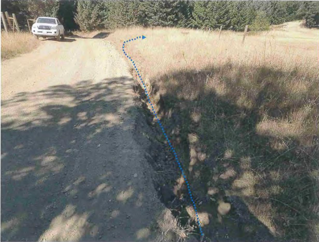
**Picture 7:** A spring pool overflows is intercepted by the road's inside ditch for 300-feet. The water is eroding the inside ditch and the Applicant shall install a DRC. Photo date 11-07-2017.
