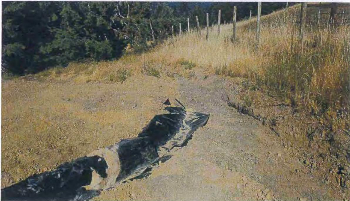
**Picture 15 + 16:** MP #3 consists of a lined spillway leading from a rain catchment pond with no rock armor or other form of energy dissipation. The Discharger shall install adequate rock armor at this location to prevent erosion from occurring. Photo date: 07/14/2016
