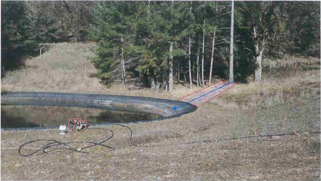
**Picture 23:** The Class III watercourse is currently bypassing the pond which is proposed to have a rocky spillway inlet constructed to facilitate larger flows through the pond. Photo date 11-07-2017.
