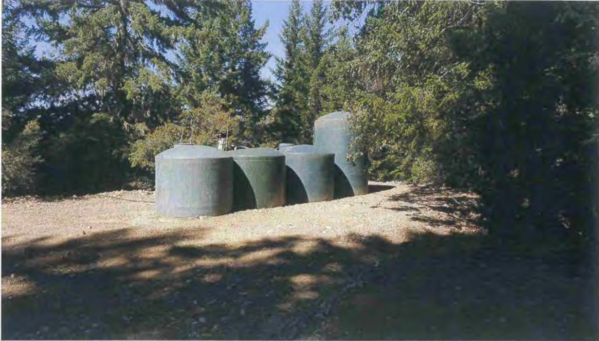
**Picture 13:** Three 3,000-gallon and one 5,000-gallon hard plastic water storage tank. Photo date 11-07-2017.
