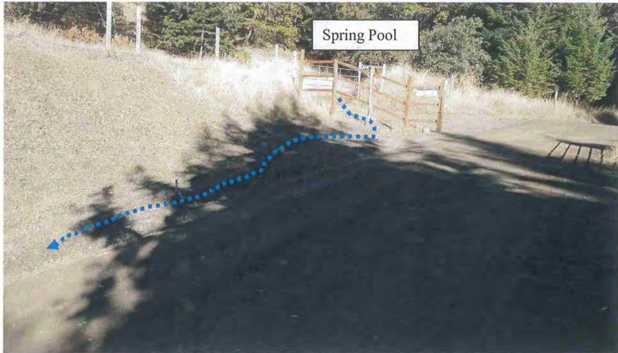
**Picture 6:** A spring pool overflows is intercepted by the road's inside ditch. Photo date 11-07-2017.
