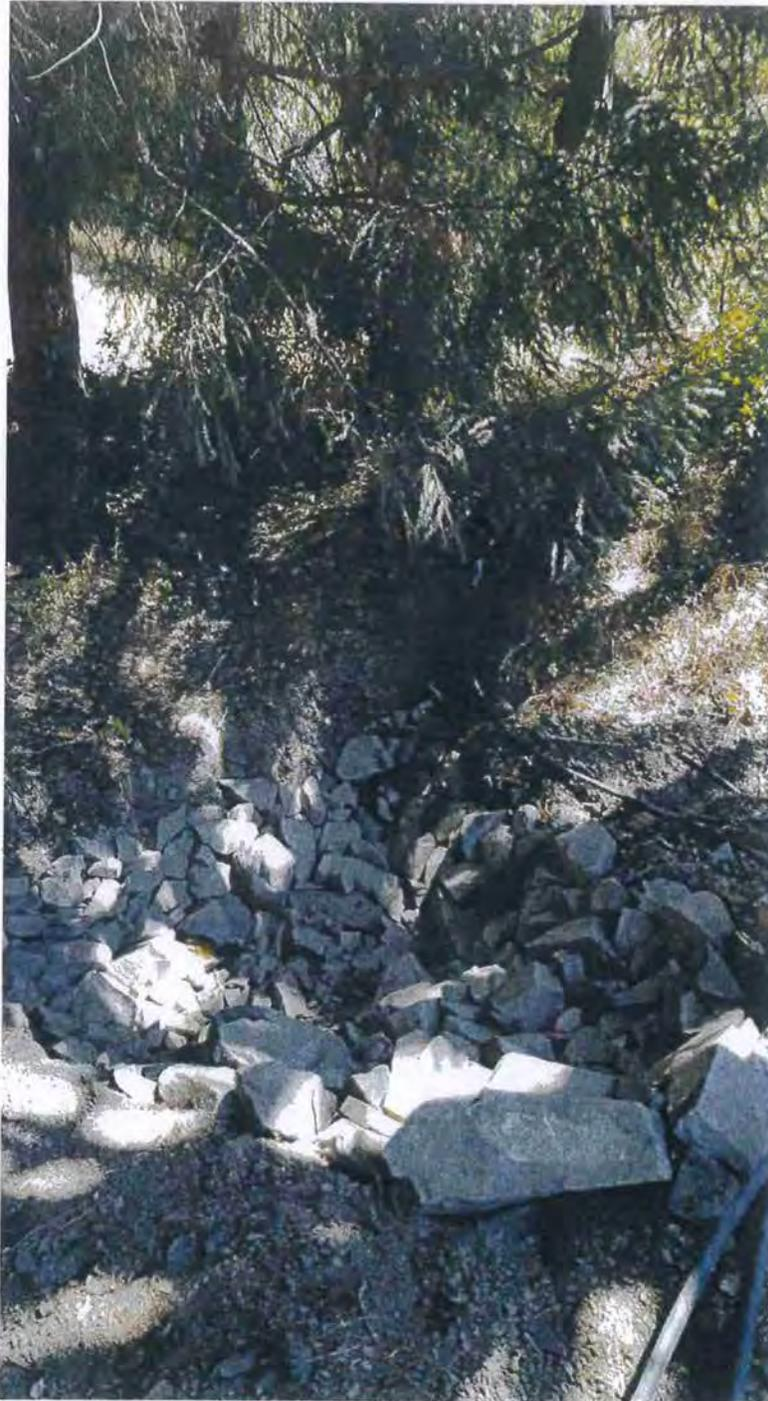
**Picture 17:** SC #1 is a 10" diameter CPP located on an unnamed Class II watercourse. This crossing shall be upgraded to a minimum 42" diameter culvert per attached specifications. Also seen in this picture is the catchment structure for the watercourse bypass. The pond shall be removed and the watercourse shall be restored per Standard Conditions A(3)c. Photo date: 07/14/2016
