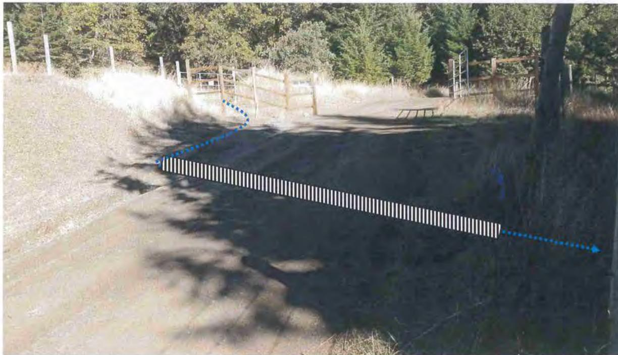
**Picture 8:** A spring pool overflows is intercepted by the road's inside ditch. The Applicant shall install a ditch relief culvert to convey the spring water into the swale feature. Photo date 11-07-2017.
