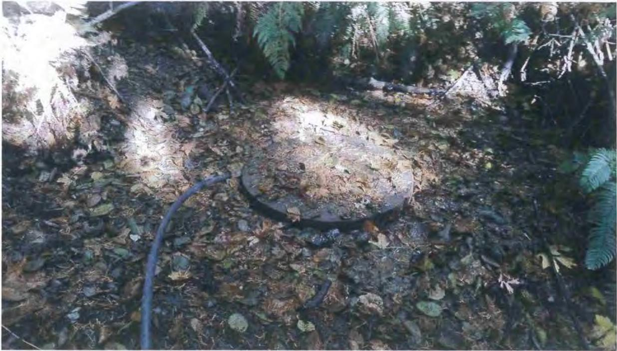
**Picture 31:** The Point of diversion is a concrete cistern in Class II Spring at the head of a watercourse. Photo date 11-07-2017.
