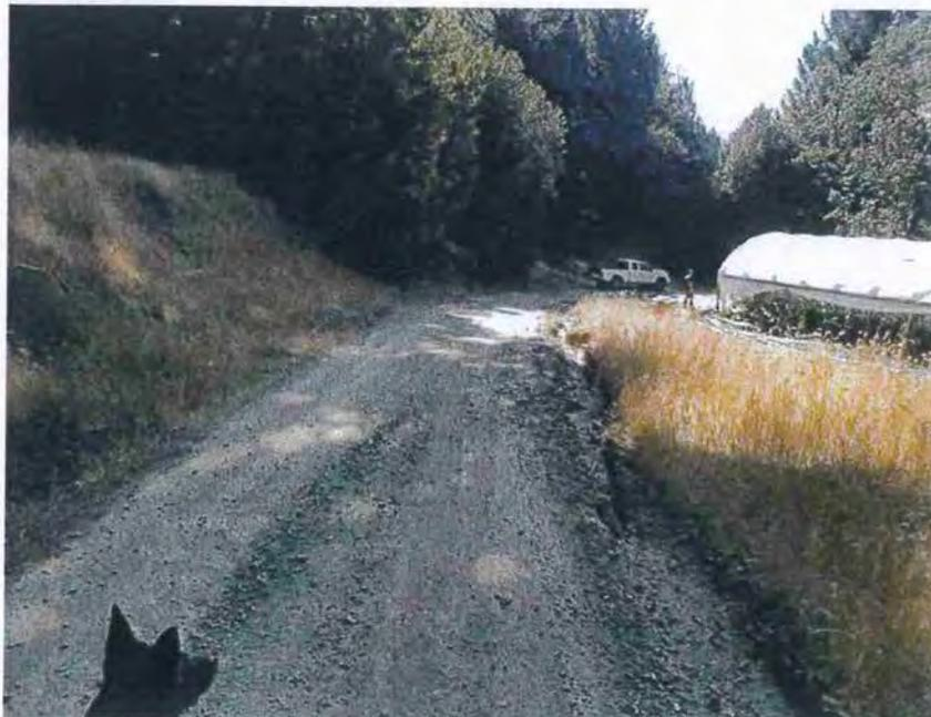
**Picture 14:** MP #2 is where storm runoff is concentrating along the outboard edge of the road and has eroded the road surface. The Discharger shall repair the drainage feature located behind the photographer in this picture. Photo date: 08/03/2017
