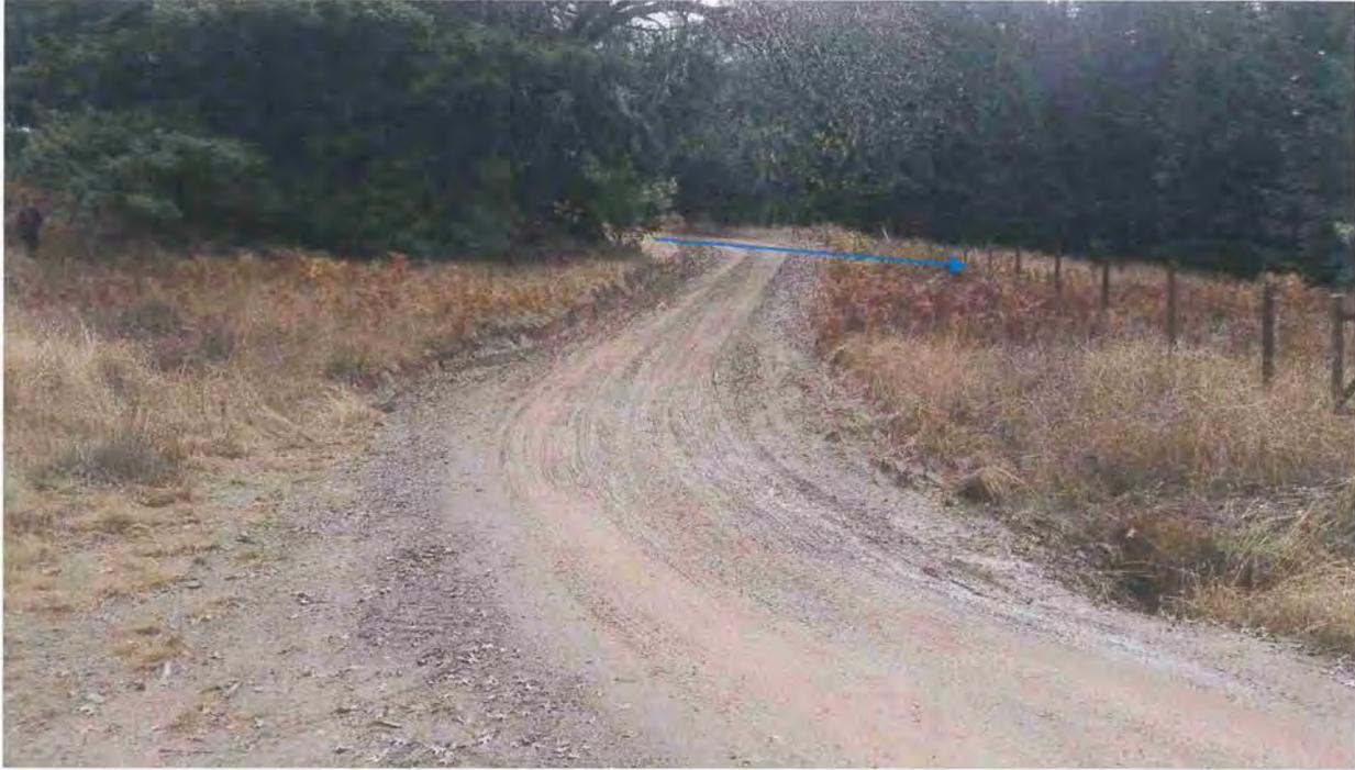
**Picture 10:** The inside ditch is drain 400-feet of road and is hydrologically connected to the Class III watercourse at the inlet of Crossing #1. The Applicant shall install a ditch relief culvert to disconnect the road surface runoff. The proposed location is mapped and flagged. Photo date 11-07-2017.
