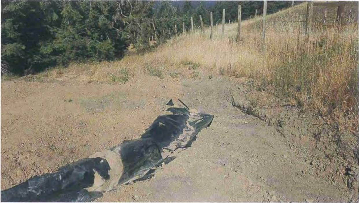
**Picture 48:** Rain Catchment Pond overflow spillway is not hydrologically connected and outlets into a vegetated swale 30-feet west. Photo date 07-14-2016.
