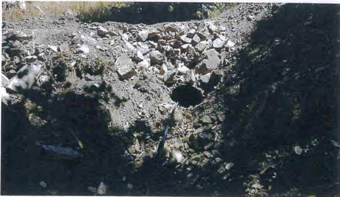
**Picture 19:** Outlet of SC #3. This crossing is a 24" diameter CPP located on an unnamed Class III watercourse. This culvert shall be upgraded to a minimum 42" diameter culvert per attached specifications. Photo date: 07/14/2016
