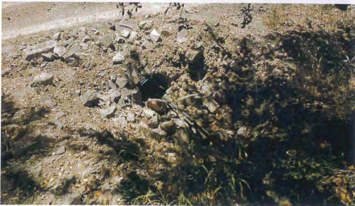
**Picture 20 + 21:** Inlet (top) and outlet (bottom) of SC #4. This crossing consists of a 24" diameter CPP located on an unnamed Class III watercourse. This culvert shall be upgraded to a minimum 42" diameter culvert per attached specifications. Photo date: 07/14/2016
