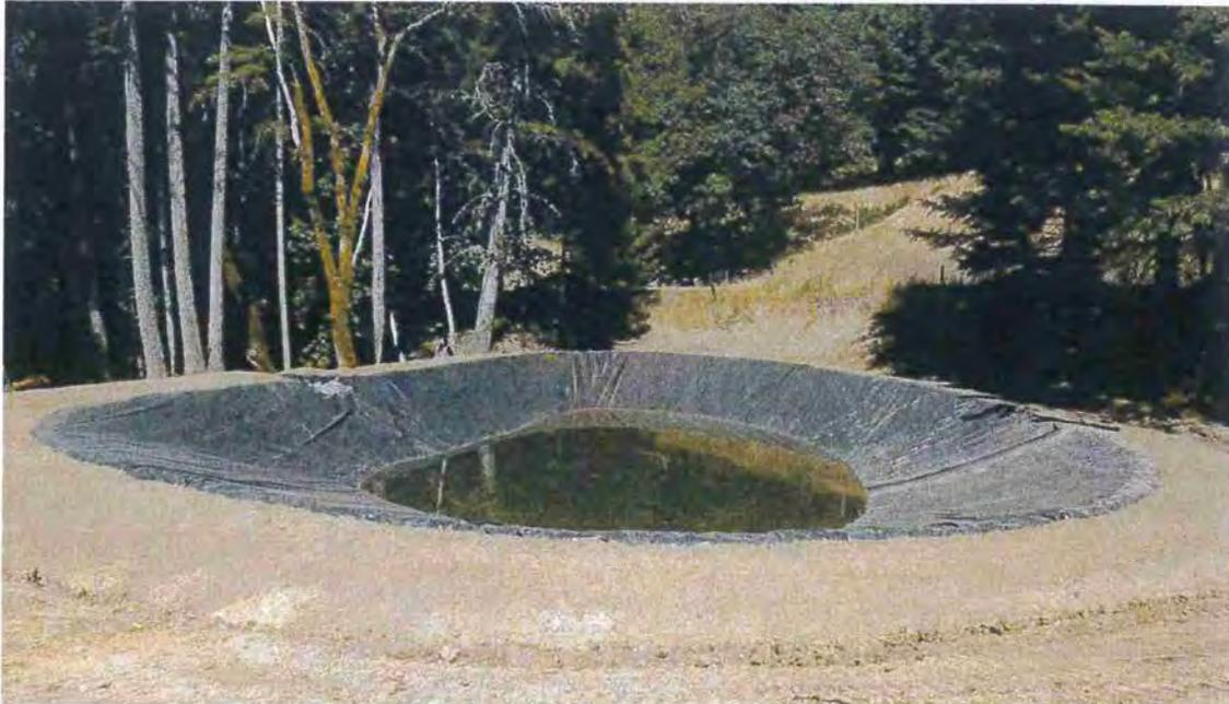
**Picture 23:** MP #2 consists of an 80' wide by 95' long by 10' deep rain catchment pond. This pond was constructed atop a Class II watercourse. The Discharger shall remove the pond liner, contour the site back to native conditions, and plant native riparian species to restore the riparian buffer per attached specifications. Photo date: 07/14/2016
