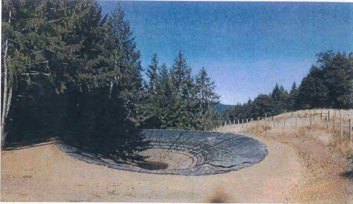
**Picture 11:** One source of agricultural water in the property is a 275,000 gallon rain catchment pond. The pond is 108' wide by 75' long by 15' deep with an average depth of 6'. Photo date: 07/14/2016
