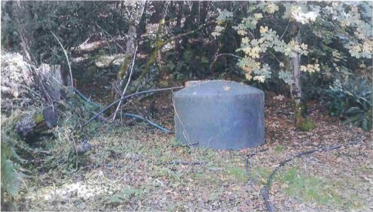
**Picture 34:** One 1,550-gallon hard plastic water storage tank plumbed to POD. Photo date 11-07-2017.
