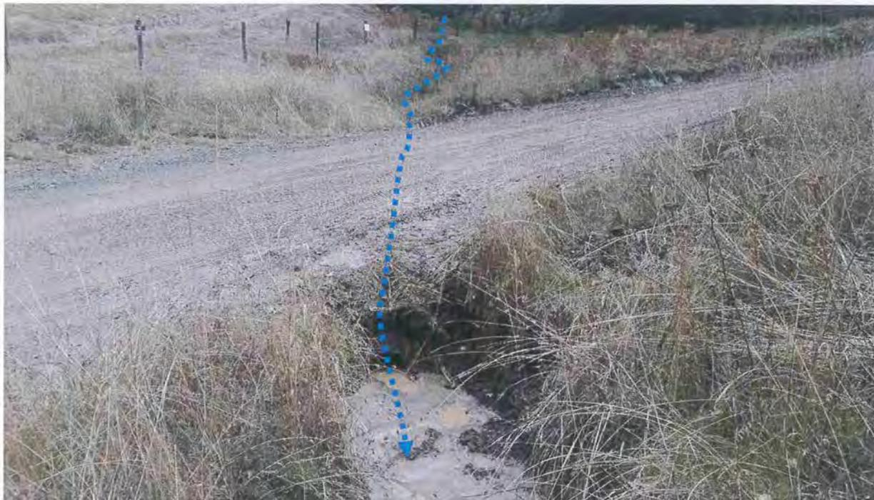
**Picture 11:** Looking upstream at the outlet of Crossing #1 on a Class III watercourse. The outlet is half buried in sediment due to the hydrologically connected inside ditch. Photo date 11-07-2017.
