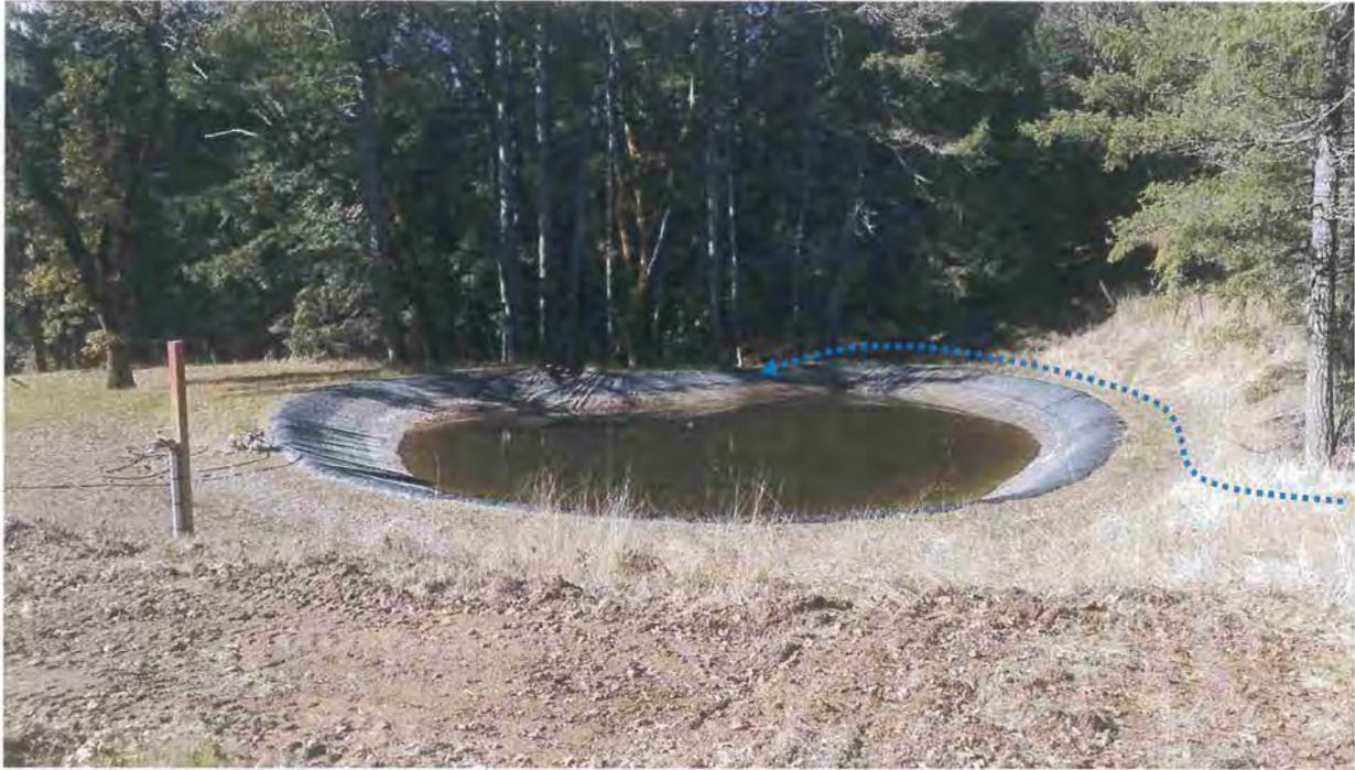
**Picture 20:** On-stream Pond located within the Class III watercourse. The pond has been constructed over the Class III watercourse. The watercourse is by passing around the northside via a 10-inch diameter flex pipe to bypass the pond. Photo date 11-07-2017.
