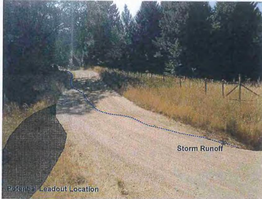
**Picture 13:** MP #1 is where storm runoff is concentrating along a road resulting in sediment delivery to a Class III watercourse. The Discharger shall install a drainage structure at this location. A lead out along the inboard edge of the road at this location is recommended. Photo date: 08/03/2017
