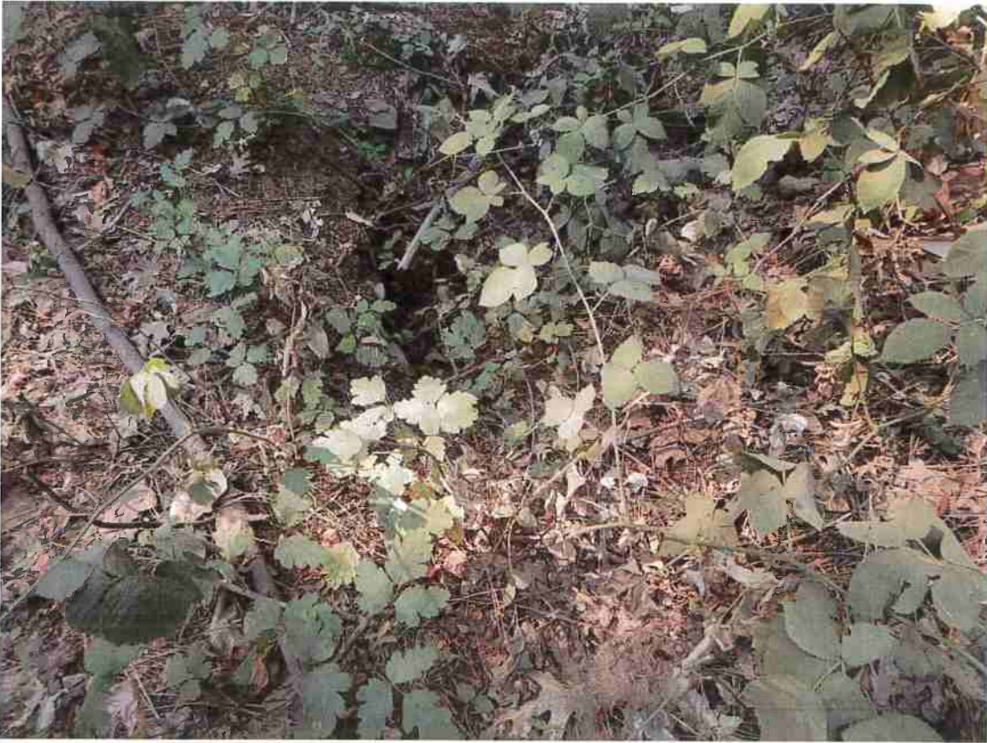
Photo 16: RP 8. Inlet to drainage relieve culvert.
