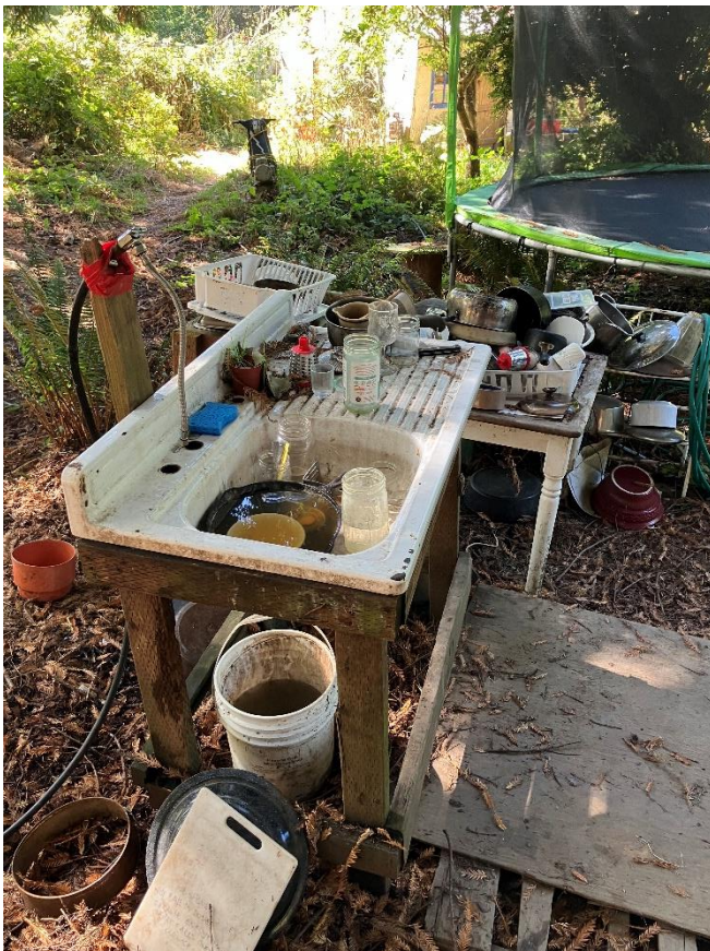
sink discharge to bucket near #93
