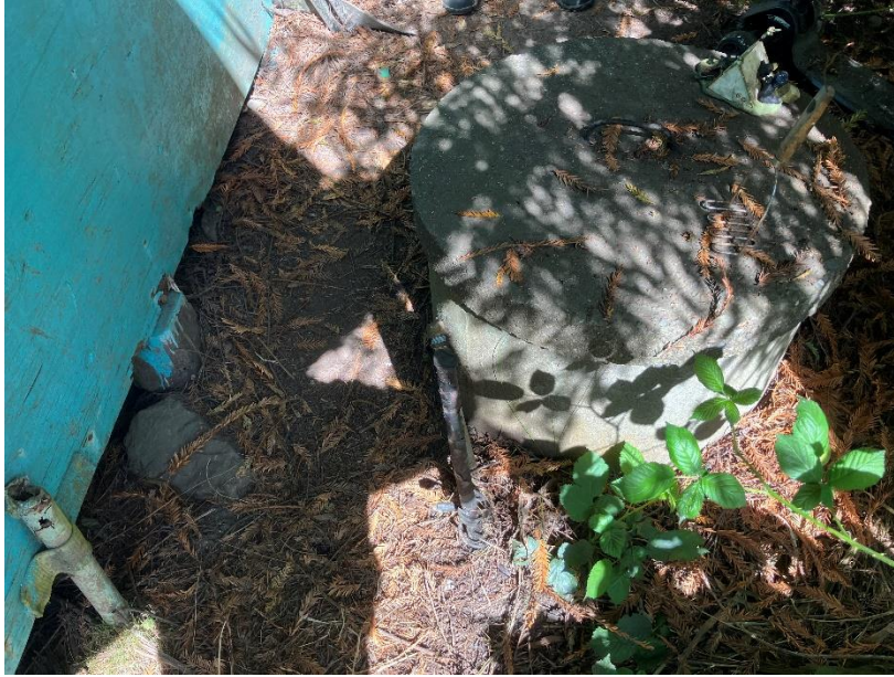
Dug well near structure #99
