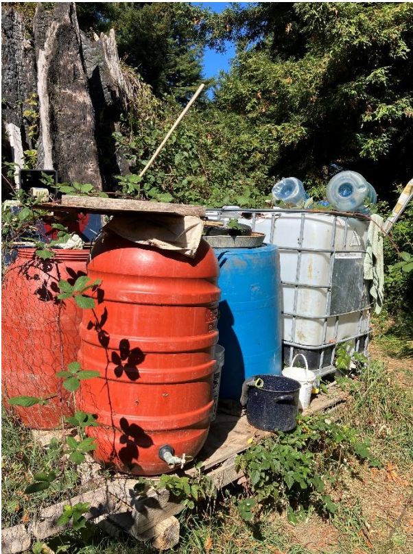
Miscellaneous water storage for irrigation or potable system
