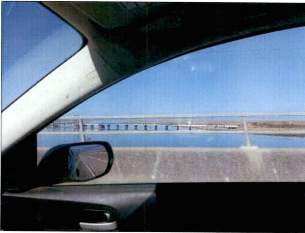
Image 2 (VAU 2, KOP 2). View of Eureka Slough NCRA railroad bridge from Highway 101 south. View looking north.
