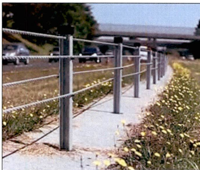
Typical cable barrier fencing (all project segments.)
